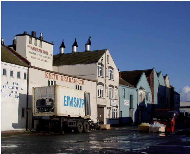
Figure 9.2 Fish processing buildings at Grimsby Fish Dock, including a smokehouse (© Colum Giles)
