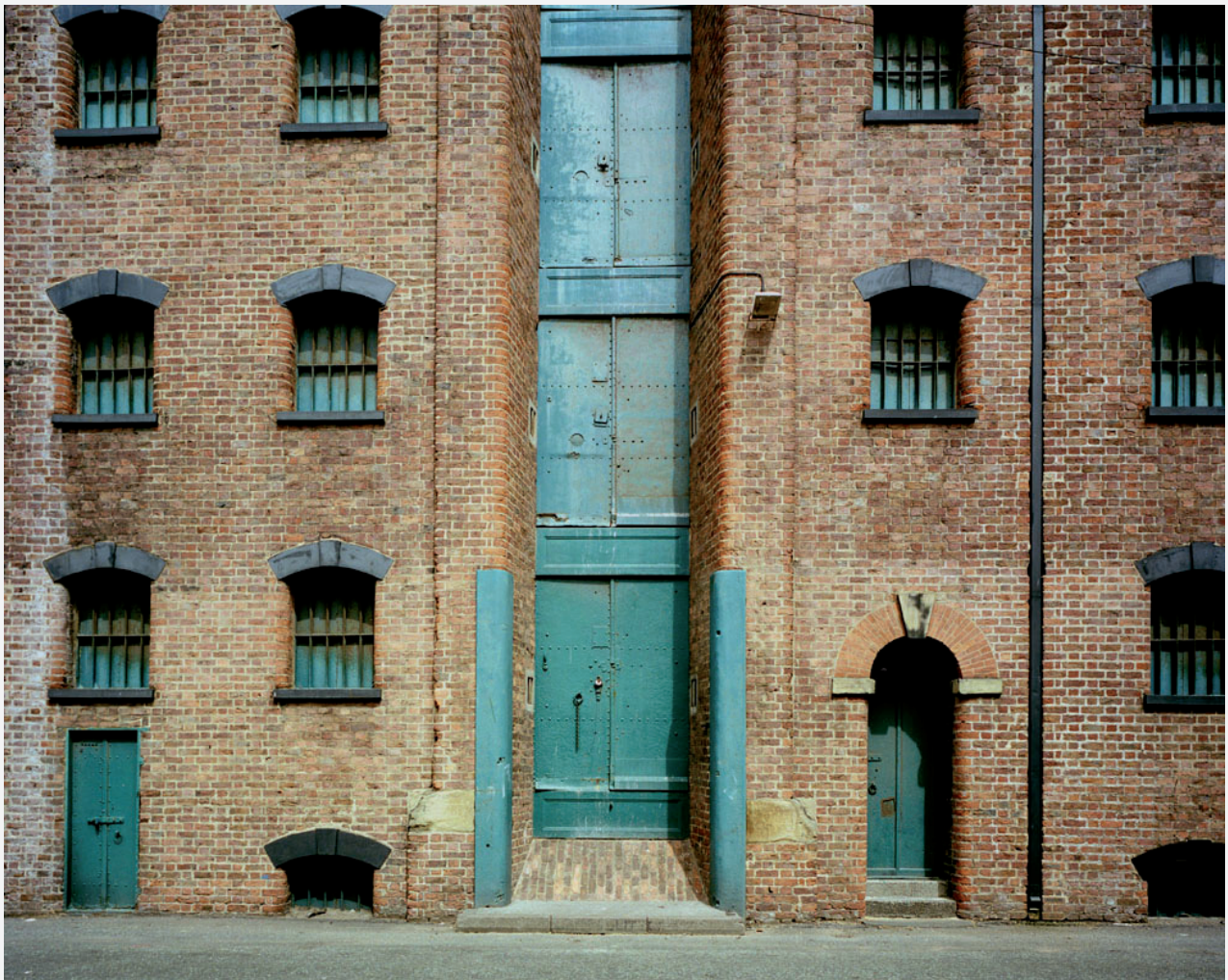
Figure 8.2 Fireproof warehouse, Liverpool, built in the 1840s (© English Heritage)
