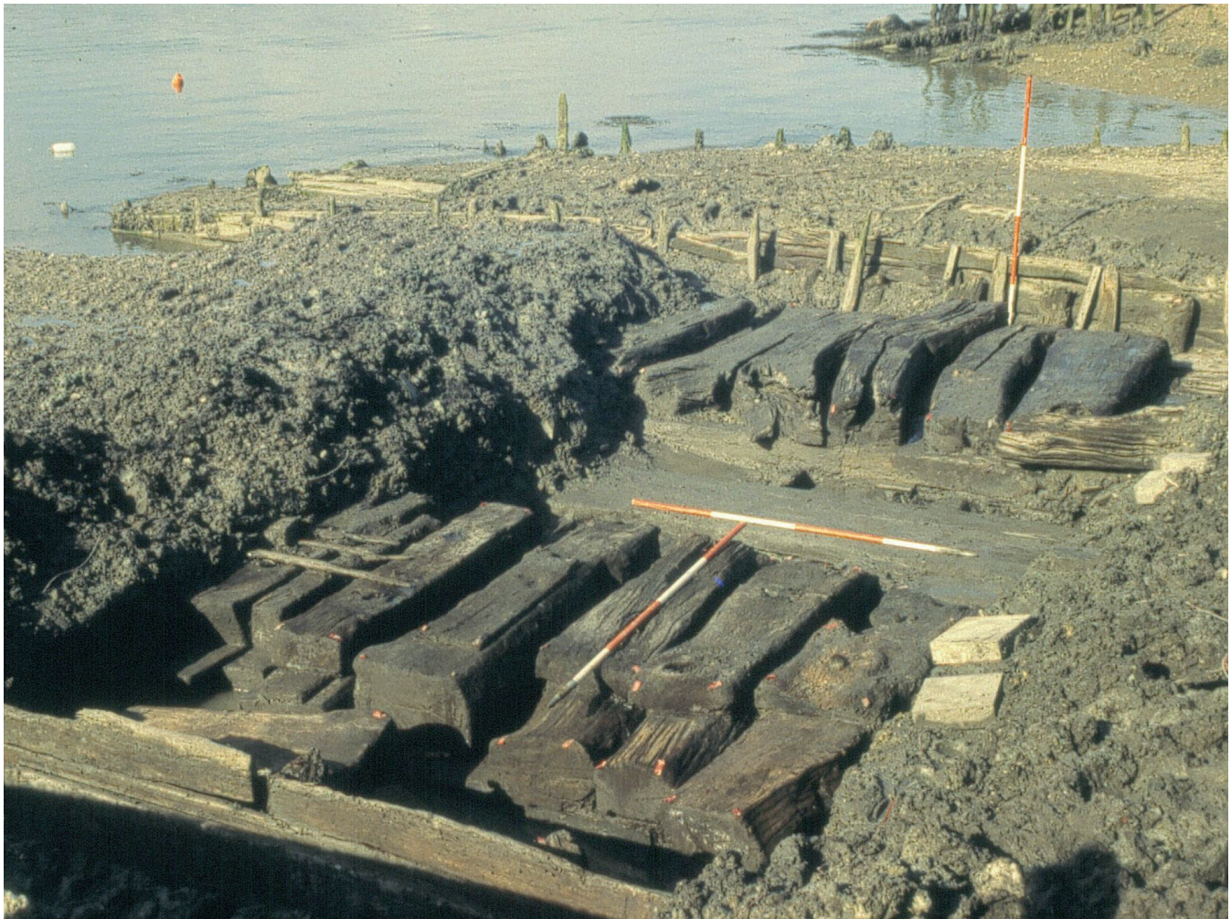
Figure 8.3 Excavations at Buckler's Hard in the mid-1990s reveal a wooden slipway (source: J Adams)
