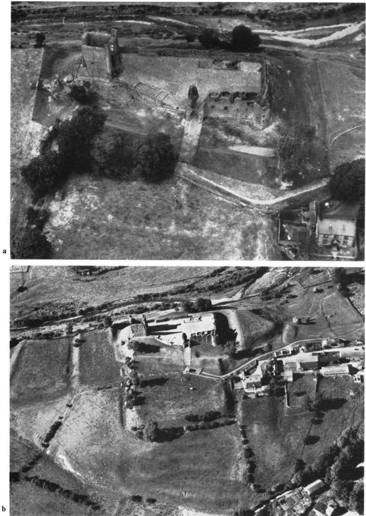
Fig. 3 Brough Castle (Cumbria) (NY 792141), looking north. a. In diffuse lighting, 9 July 1949: the absence of strong shadows permits nearly all the visible stonework to be studied in detail. Lines of parching in the grass (west of the house in the foreground) may be caused by the street system of the underlying Roman fort. b. In bright afternoon sunlight, 6 July 1971: oblique lighting picks out the earthworks of the Roman fort and medieval castle. Photos: (a) Crown Copyright reserved, (b) University of Cambridge; copyright reserved
