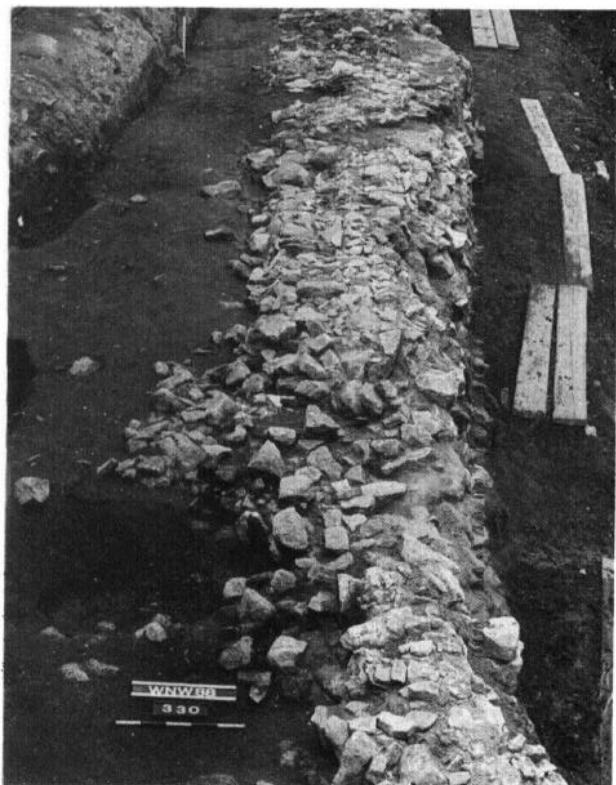
Fig 21.4 Lincoln: Waterside North excavation, possible stone pier or slipway foundation
