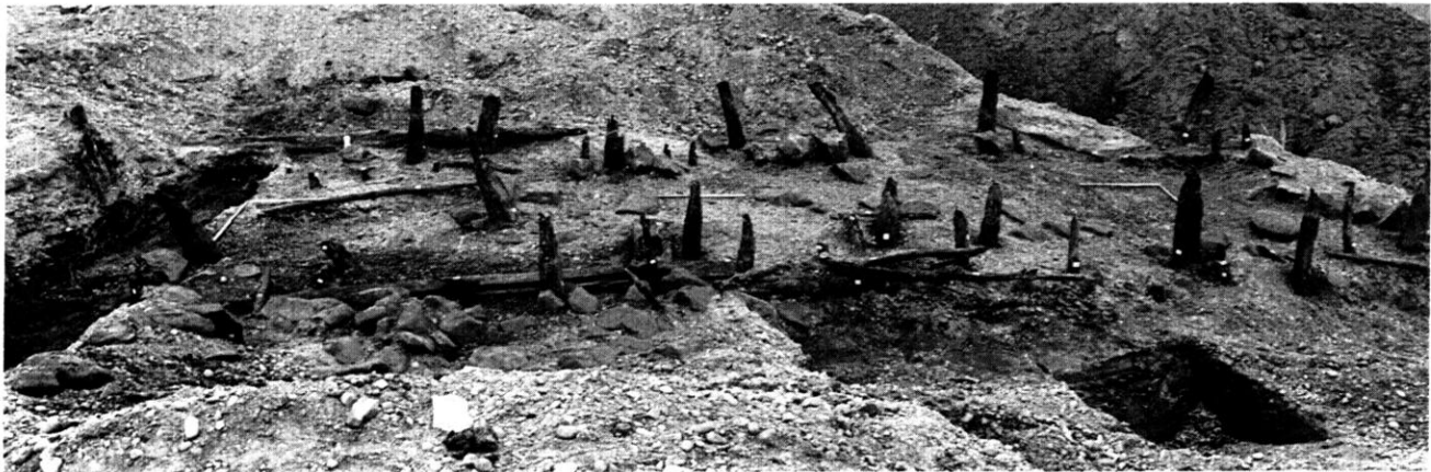
Fig 11.13 A Norman mill-dam at Hemington, Leicestershire. The double row of watted posts holds a core of quarry rubble and millstone fragments. An earlier fishweir shows on the left as wattle and a line of small posts
