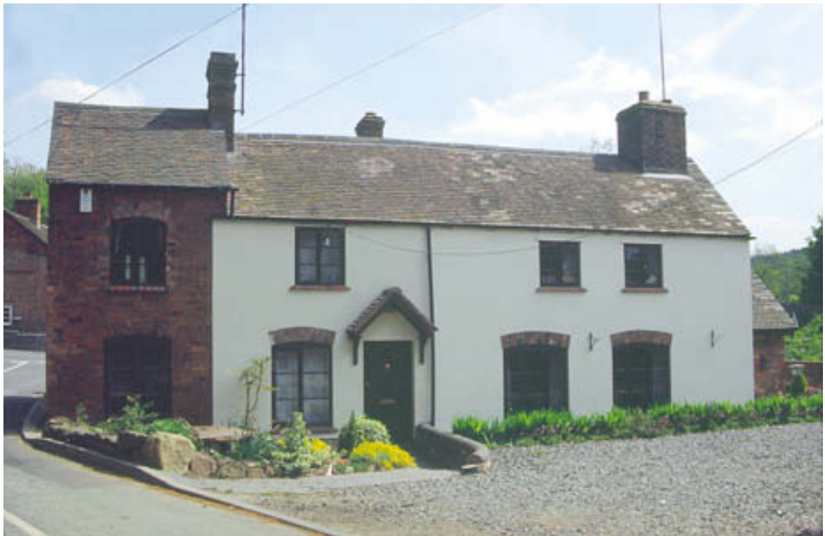
Figure 4.5 Cottages at Coalport after conservation. Windows and doors have been replaced and considerable renewal has taken place.
