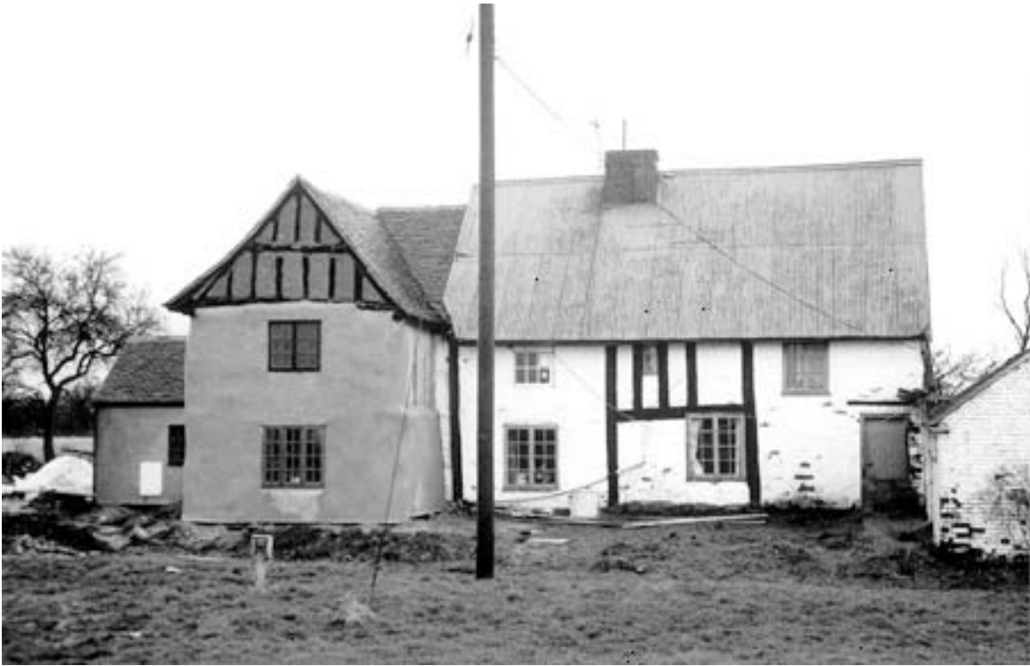
Figure 10.3 Hall House, Sawbridge, Warwickshire, view from east
