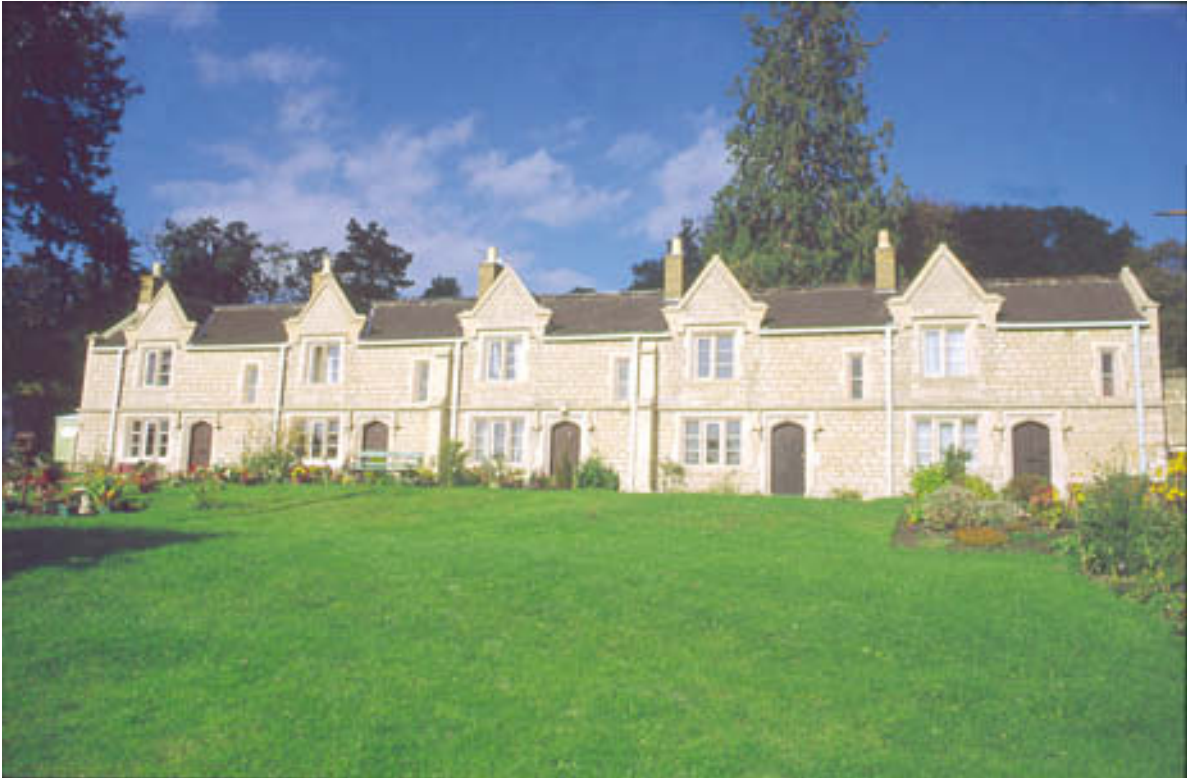
Figure 4.7 Miss Ann Bearpacker Almshouses, Wotton under Edge, Gloucestershire, 1837. The exterior of the building has been carefully conserved. In comparison, see Fig 4.8, which shows that relatively little historic fabric survives in the interior.
