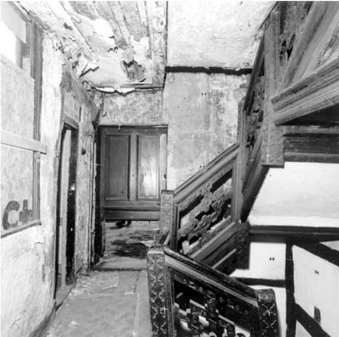
Figure 7.10 Staircase House, Stockport. 17th- century cage- newel staircase. Note the targets for rectified photography in the background. (Dennis Thompson)
