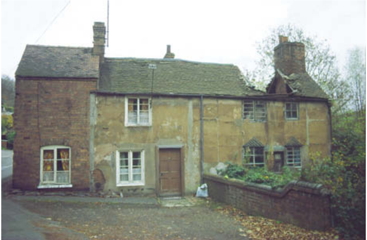
Figure 4.4 Cottages at Coalport, Shropshire, prior to conservation
