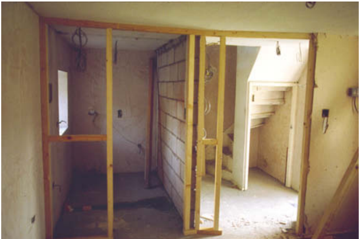
Figure 4.8 Interior of almshouses, Wotton under Edge, Gloucestershire. The surviving staircase was about to be removed at the time this picture was taken.
