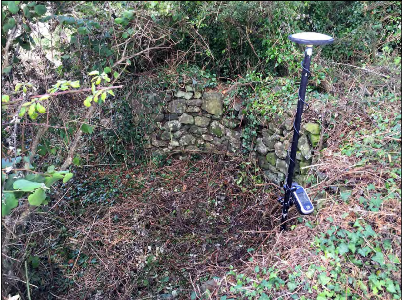
Plate 1: Location A, (Figures 2 and 3), a stone revetted likely mine shaft (scale: 2m GPS pole)
