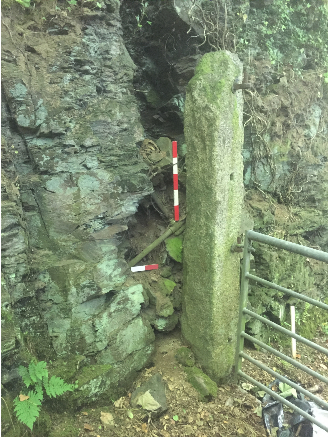
Plate 1: water pipes at the southern entrance to Plot 3, looking east-south-east (0.5m and 0.2cm scales)
