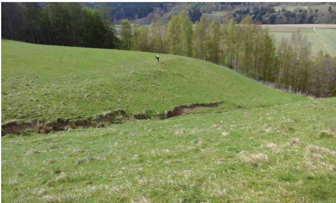
Photo A2 – Parcel 1 before survey, looking to the south-west, showing the ravine
