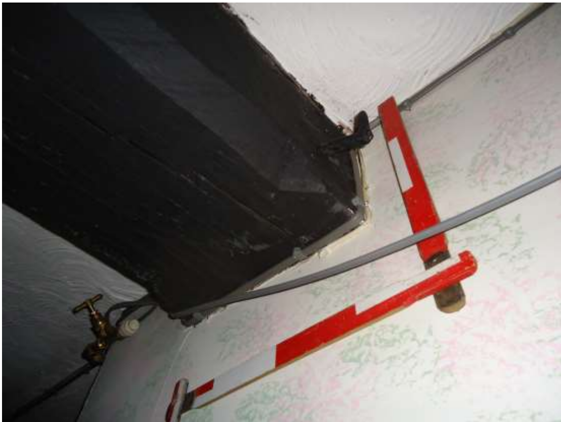
Plate 10; view of stopped-chamfer on beam over principal floor.
