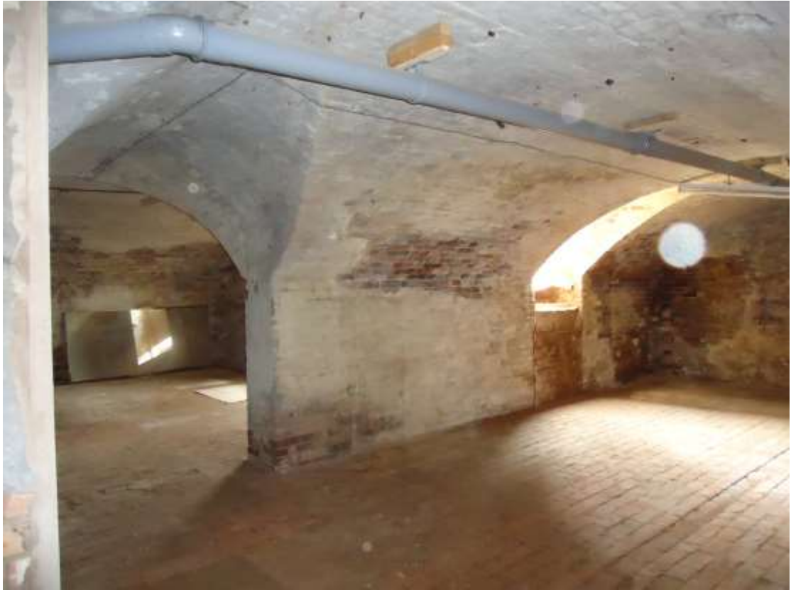
Plate 29; view to the west showing the front and rear basements.
