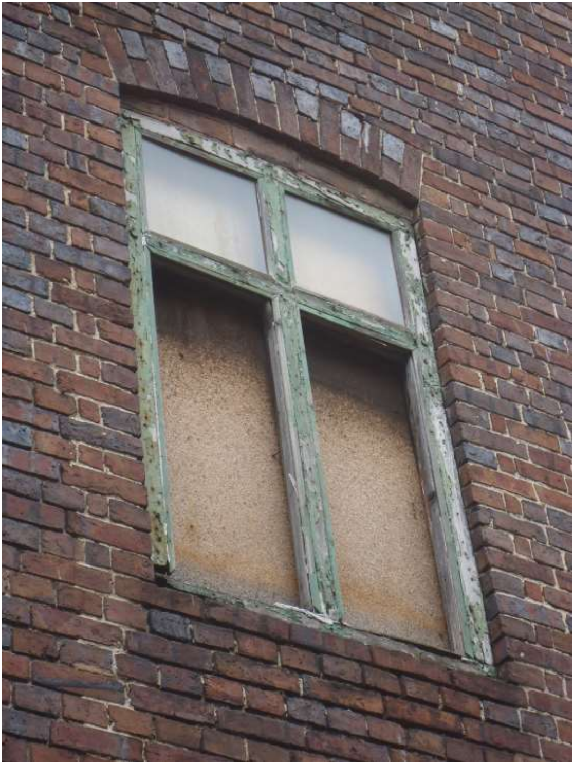
Plate 6; first floor window on front elevation.
