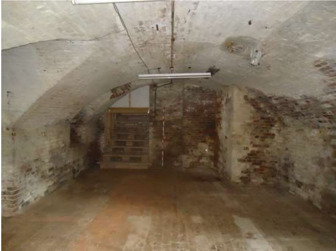
Plate 31; view within the rear basement to the south-east.
