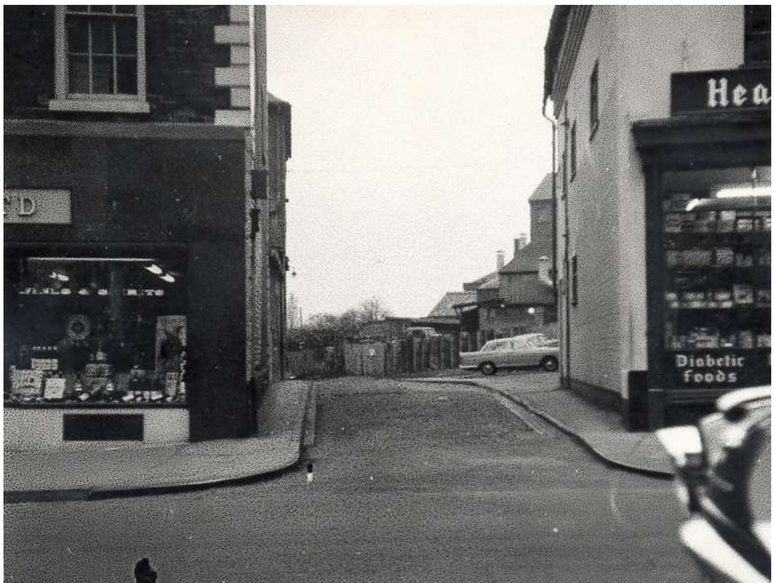
Plate 36; the junction of Dolday and Broad Street in the 1960s, view from the south-east.
