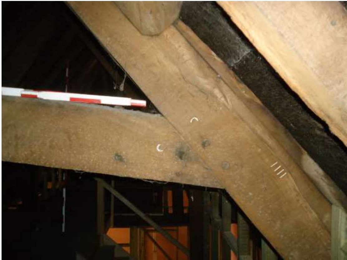
Plate 25; and another detail of carpenter's numbers within the rear roof.
