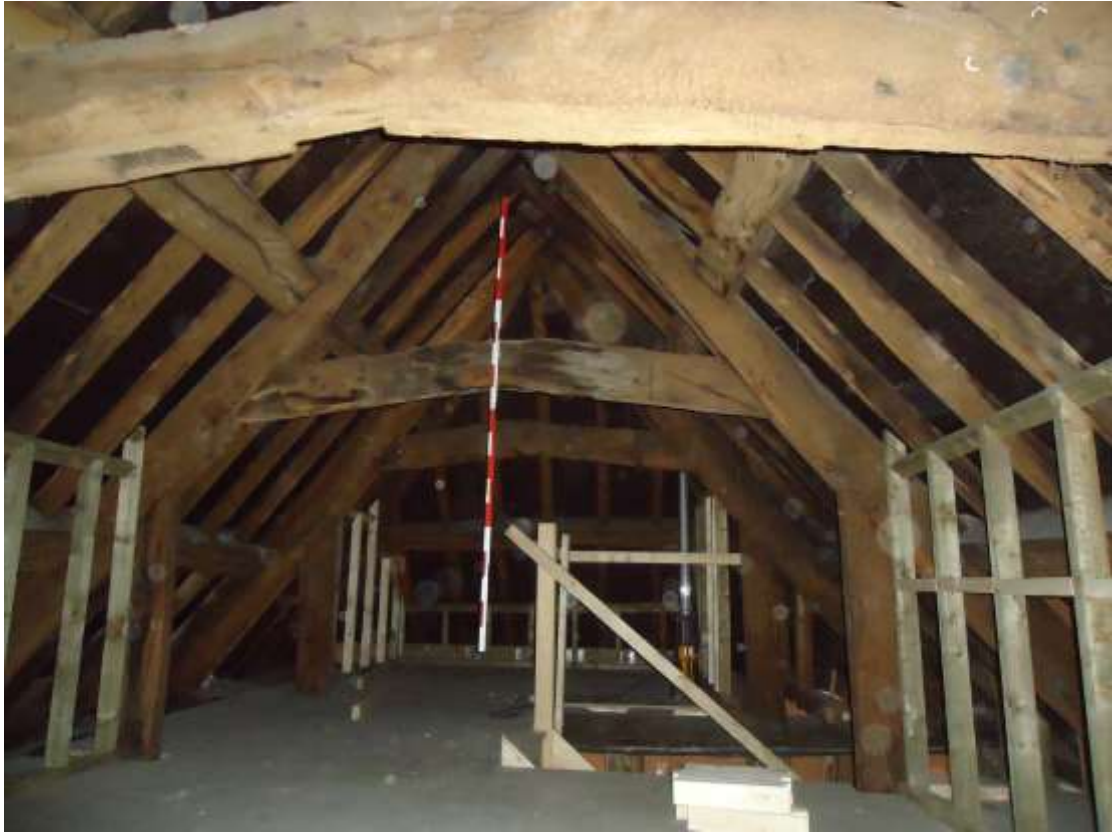
Plate 19; view within the rear roof to the south-east during construction.
