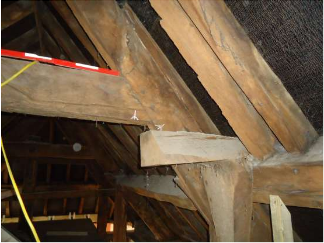
Plate 21; remains of hoist structure within the front roof.
