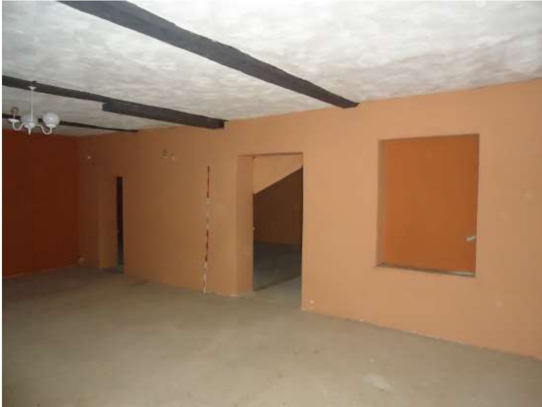
Plate 13; view to the north at second floor within the rear range.
