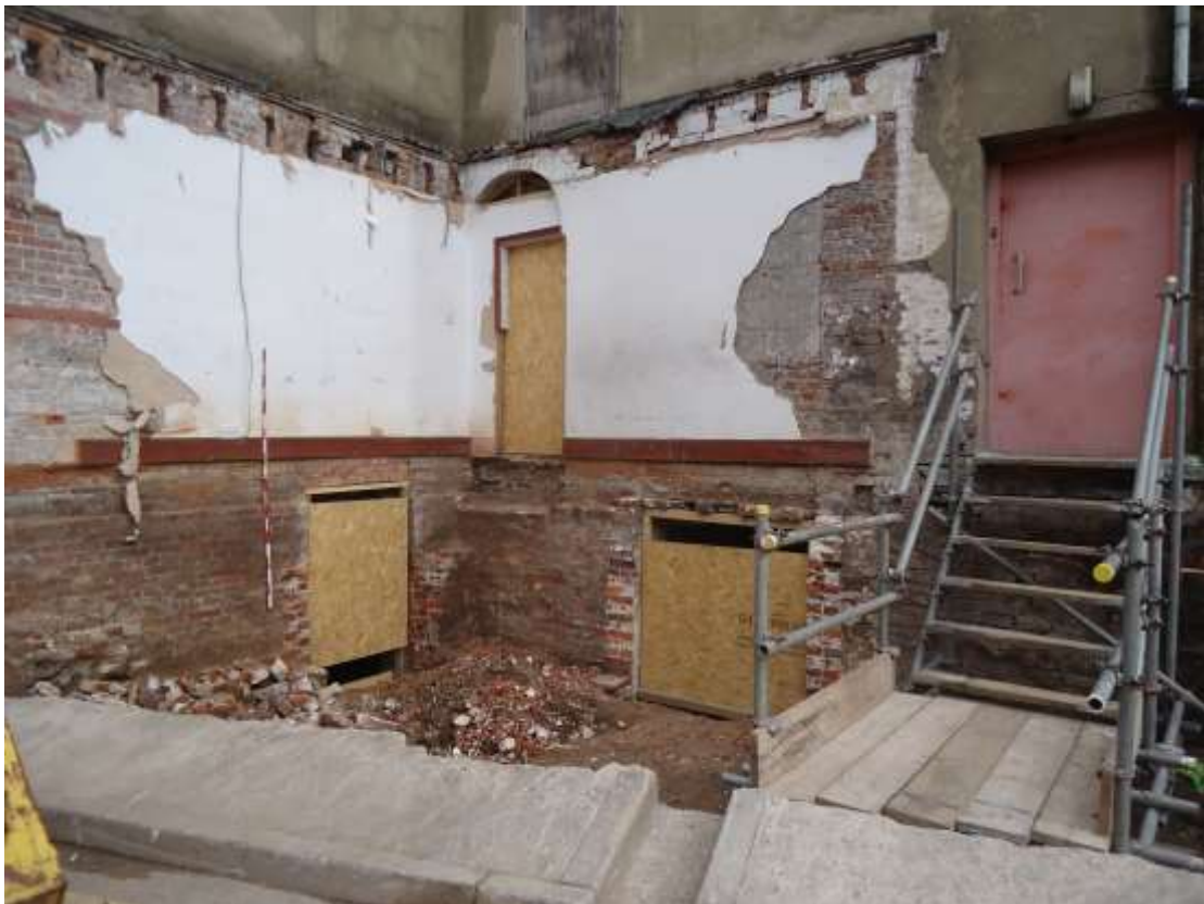
Plate 8; view of warehouse from the west during 2013 works.
