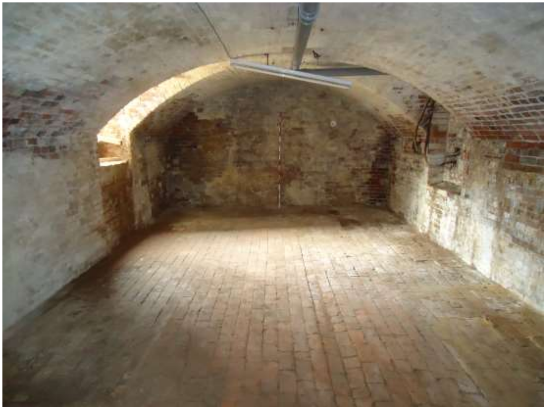
Plate 26; view of the front basement to the north-west.
