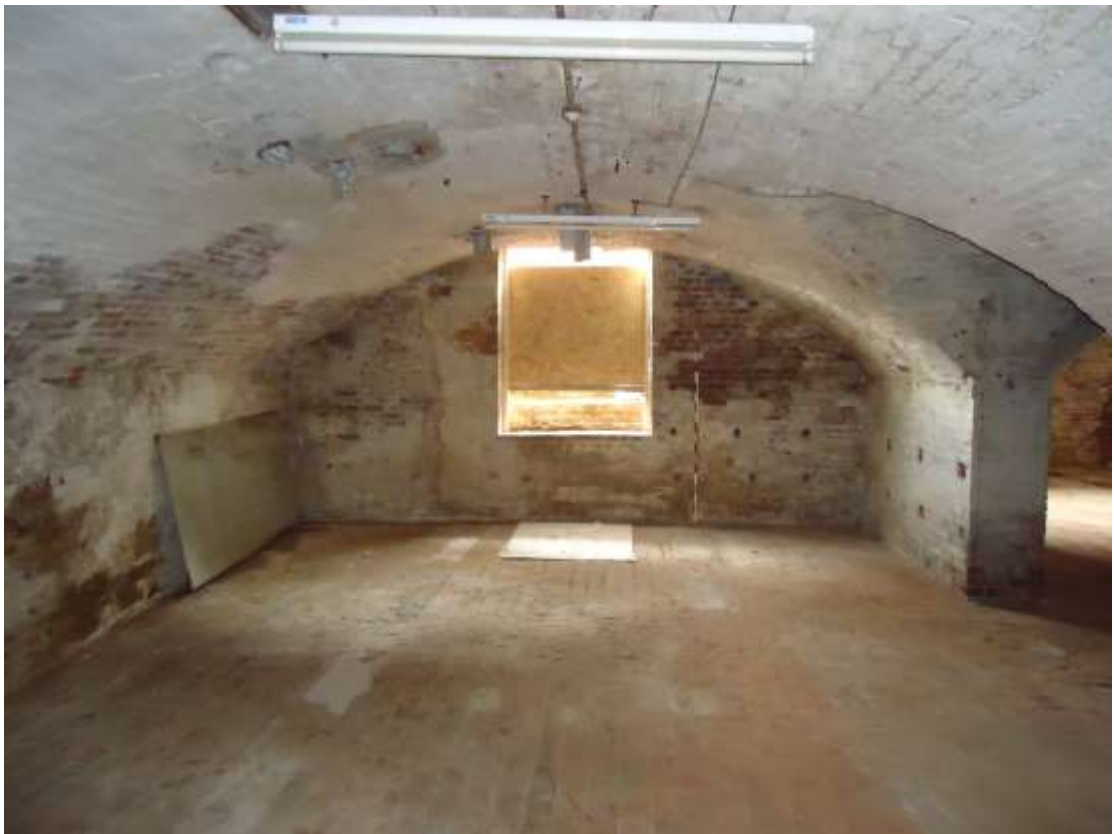
Plate 30; view of the rear basement to the north-west.
