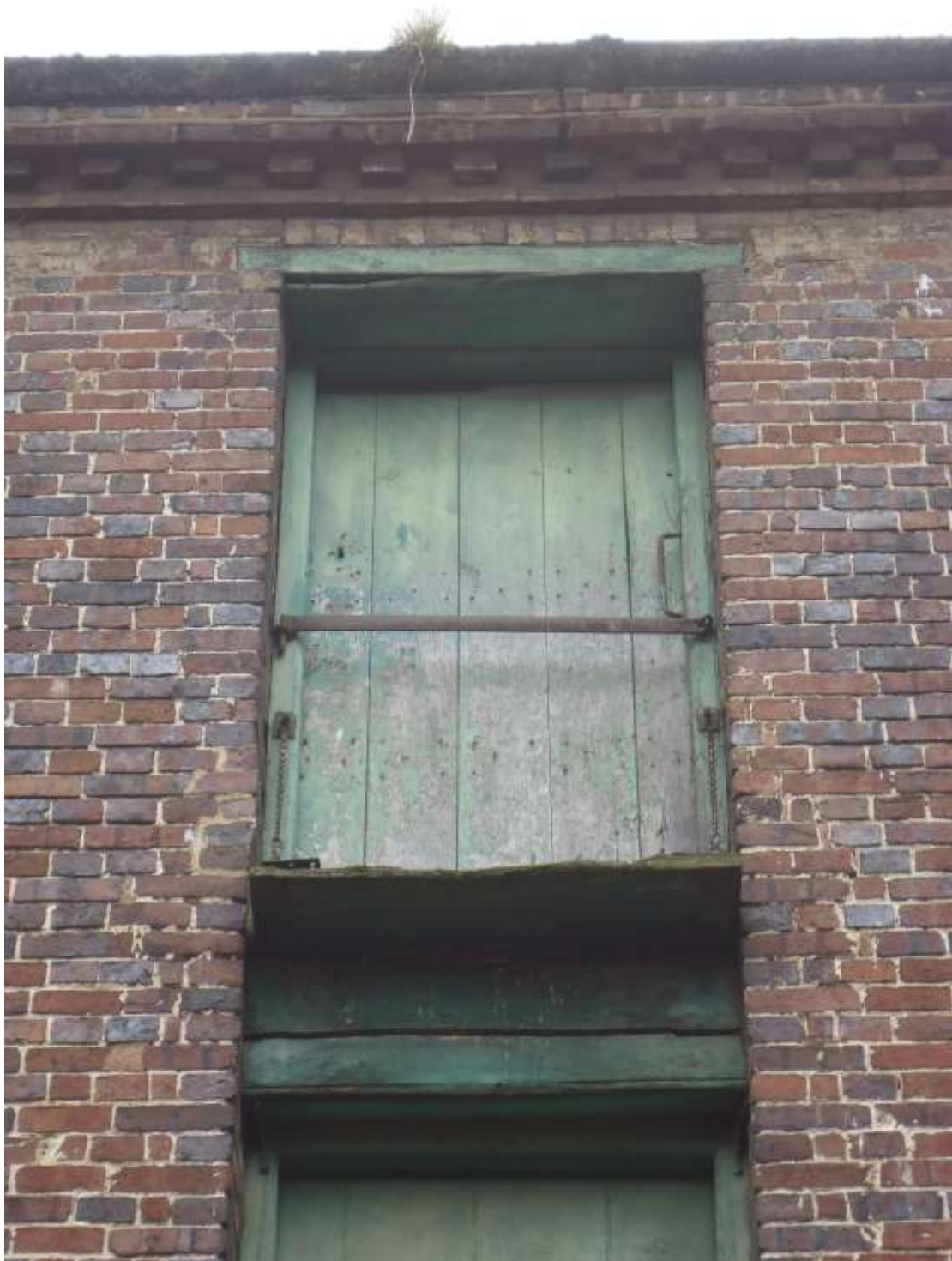
Plate 5; central goods door on the second floor.
