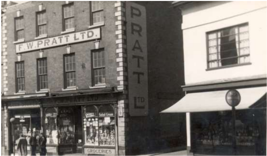
Plate 35; Pratt grocers shop front on Broad Street, view from the east
