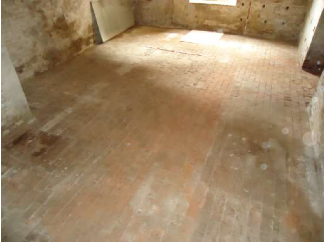
Plate 33; view of the rear basement floor to the west.
