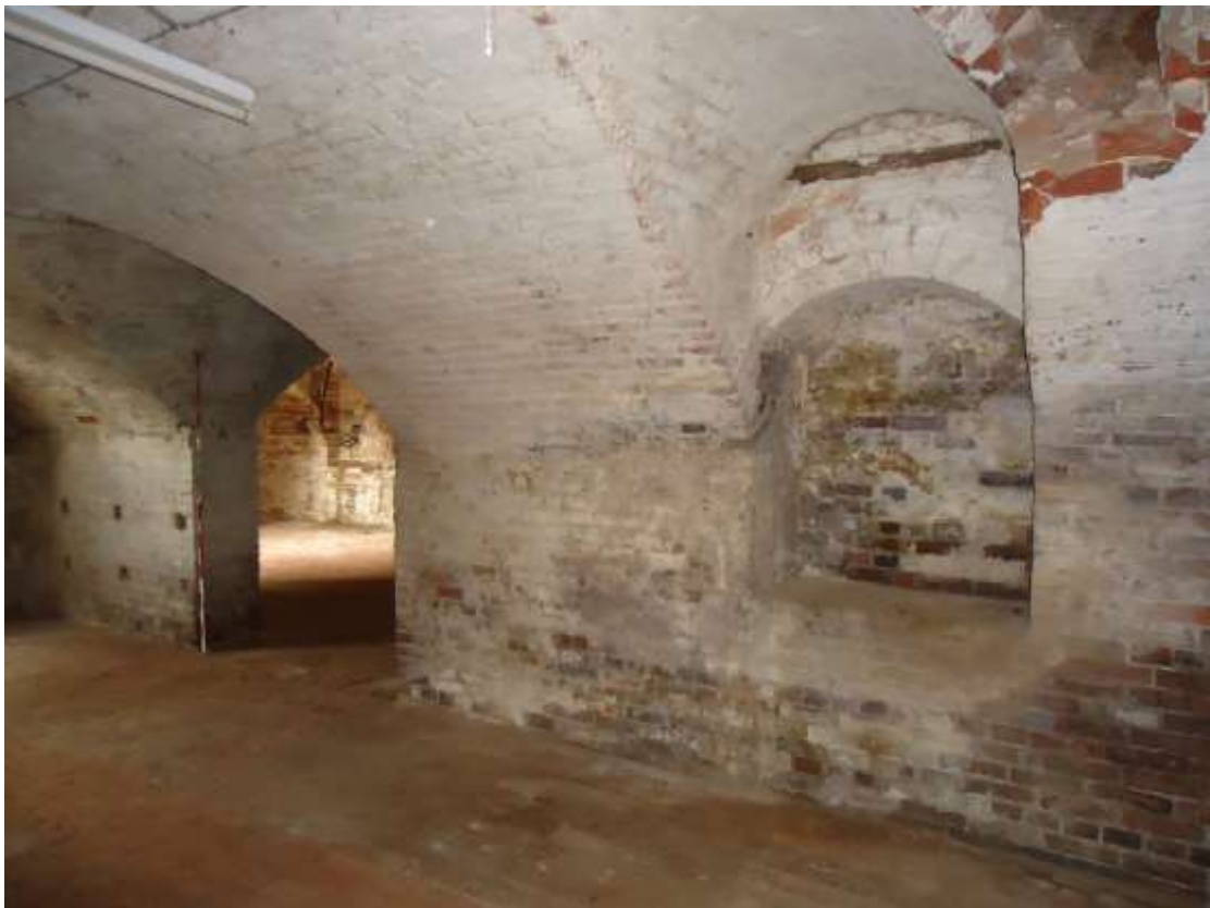
Plate 32; view within the rear basement to the north.
