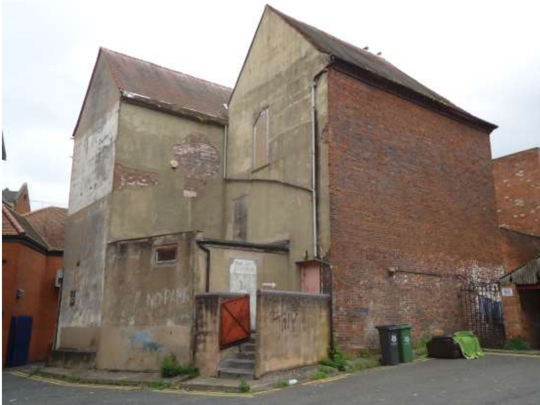
Plate 7; view of the warehouse from the west prior to 2013 works.
