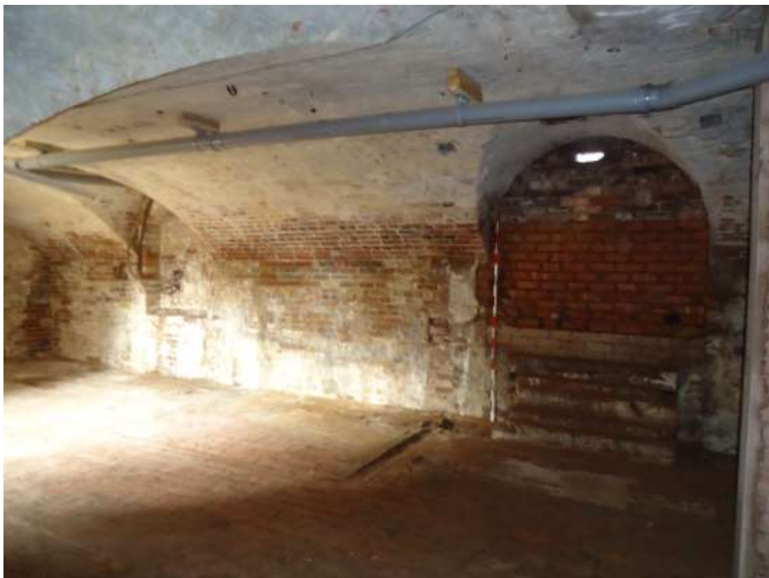
Plate 28; view of the front basement to the north.
