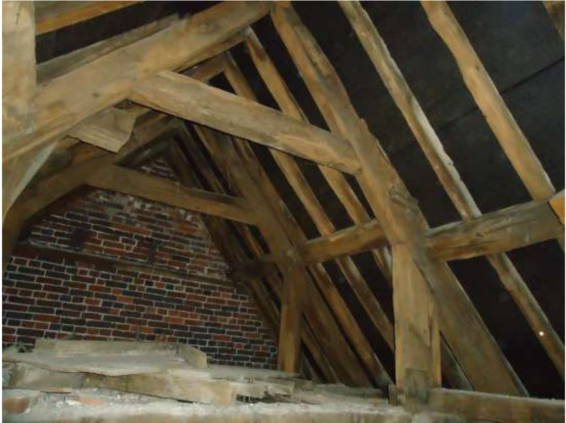
Plate 17; view within the front roof to the north.
