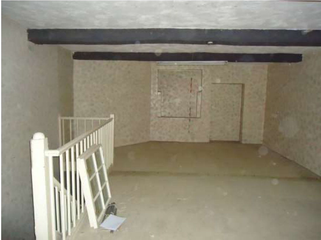
Plate 11; view to the north-west at first floor level within the rear-range.
