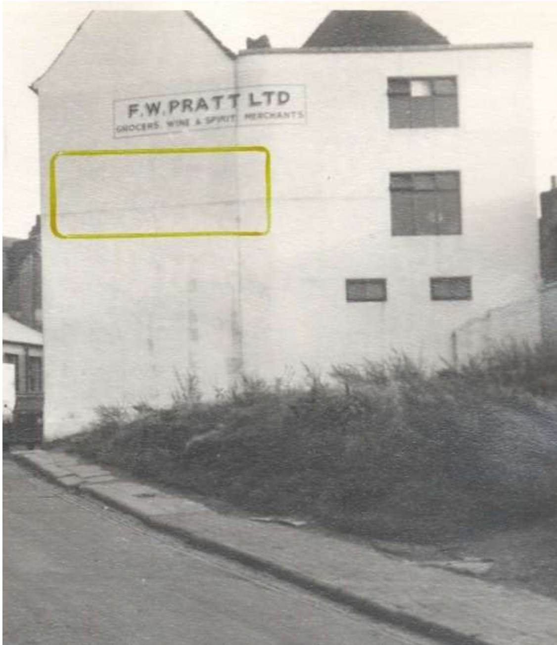
Plate 37; north-west elevation in the 1950s, the sign F.W Pratt Ltd in the picture is now gone, the paintwork having weathered away to reveal an earlier sign the lettering of which is consistent with that on the front and shown in plate 34. The lowest floor of the three-storey flat roofed infill of the west angle, probably built following the demolition of adjacent properties in the 1930s. survived until the present study.
