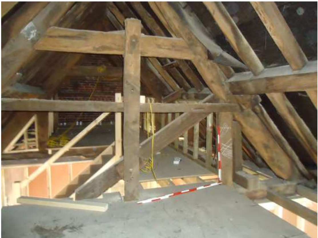
Plate 18; view within the front roof to the north during construction.
