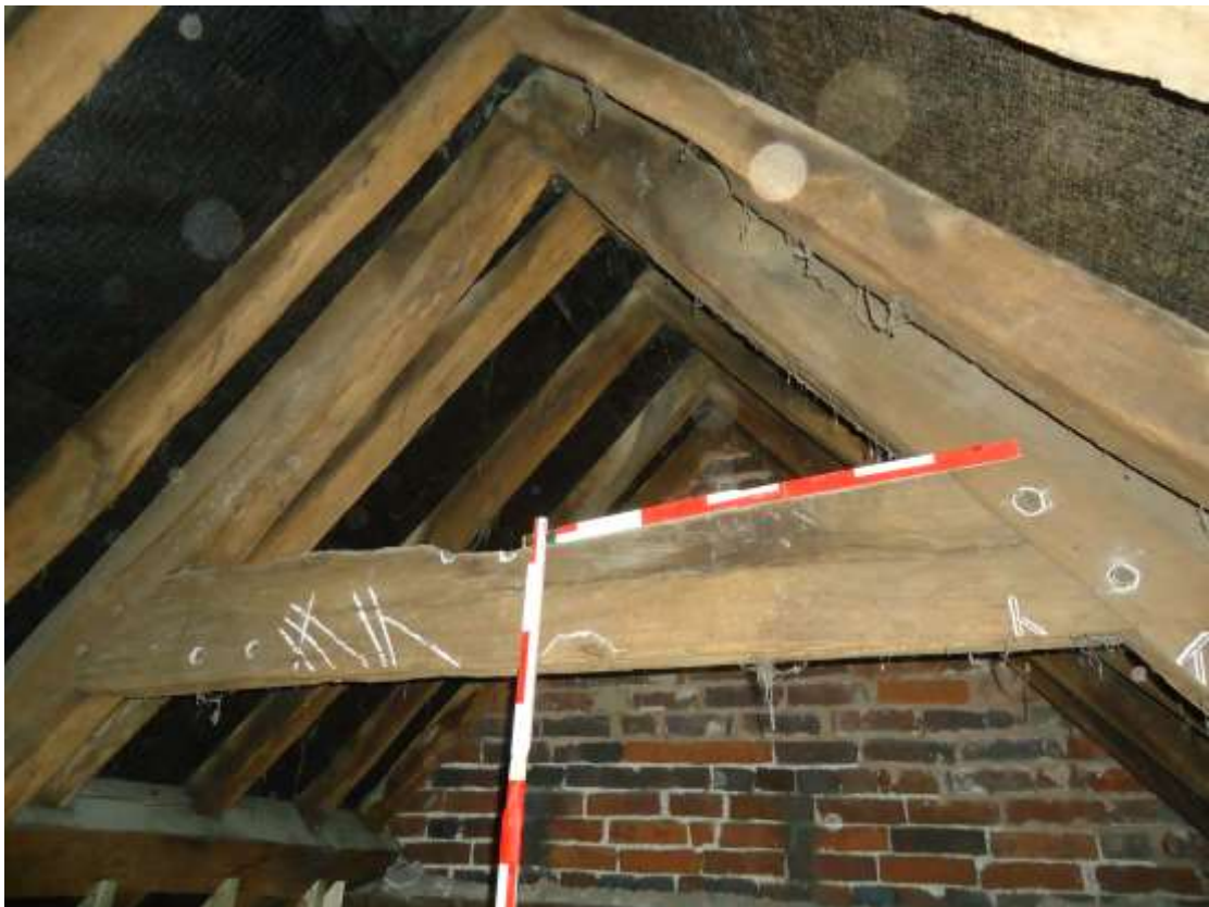
Plate 20; roof detail at north-west end of front roof.
