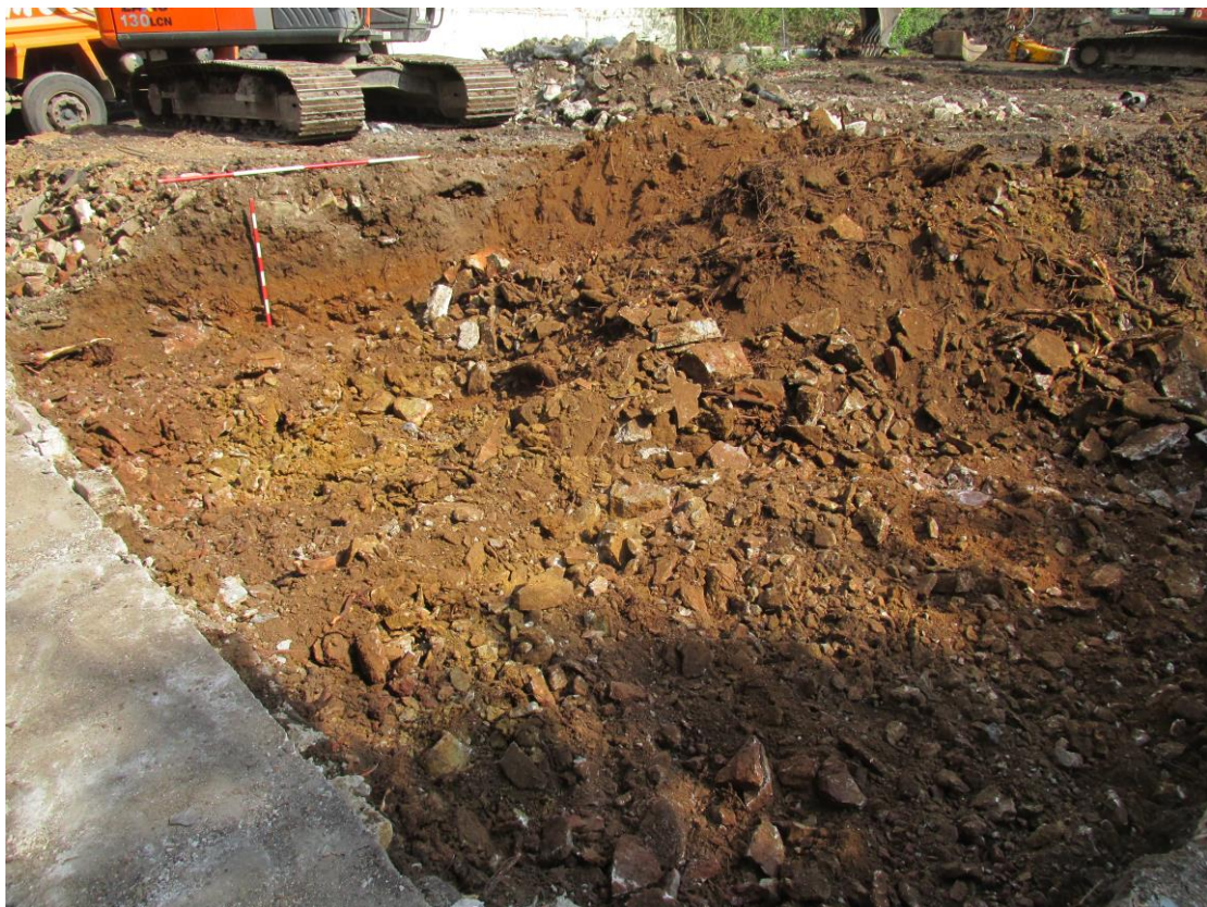
Plate 26; section g, overall view
