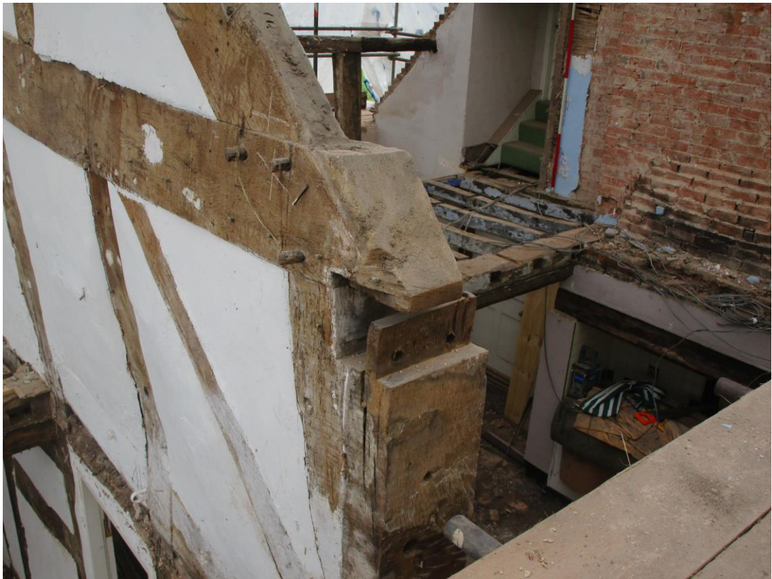
Plate 23; eastern tie-beam assembly from south-east.
