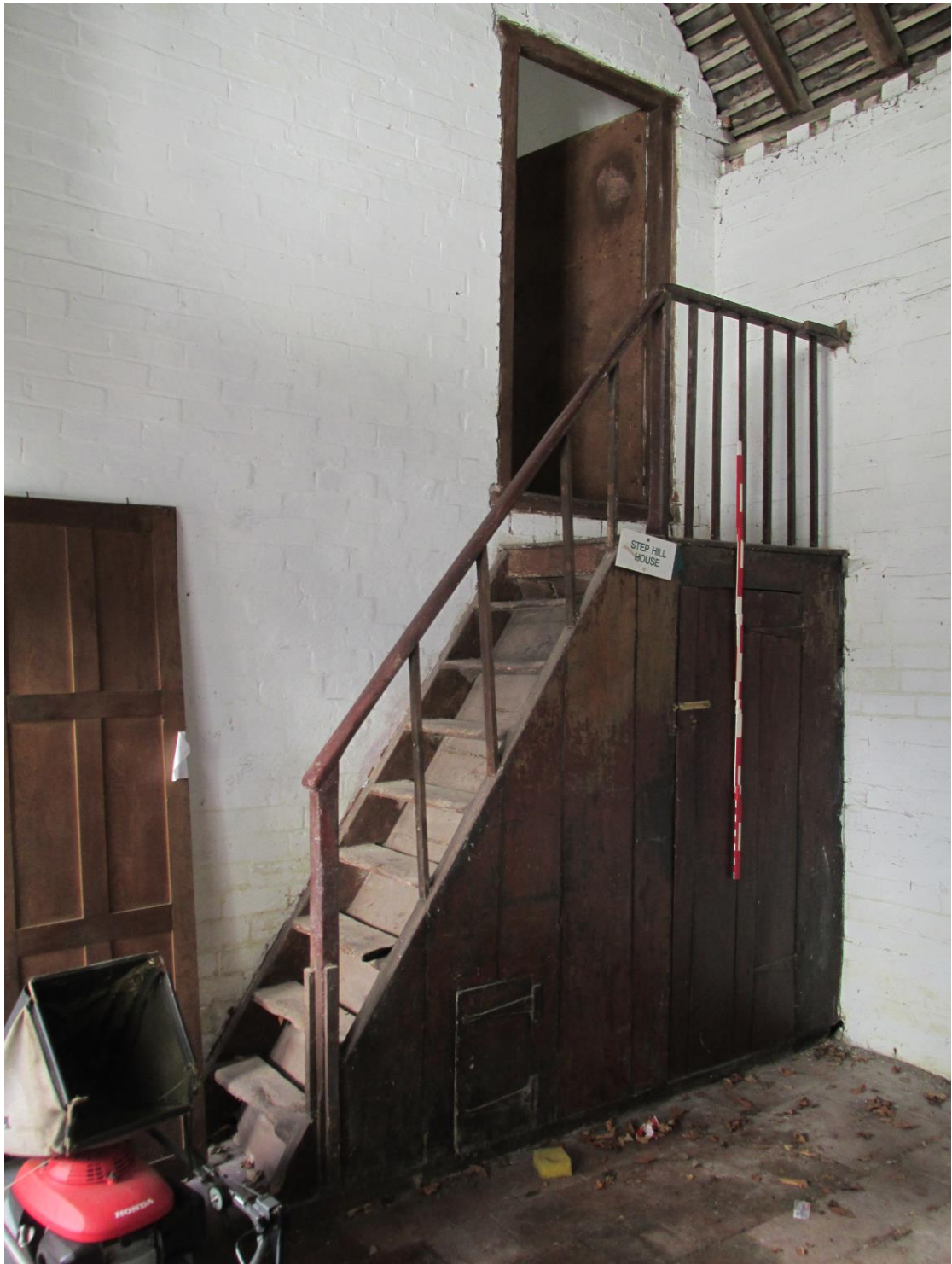
Plate 14; out-house stair to north-east.
