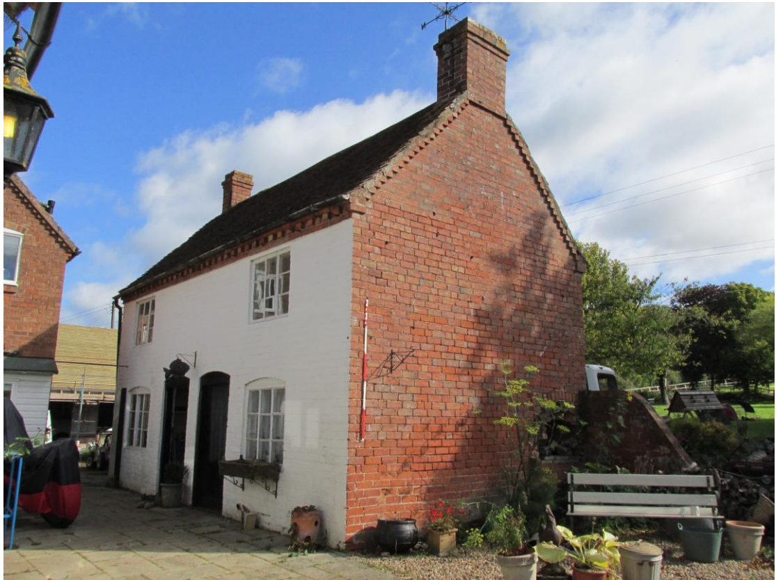
Plate 3; out-house from south-west.
