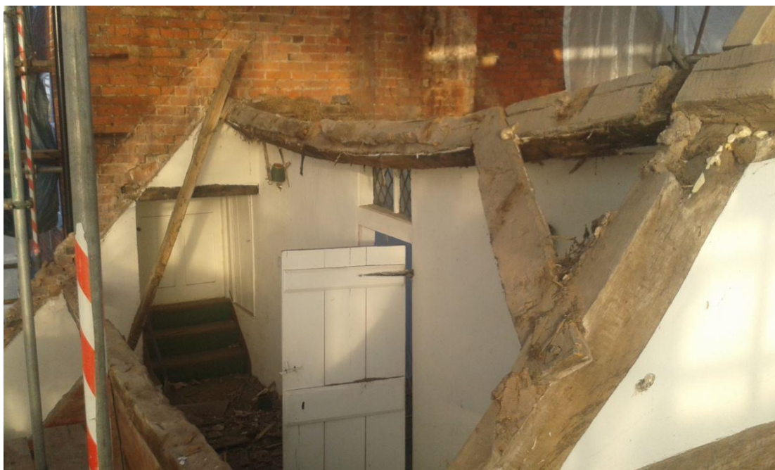
Plate 30; north-bay west-purlin; re-used principal-joist (see Pl. 28).
