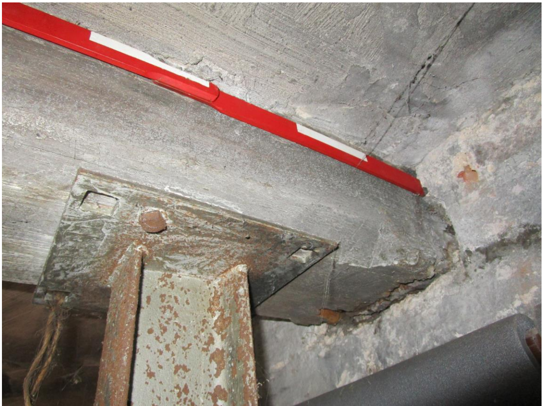
Plate 7; chamfers and stops in cellar
