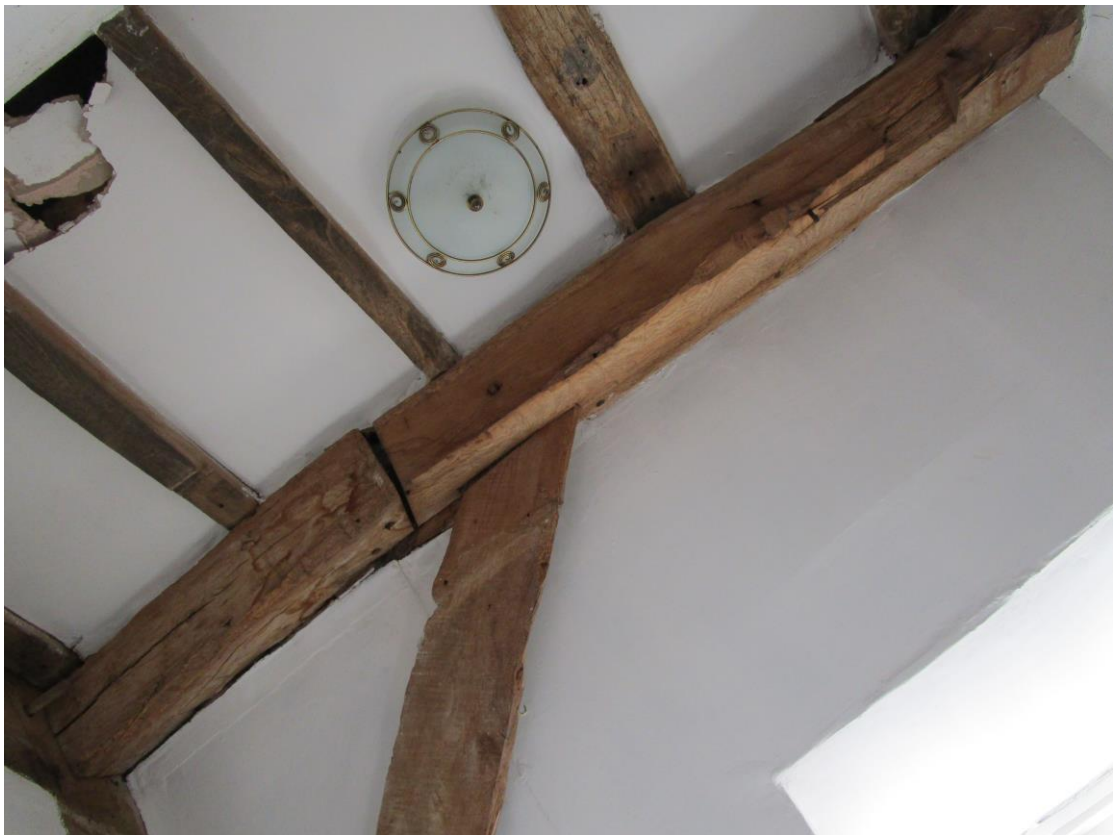
Plate 28; south-bay east-purlin, scarp and wind-brace.
