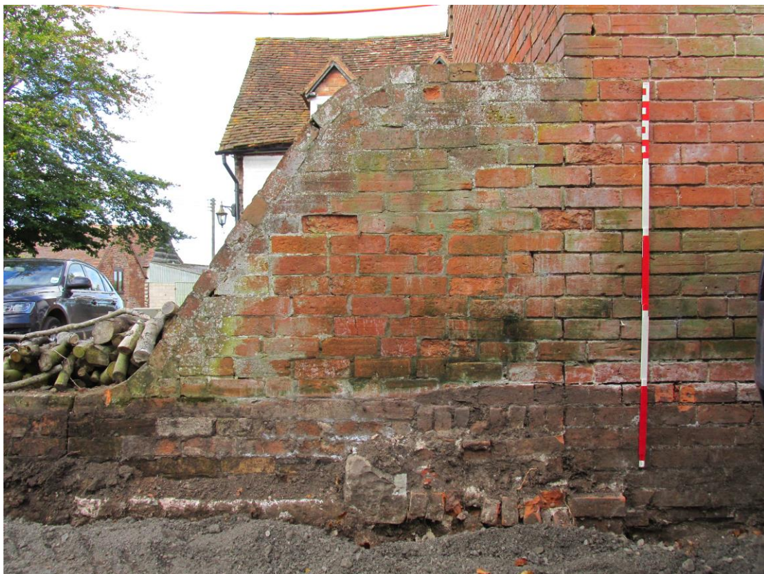
Plate 10; blocked opening below oven from east.
