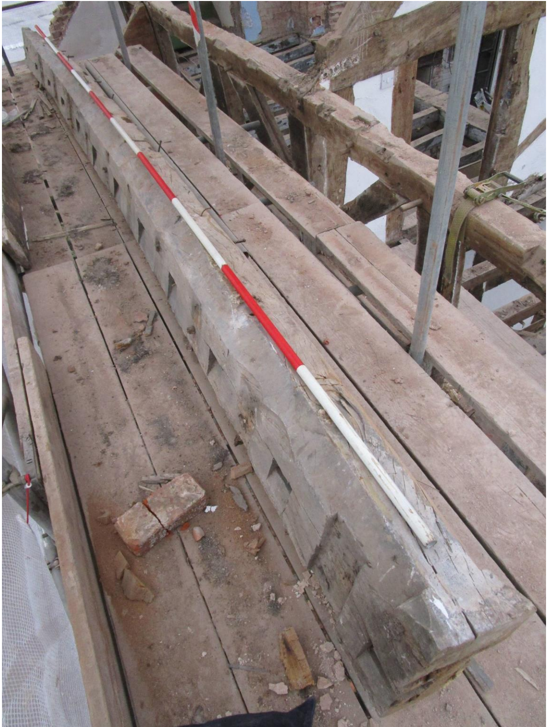
Plate 29; north-bay west-purlin; a re-used principal-joist (see Pl.29).
