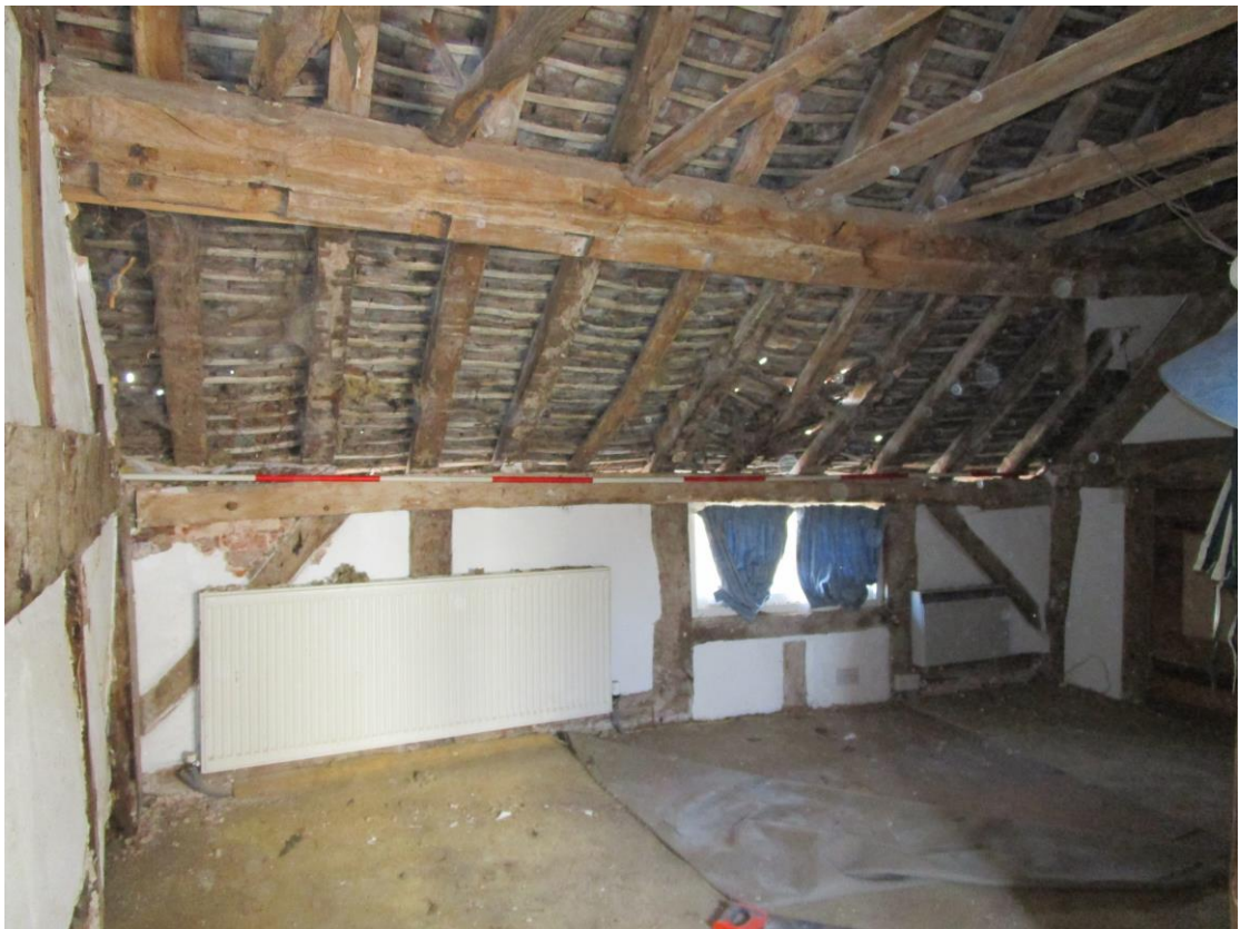
Plate 19; south-wing interior to west.
