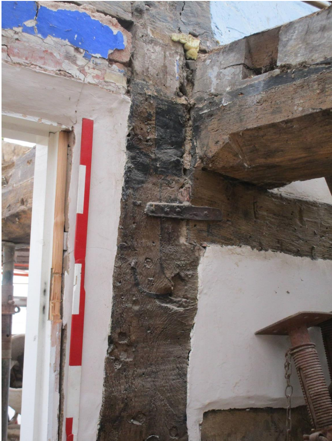
Plate 25; detail of middle frame and principal from north.
