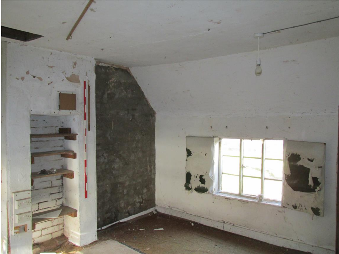
Plate 11; out-house upper room to north-east.
