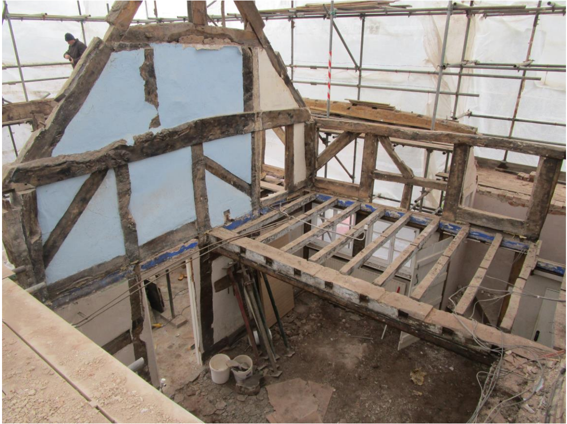
Plate 18; south-wing interior to south-west.
