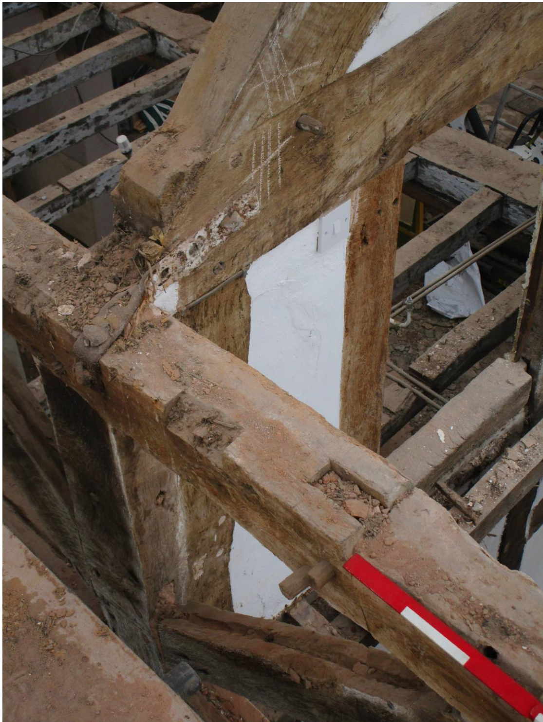
Plate 21; western tie-beam assembly from south-west (see Pl. 21)
