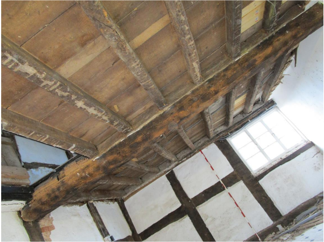
Plate 27; south-bay showing upper-floor construction to west.
