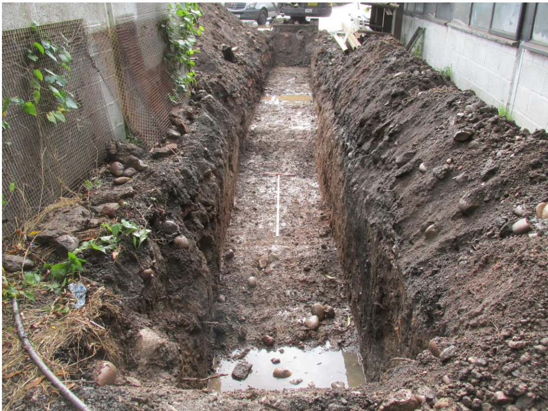
Plate 2; view of excavated trench, from the north-east
