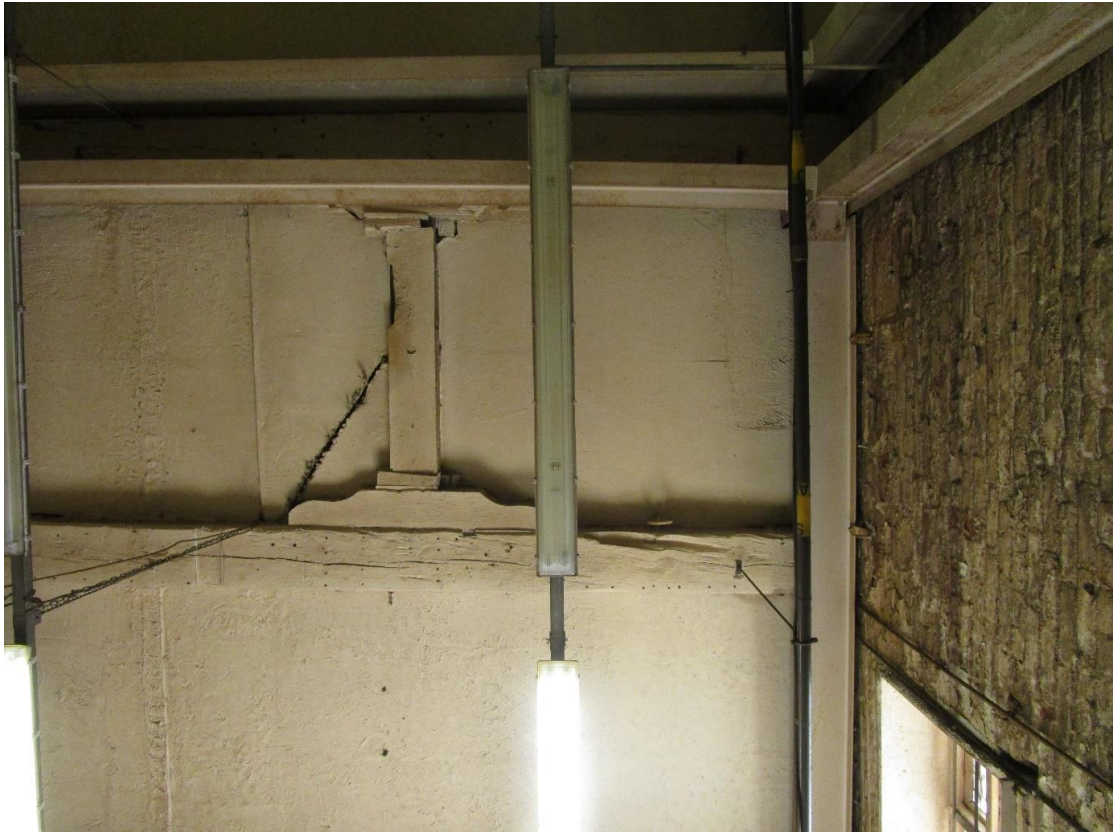
Plate 12; Timber feature in upper floor
