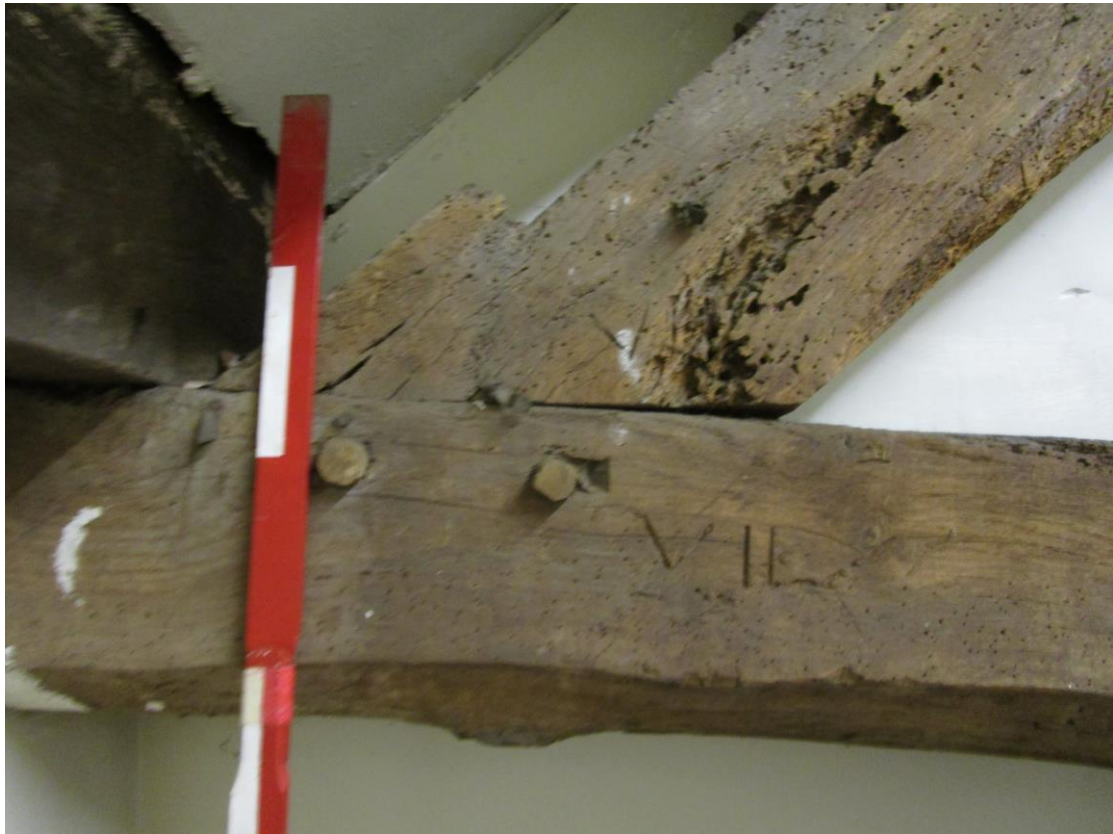
Plate 13; Carpenters' numbers on roof truss B, for location see Fig 5
