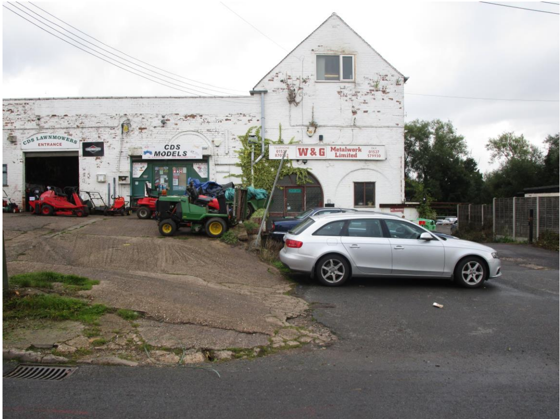
Plate 6; End of mill and existing road frontage
