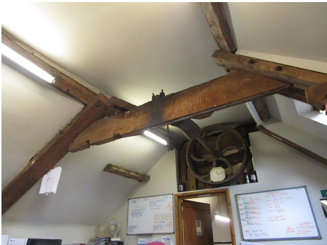
Plate 14; Remains of hoist in central part of mill
