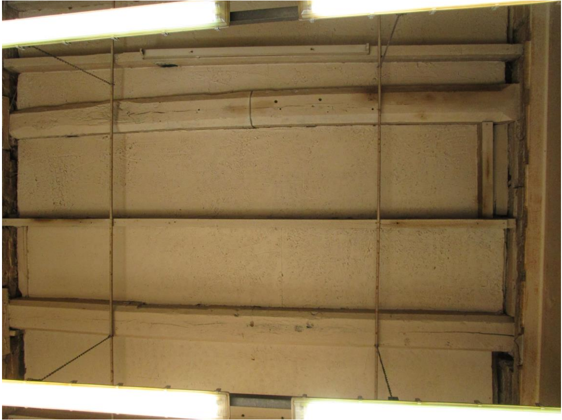
Plate 11; Chamfered beams in eastern part of mill
