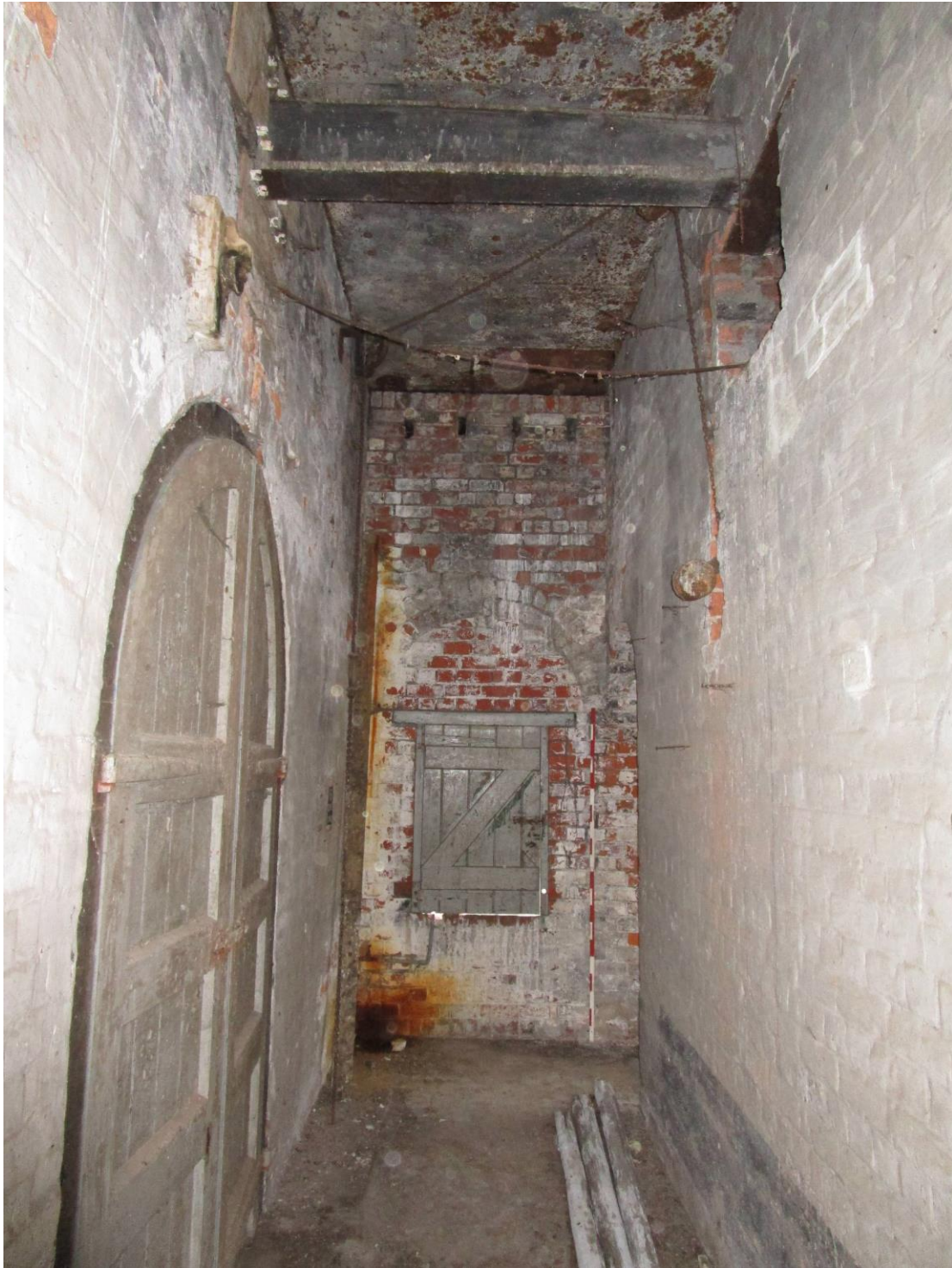
Plate 16; Stair-tower; fourth storey interior from north
