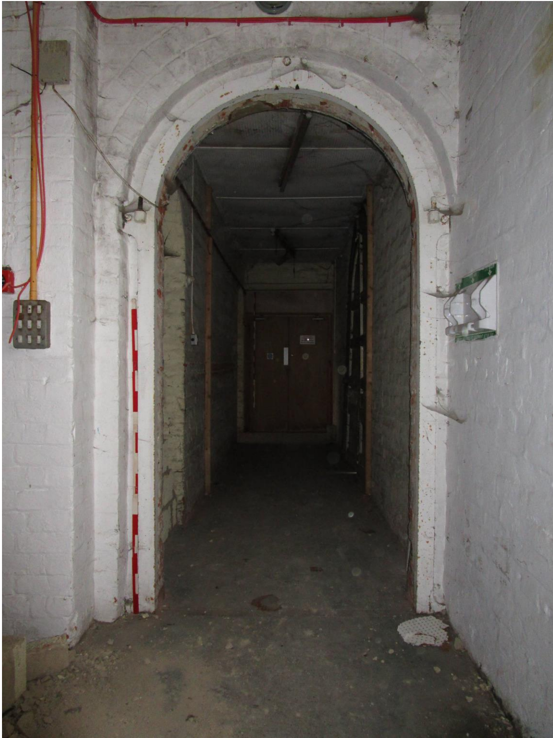
Plate 19; Stair-tower 1 st floor passage from south showing original building 3 iron door-frame
