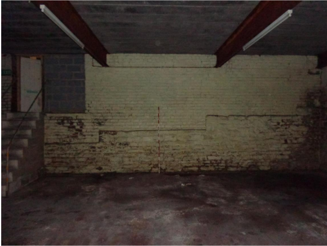
Plate 40; Building 9 interior east end of north wall
