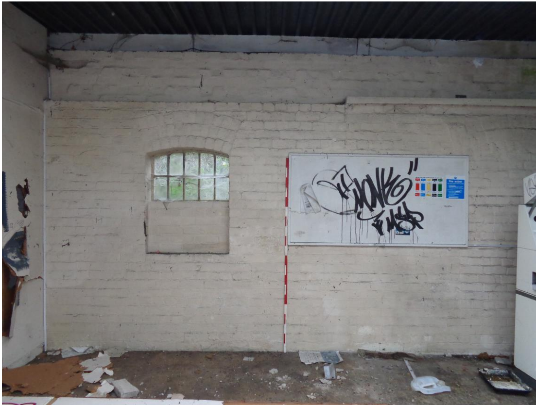
Plate 42; Building 9 interior north wall detail
