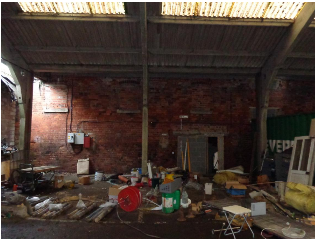
Plate 43; Building 9 from north showing blocked 1 st floor windows
