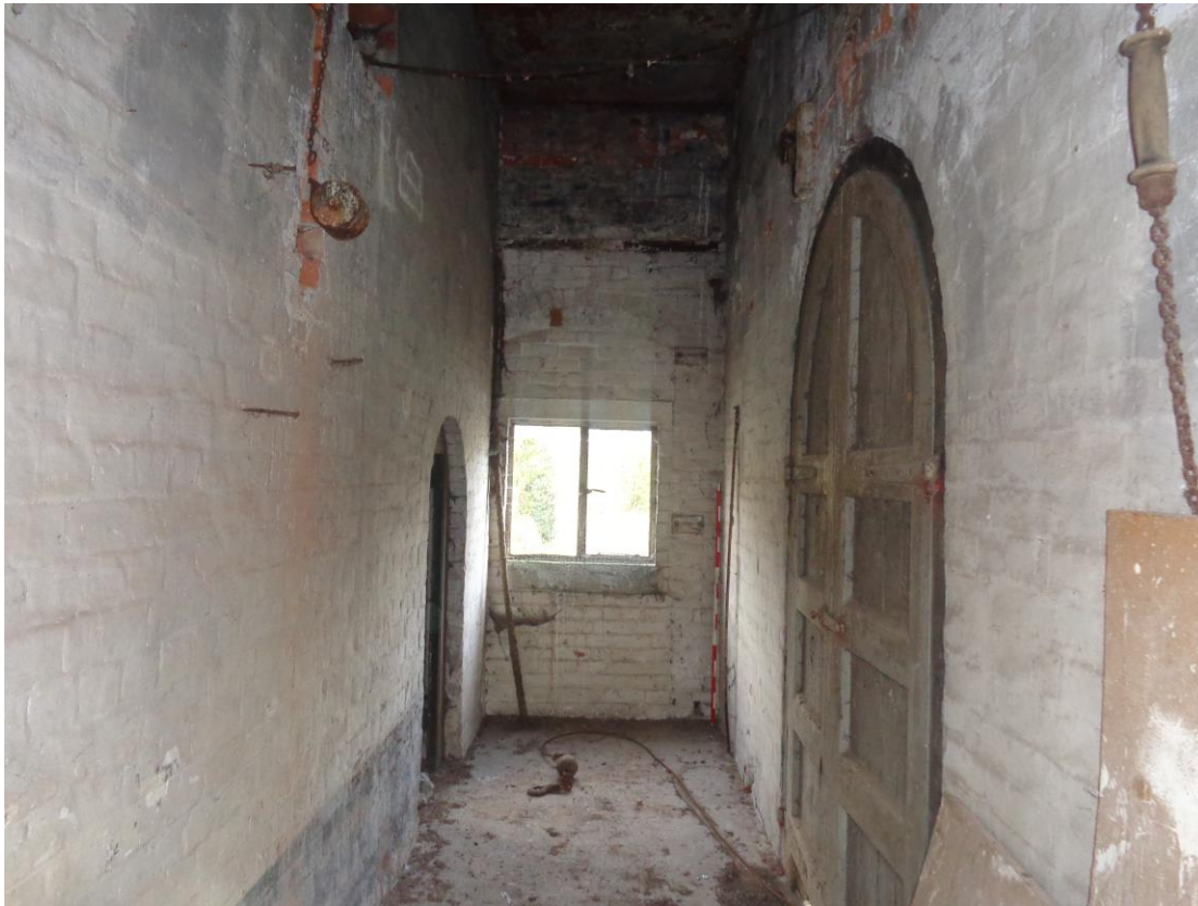
Plate 14; Stair-tower fourth-storey interior showing partly blocked doorway to building 7
