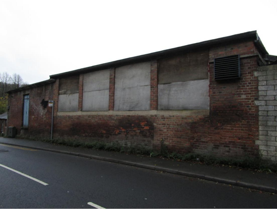
Plate 46; Buildings 7 and 9 from north-east, road-frontage
