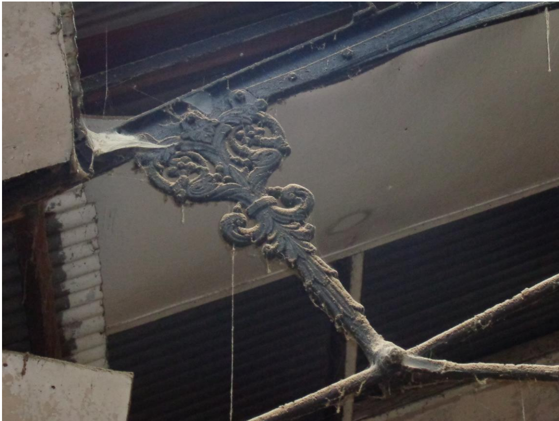
Plate 6; Building 2 roof detail
