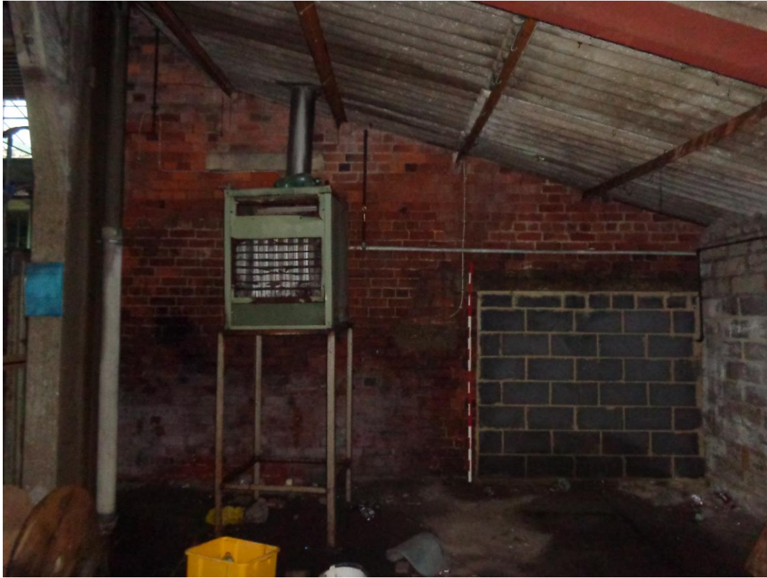
Plate 44; Building 9 north wall detail from covered-yard
