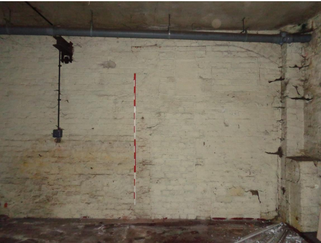
Plate 27; Building 7 cross-wall from east showing blocked doorway
