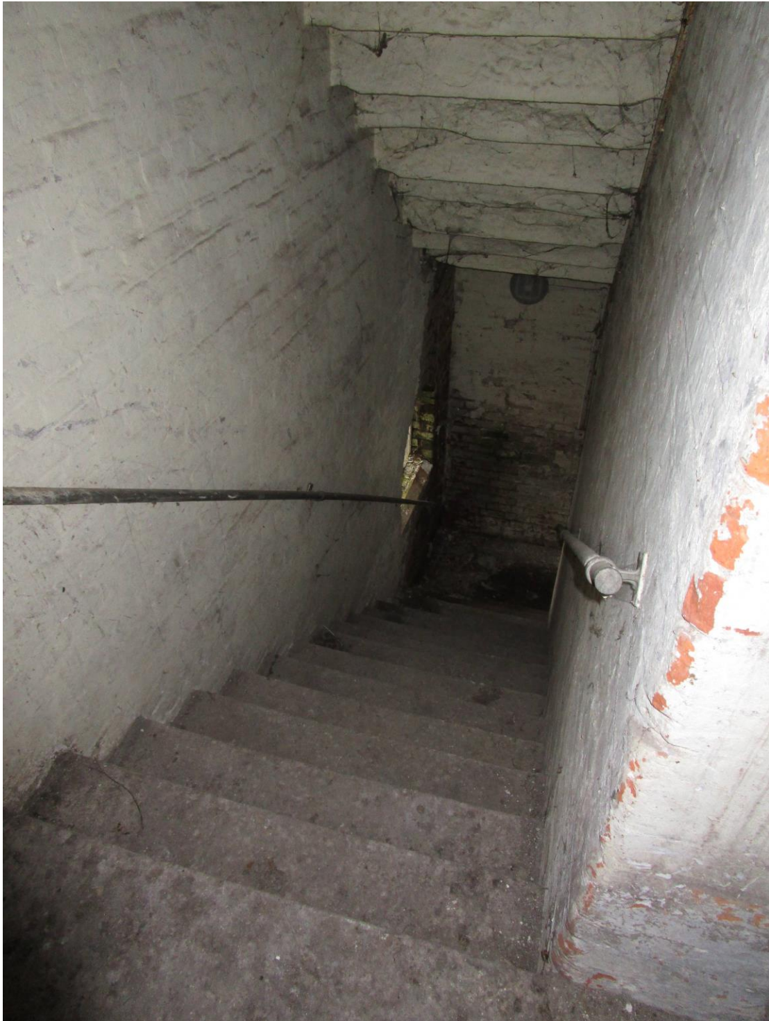
Plate 18; Stair-tower; third storey stair from south
