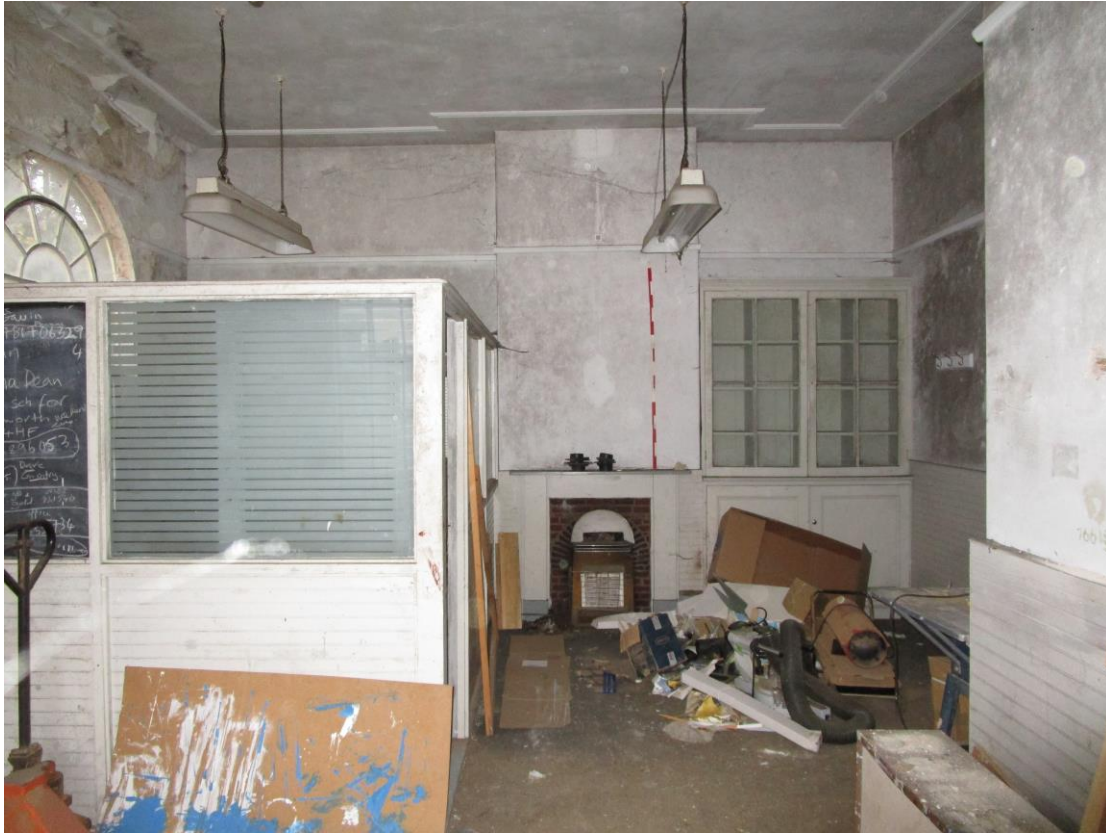
Plate 2; Building 1 interior from north
