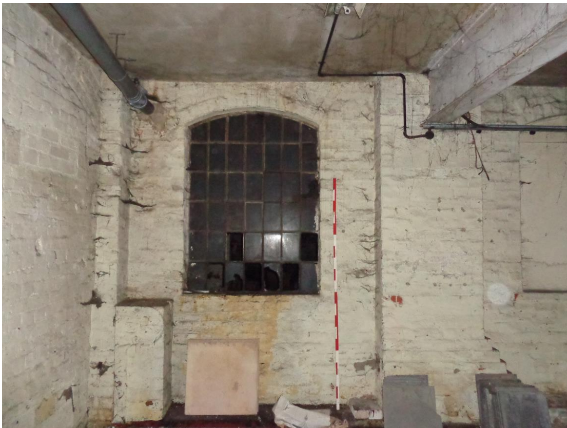
Plate 29; Building 7 north wall interior adjacent to cross-wall
