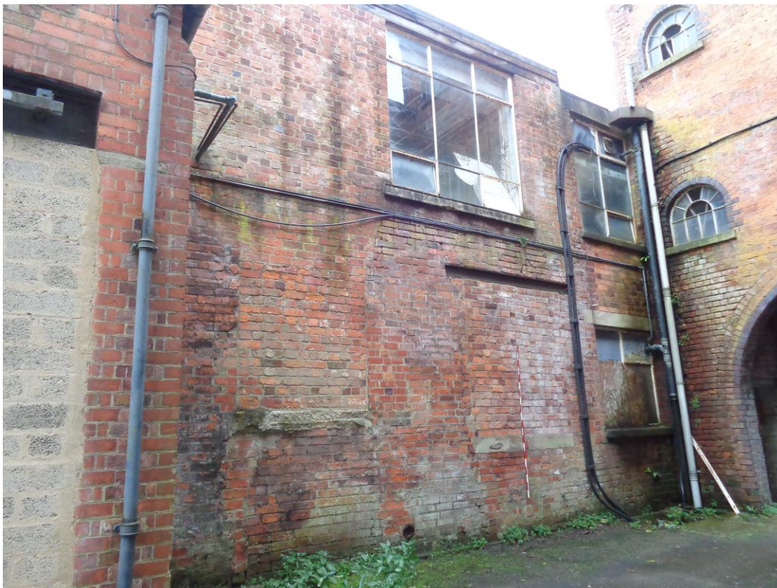
Plate 31; Building 7 west end from south showing blocked door, left, and window
