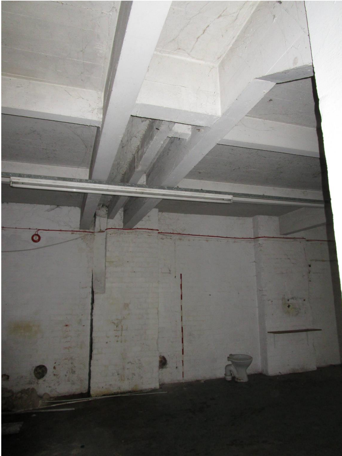
Plate 10; Building 3 first-floor interior showing inserted concrete floor and cut-back fabric to accommodate belt-wheel.
