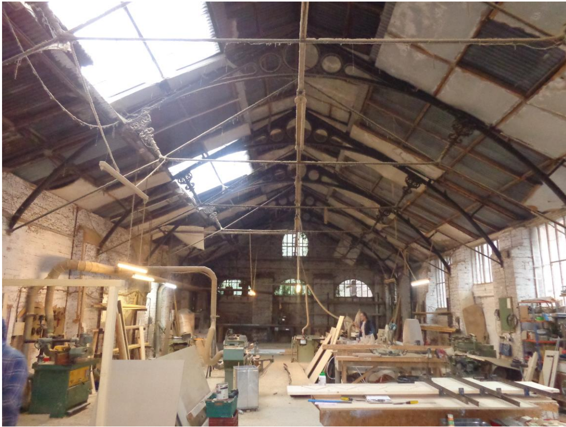
Plate 4; Building 2 interior from east
