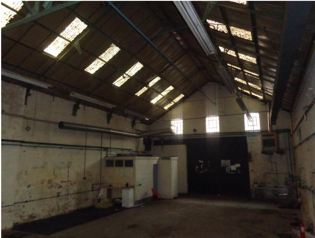
Plate 36; Building 8 interior from north-west showing west (masonry) end of building 7
