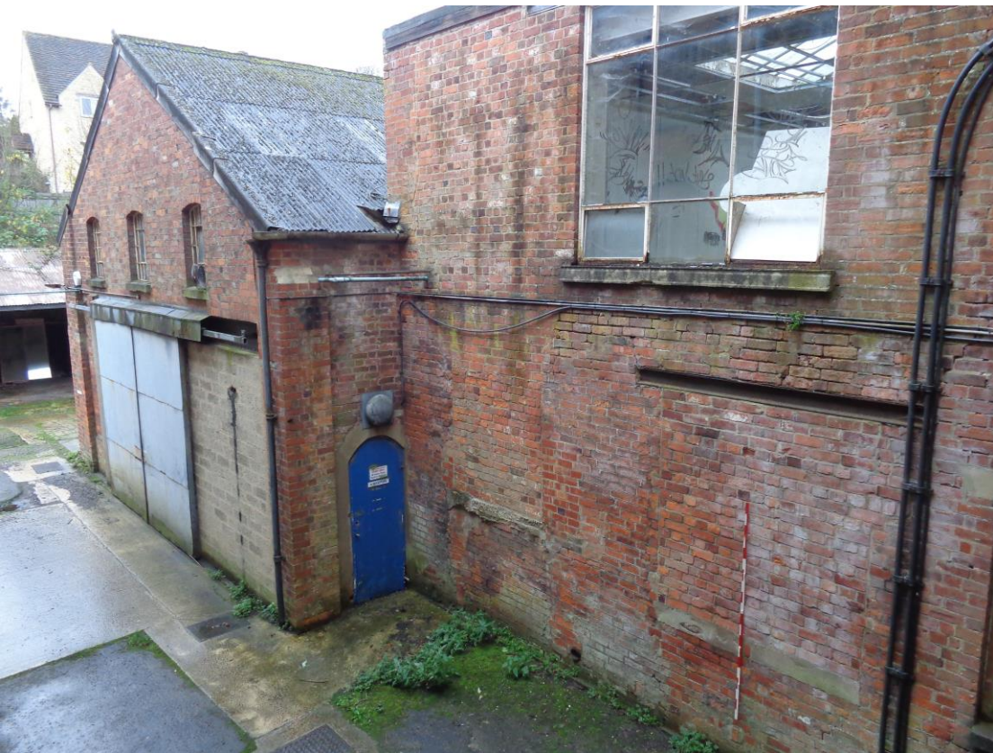
Plate 33; Building 8, and 7, from south-east
