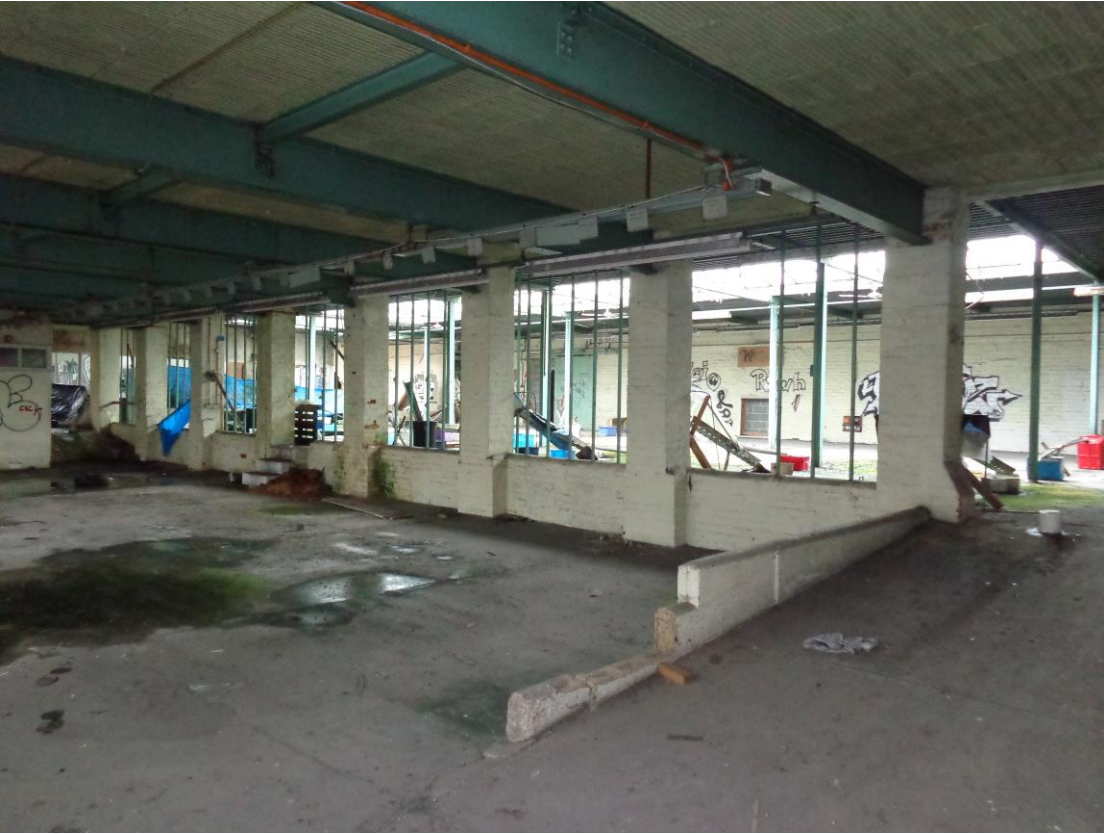
Plate 32; First floor interior of buildings 7 and 9 from south-east
