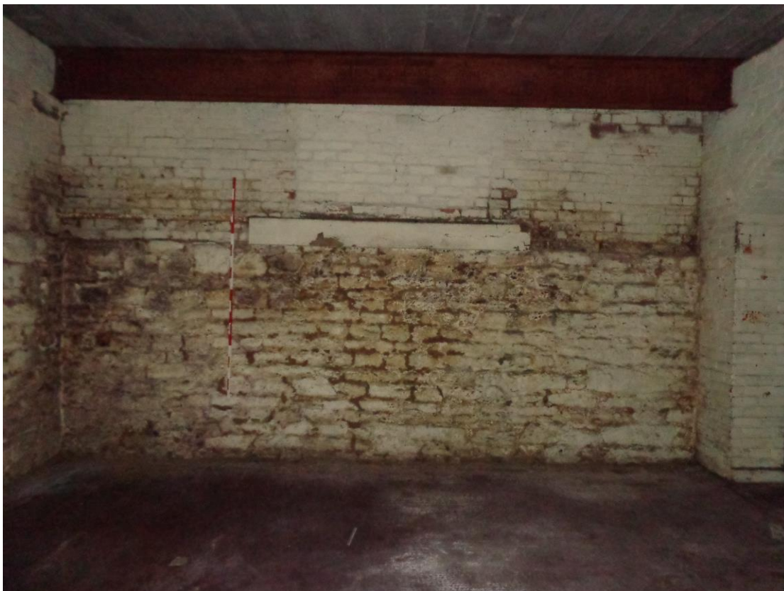
Plate 39; Building 9 interior showing masonry footings and blocked east door
