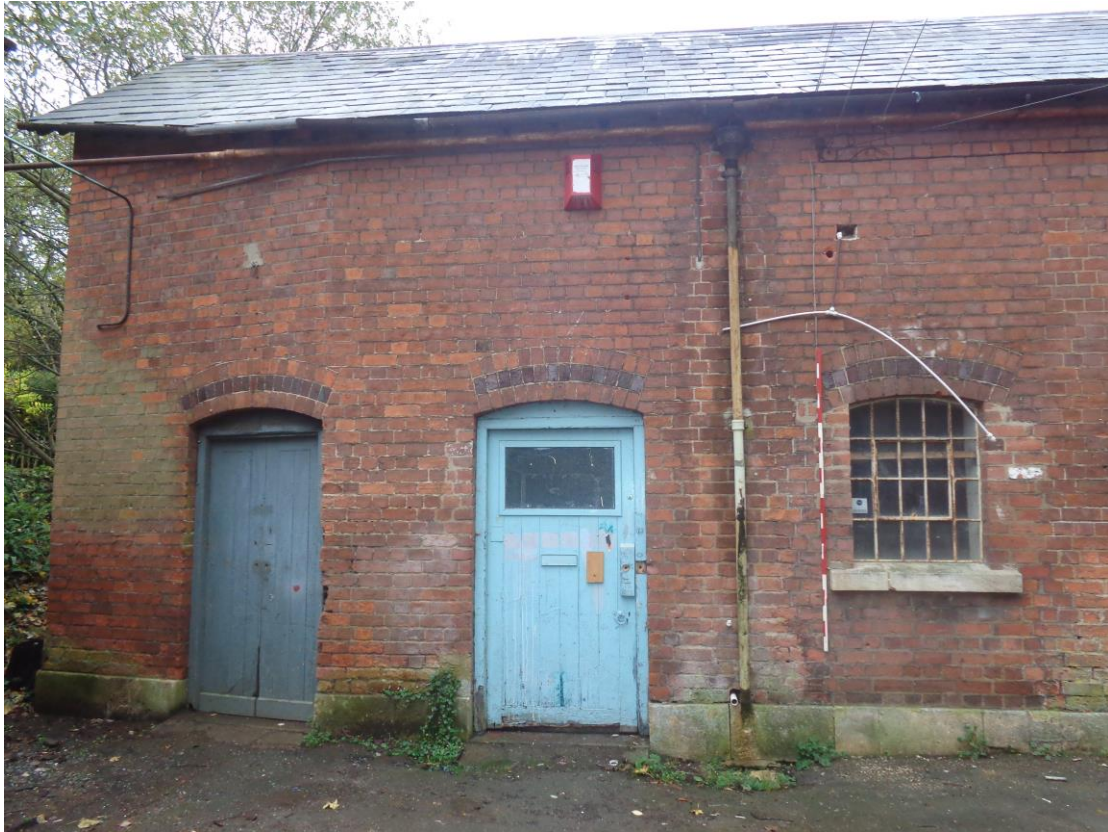
Plate 22; Building 4 (?stable)from east showing modified door and window
