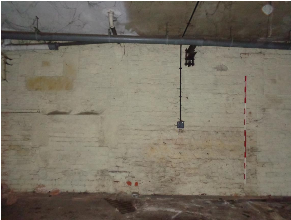
Plate 28; Building 7 cross-wall from east showing blocked masonry features
