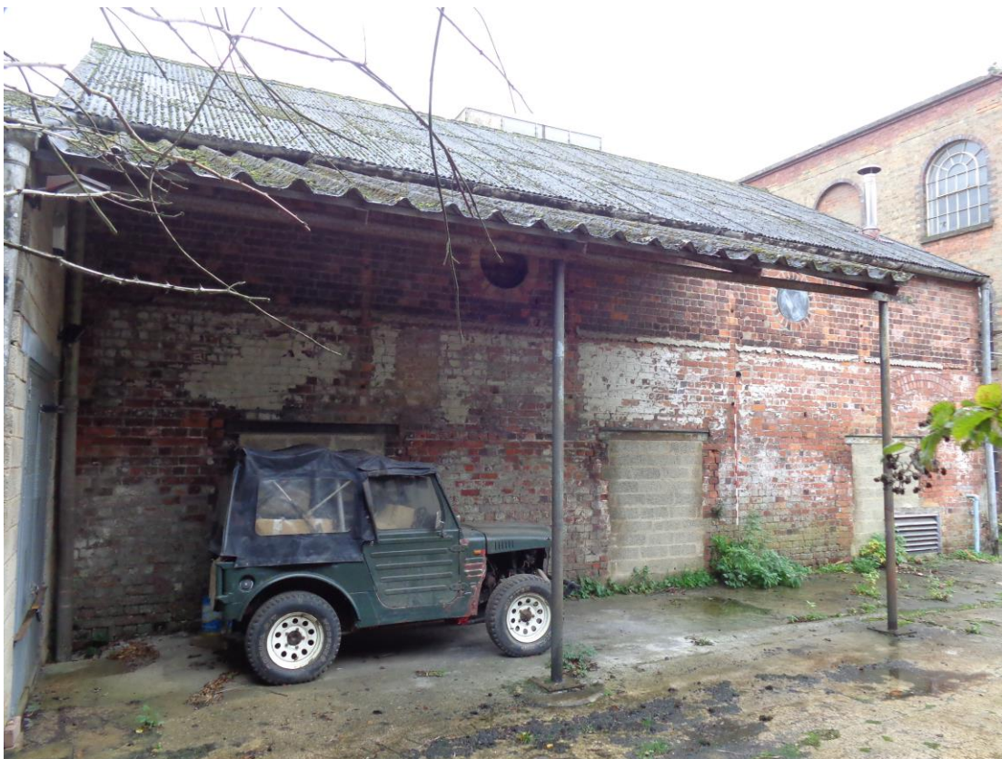
Plate 35; Building 8 from west, the round holes are inserted
