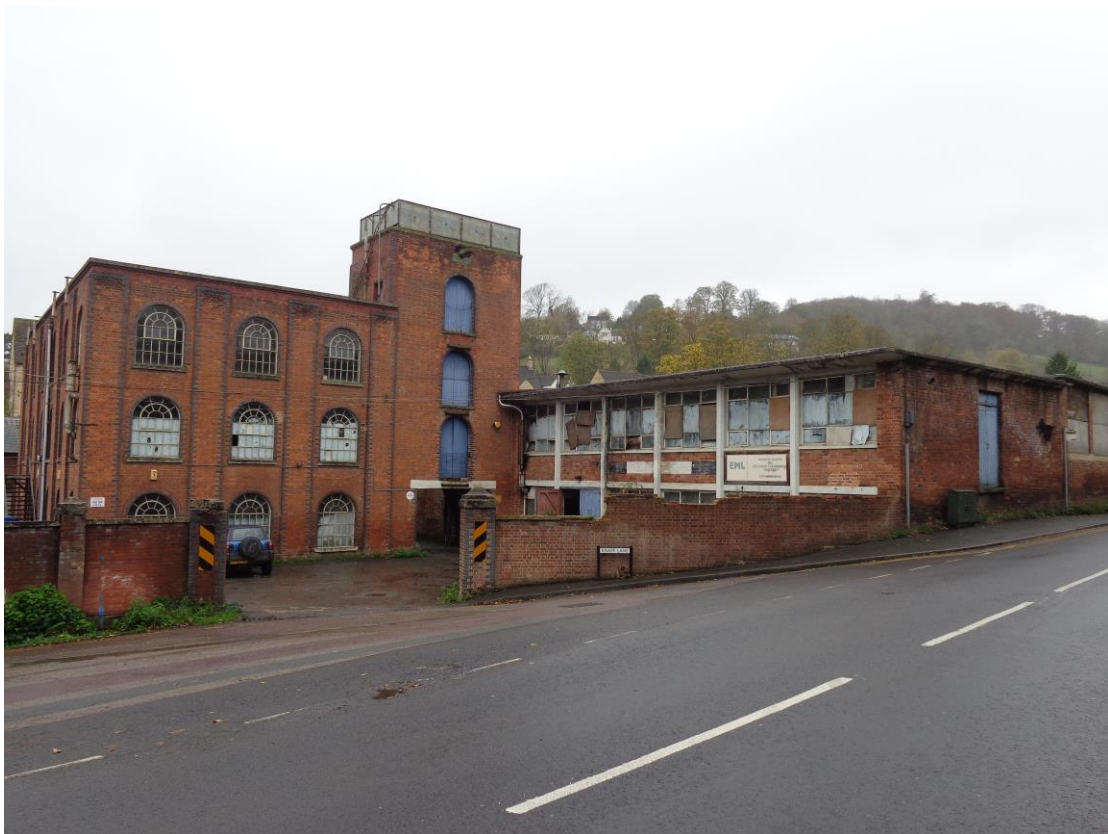
Plate 7; View of mill buildings from south-east
