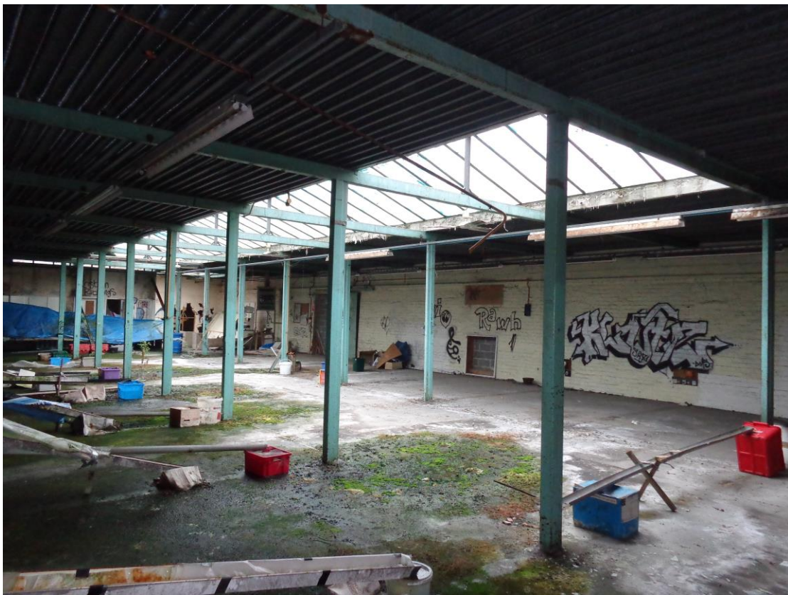
Plate 41; Building 9 1 st floor interior from south-east
