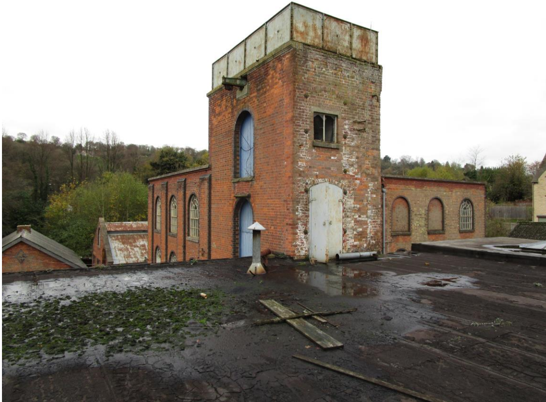
Plate 12; Top of building 3 and stair-tower from north-east
