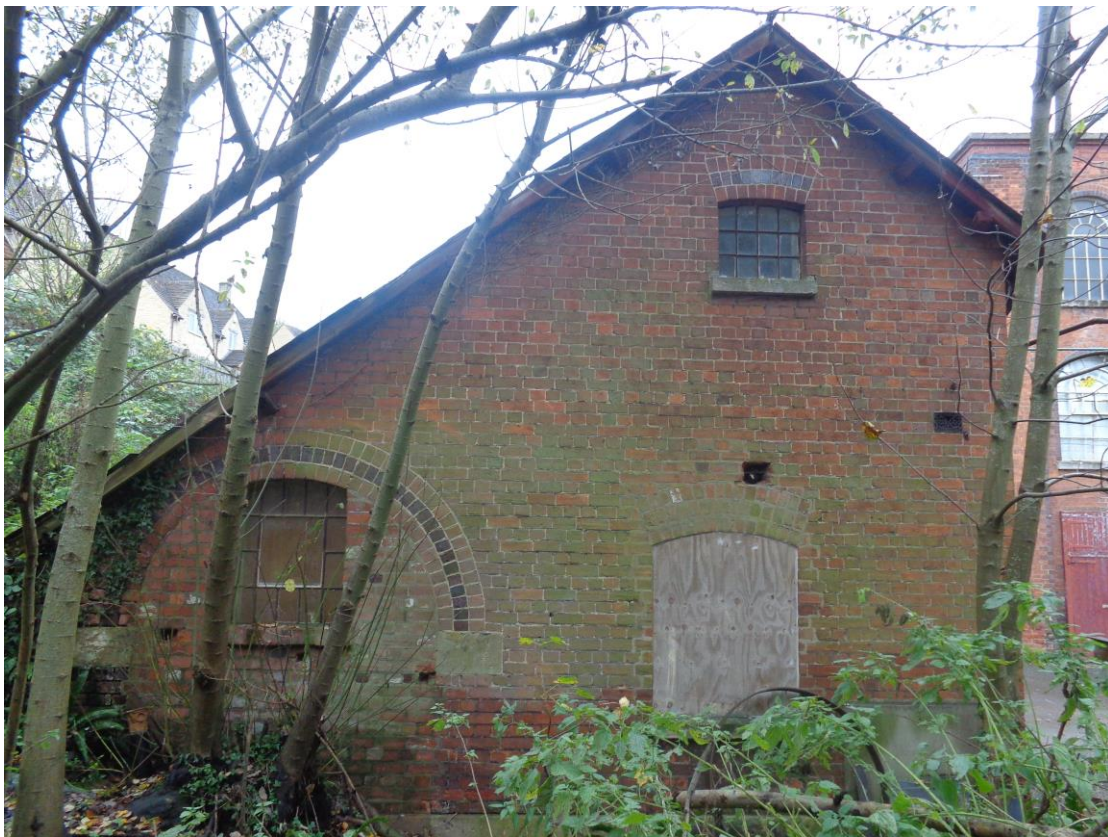
Plate 23; Building 4 (?stable) from south showing blocked arch (?cart-shed)
