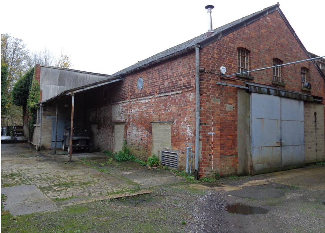
Plate 34; Building 8, and 10 beyond, from south-west showing blocked and inserted features, and remains of lost lean-to
