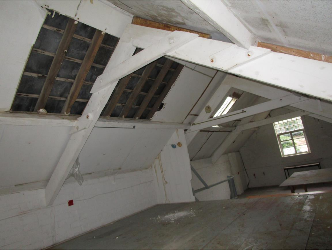
Plate 24; Building 4 ?former hayloft from raised south end
