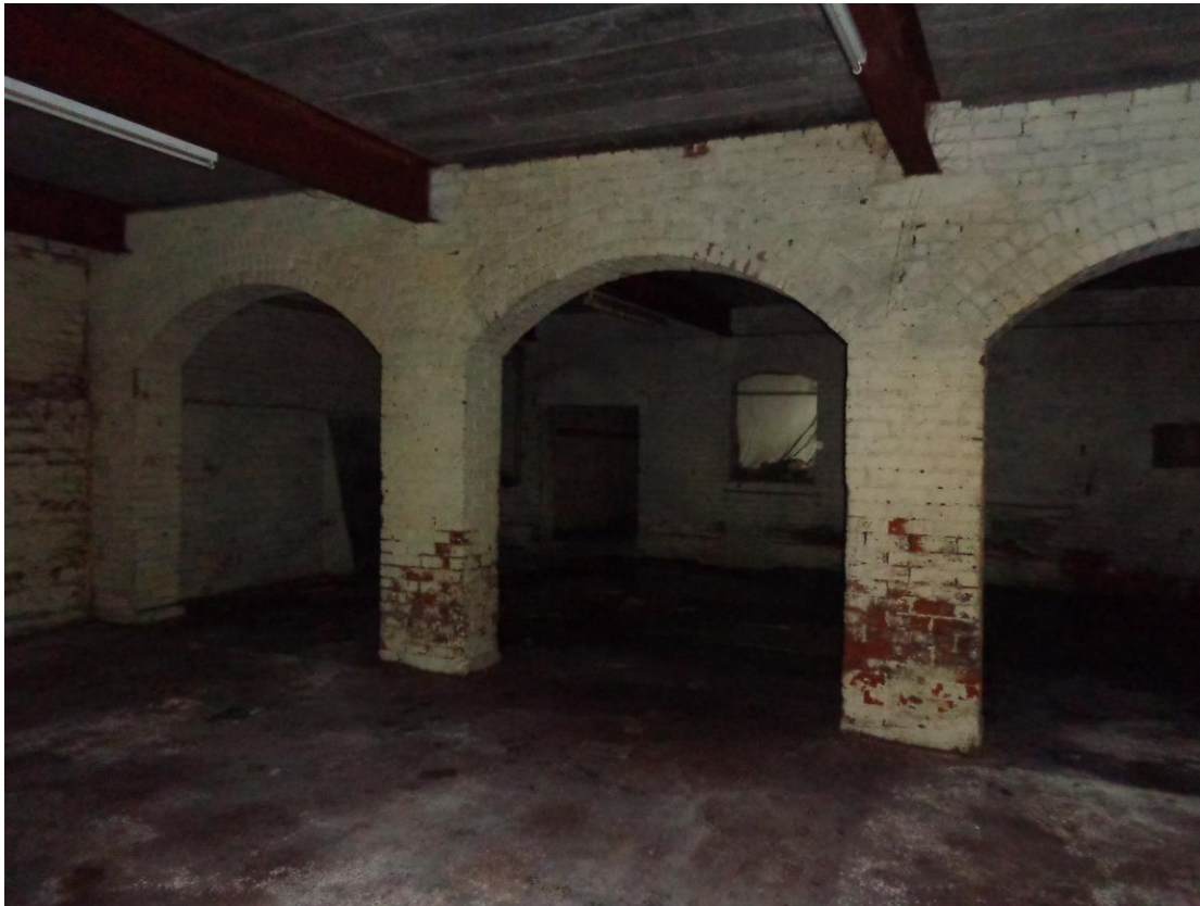
Plate 38; Building 9 interior and building 7 beyond from north-west
