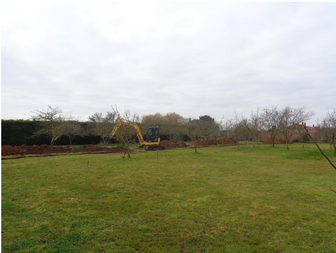
Plate 8; trenches 1 & 2, from the north-east
