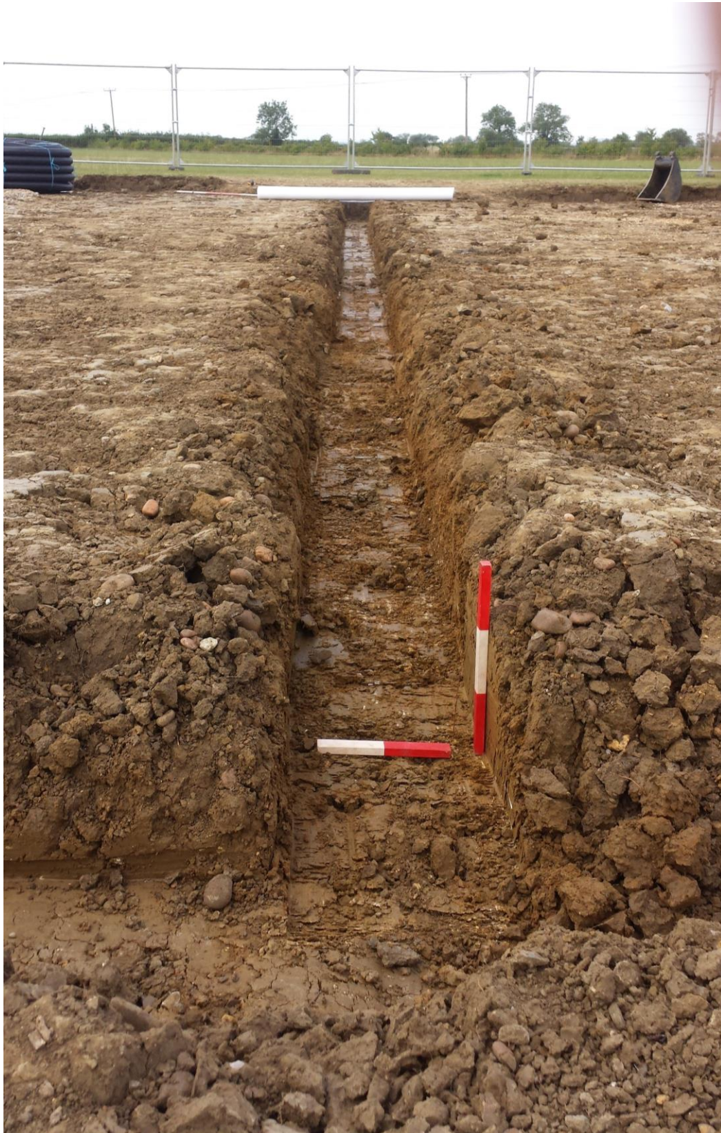
Plate 5; trench 2, soakaway trench, from the north-east
