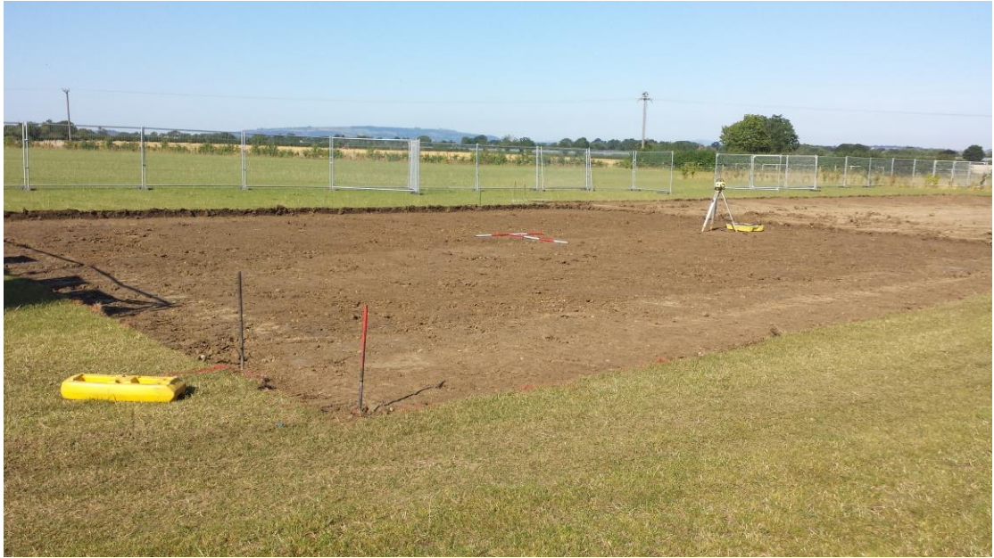
Plate 3; trench 2 south-east half, from the east
