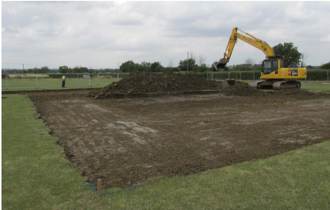
Plate 1; trench 1 under excavation, from the south-east
