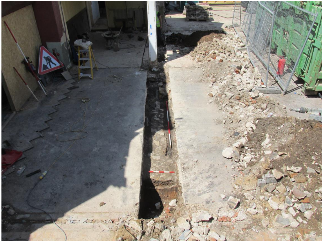
Plate 1; trench 1c, showing context (wall) 104, from the east
