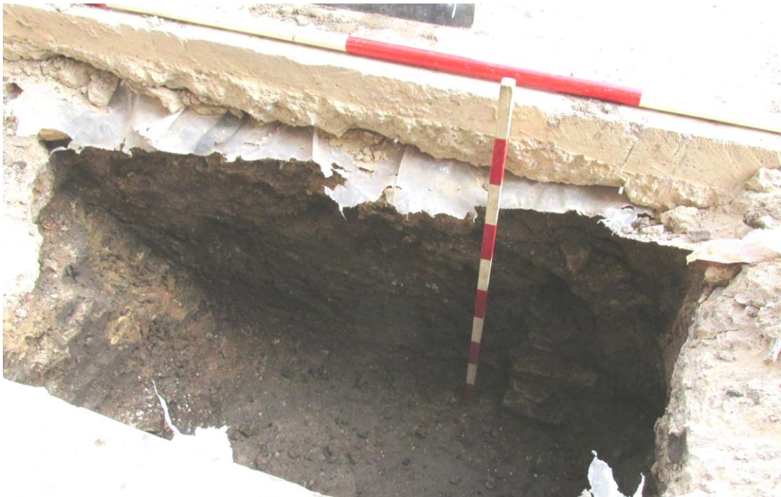
Plate 6; trench 1b with wall 108 to the right of the scale, from the south-east
