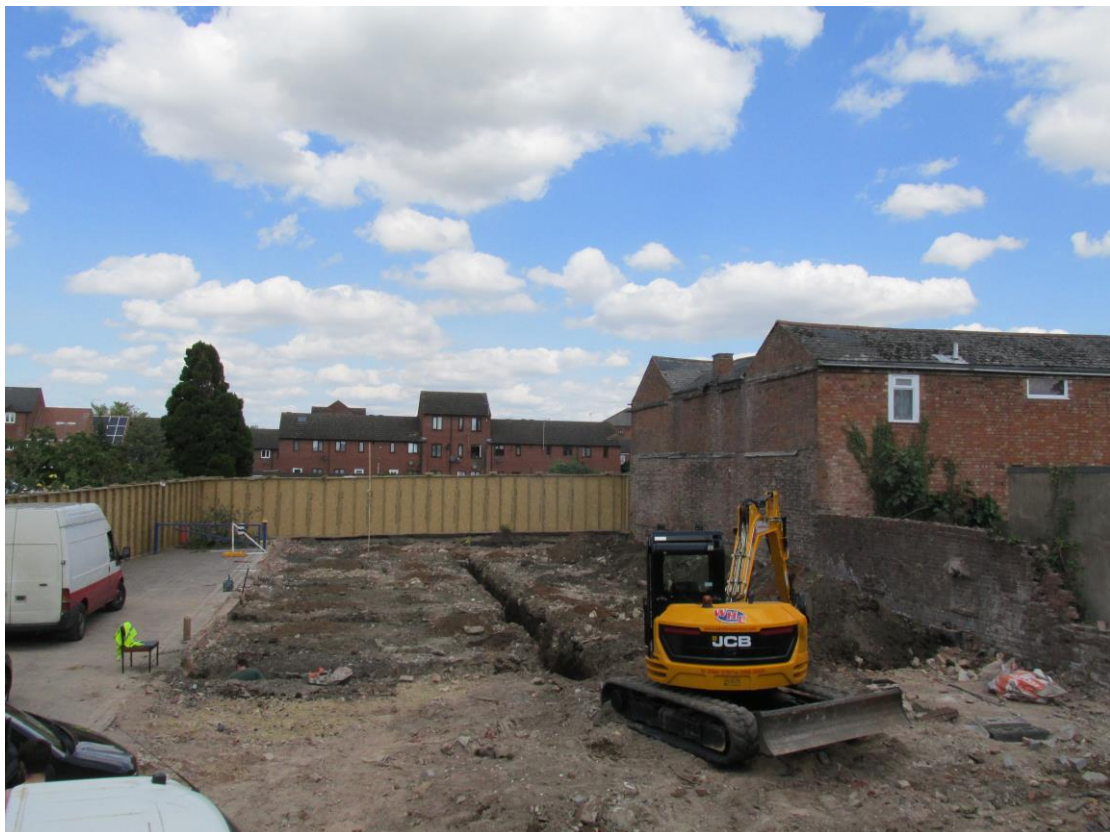
Plate 10; overall view of trench 2, from the south
