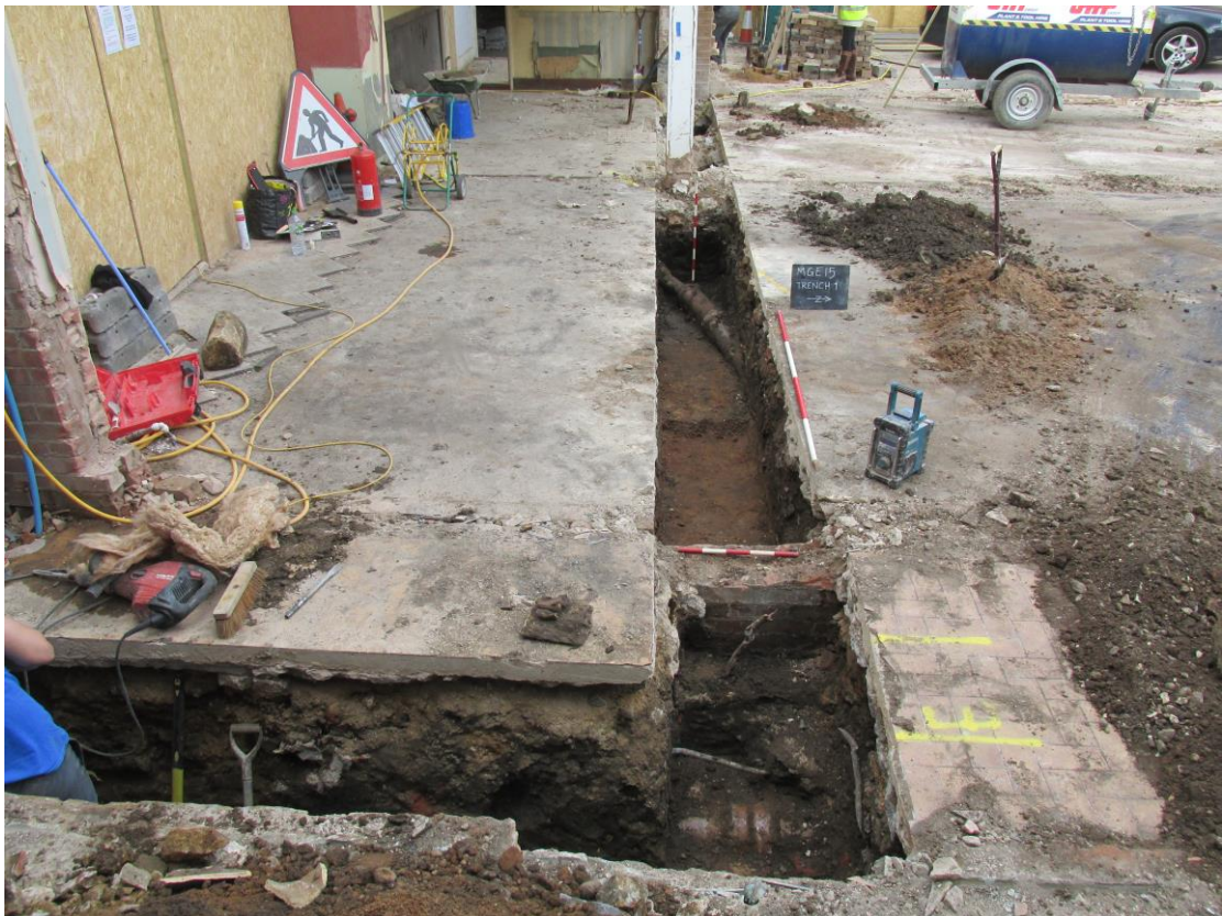
Plate 3; trench 1c fully excavated, from the east
