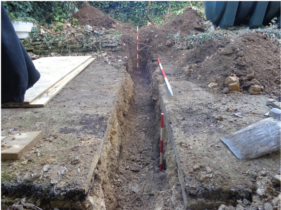
Plate 7; gas trench, from the west
