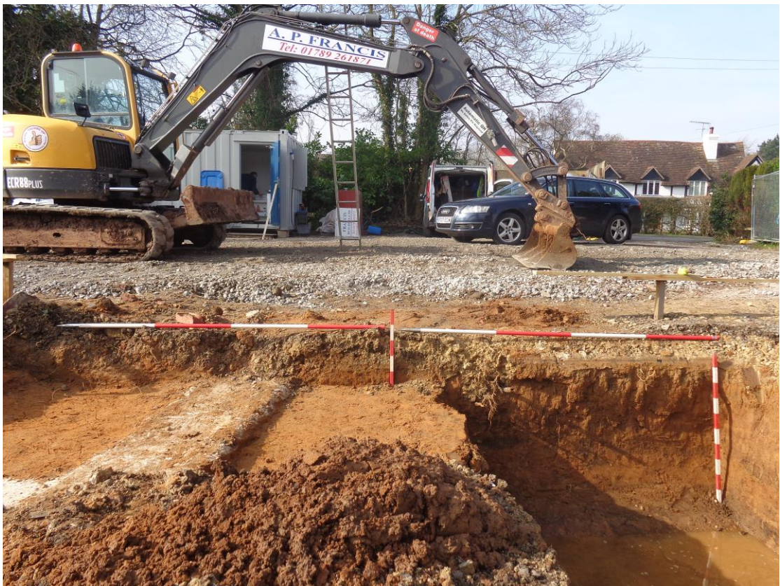
Plate 2; section 1a, from the east
