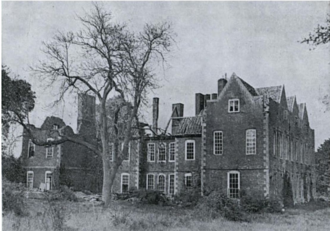
Fig. 8; Park House from south-east during demolition (1960s), showing the brickwork and distinctive quoins of the 1702 rebuild. The massive chimney, to the left of the tree, belongs to the Elizabethan service-wing.
