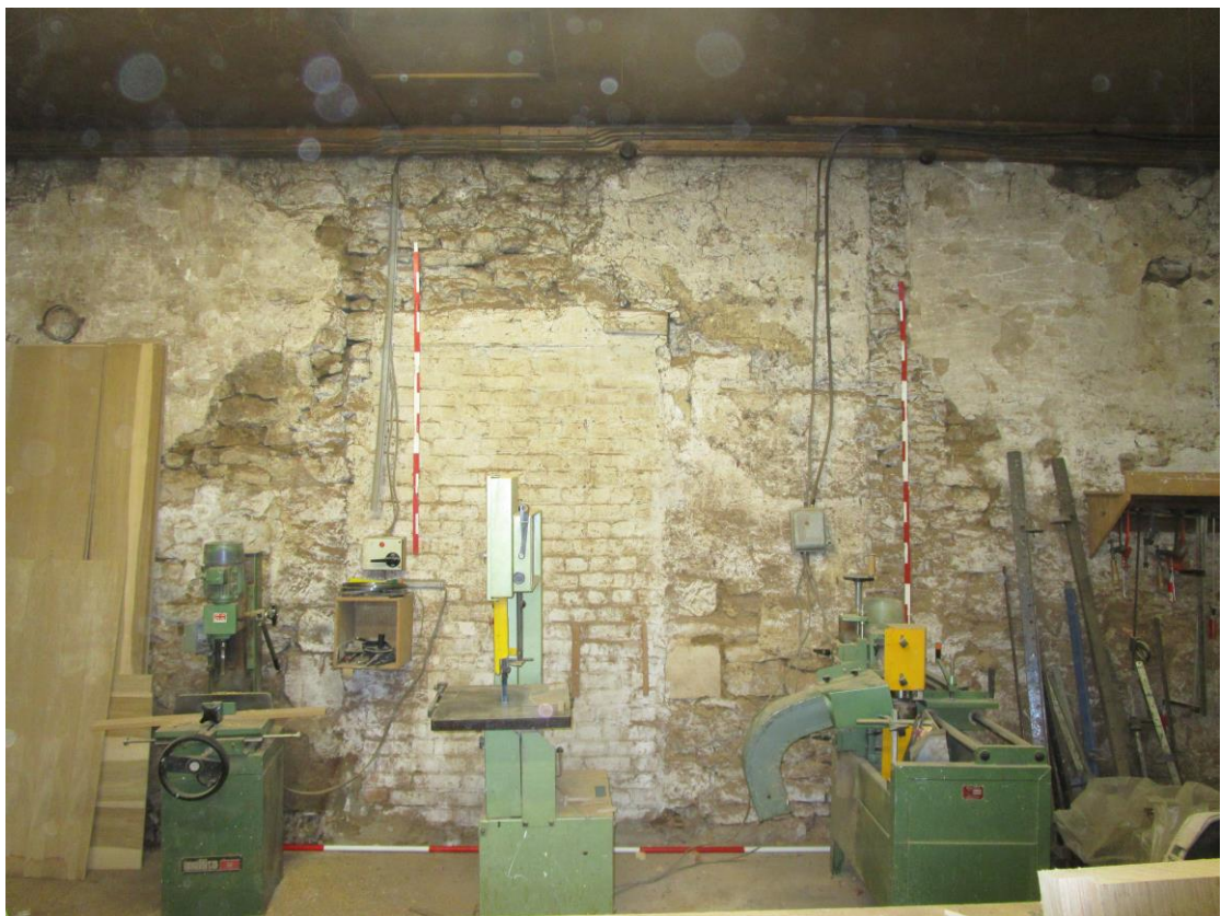
Plate 8; west wall interior centre
