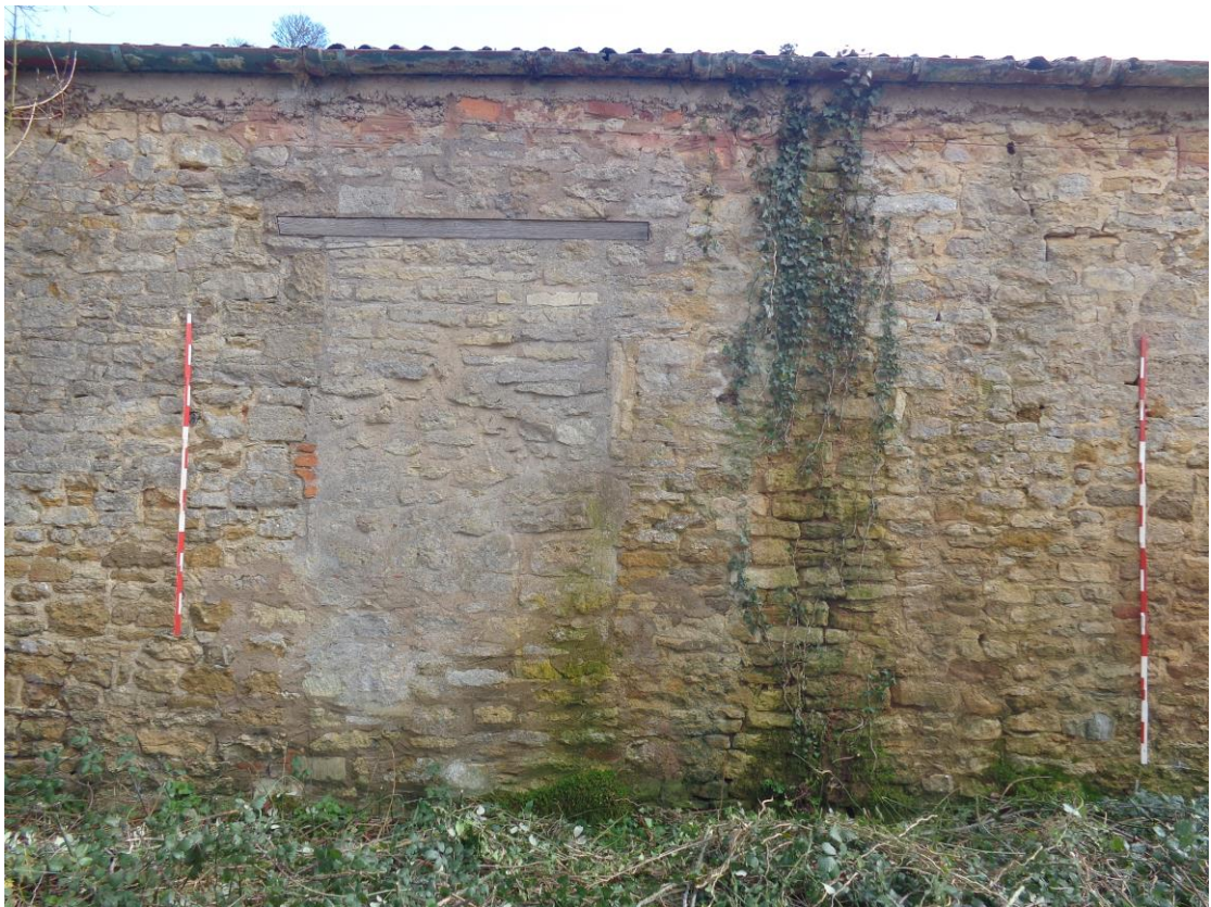
Plate 6; west elevation north end
