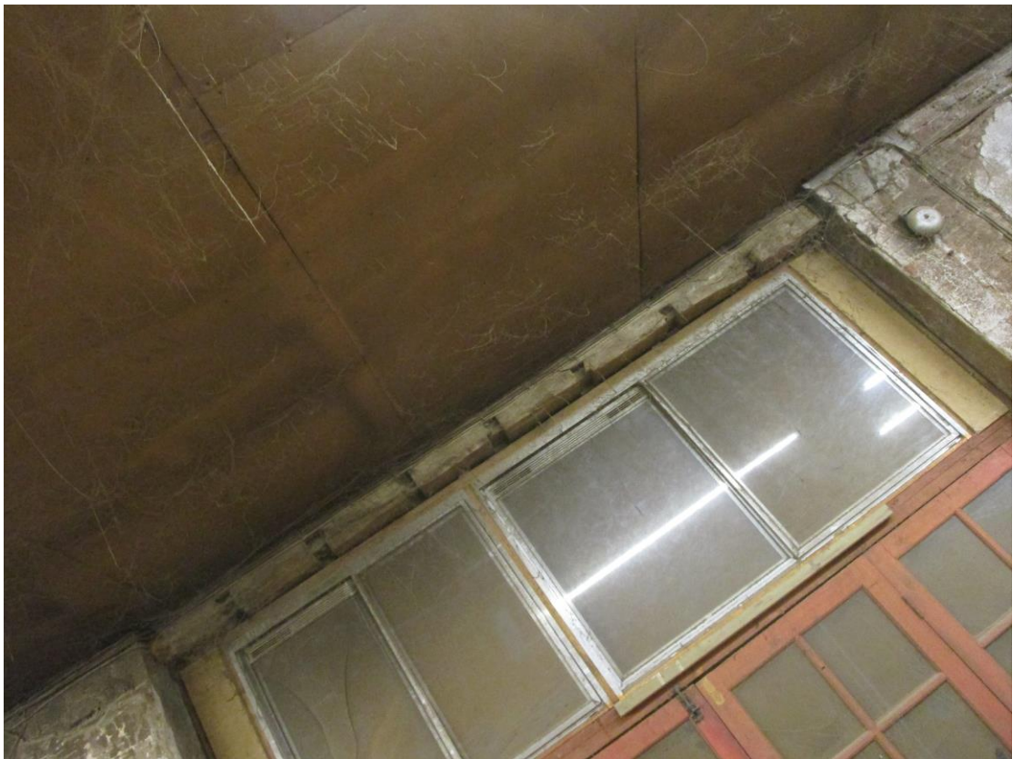
Plate16; main range interior from west showing re-used principal-joist
