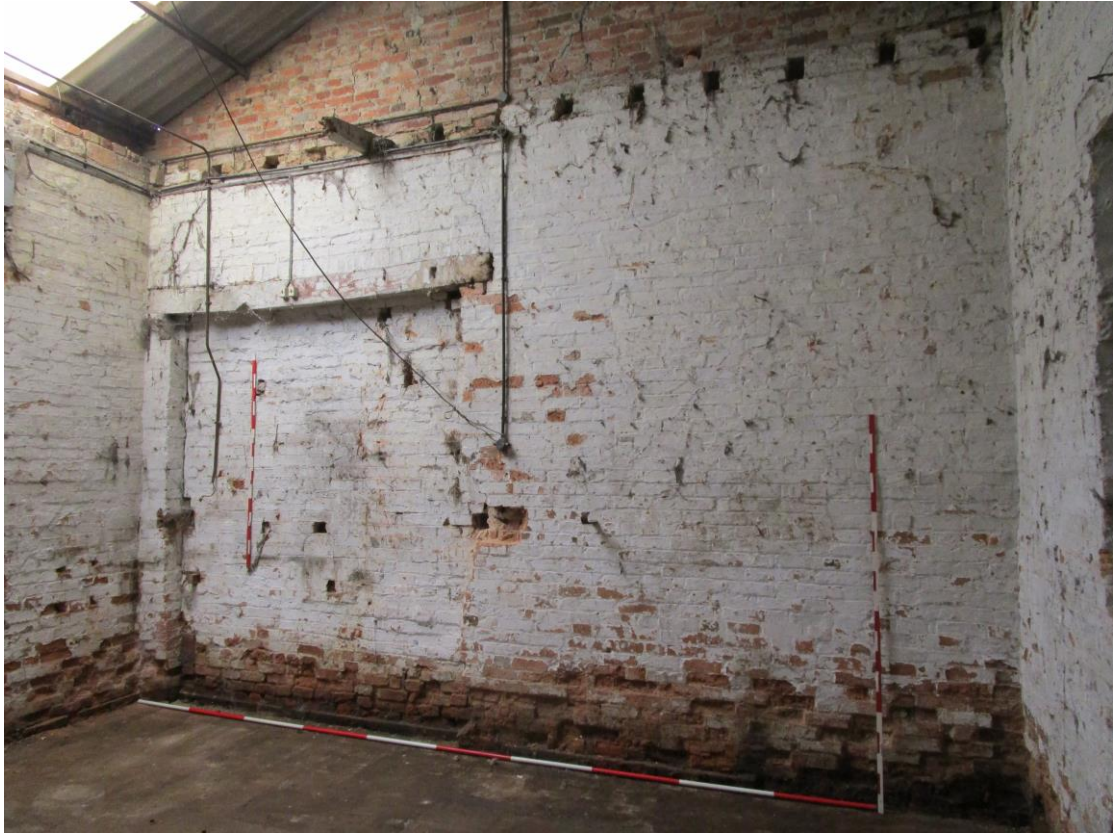
Plate11; south-wing east wall interior
