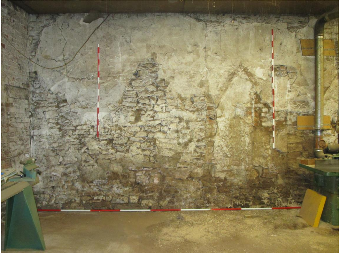
Plate 13; west wall interior south end, showing evidence for stalls
