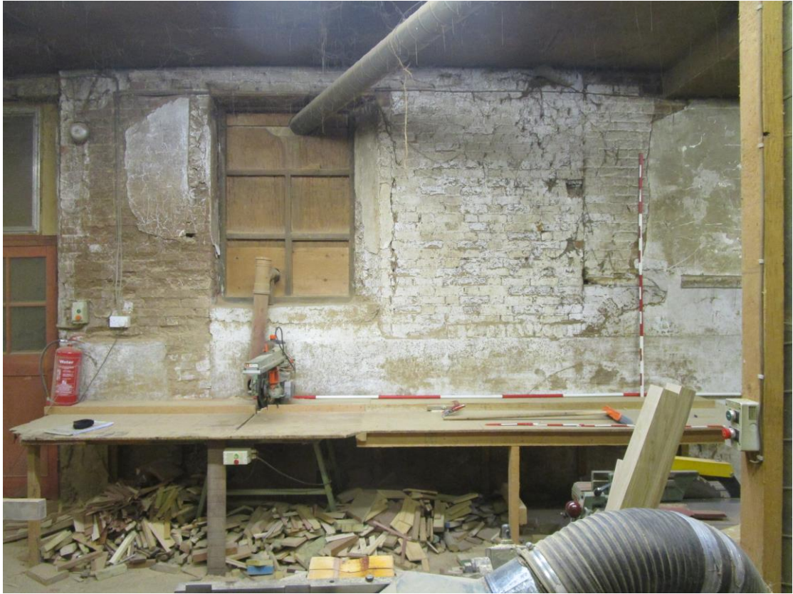
Plate 15; main range near south end interior from west
