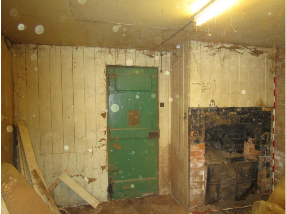
Plate 19; south-wing inserted room and fire-place from south
