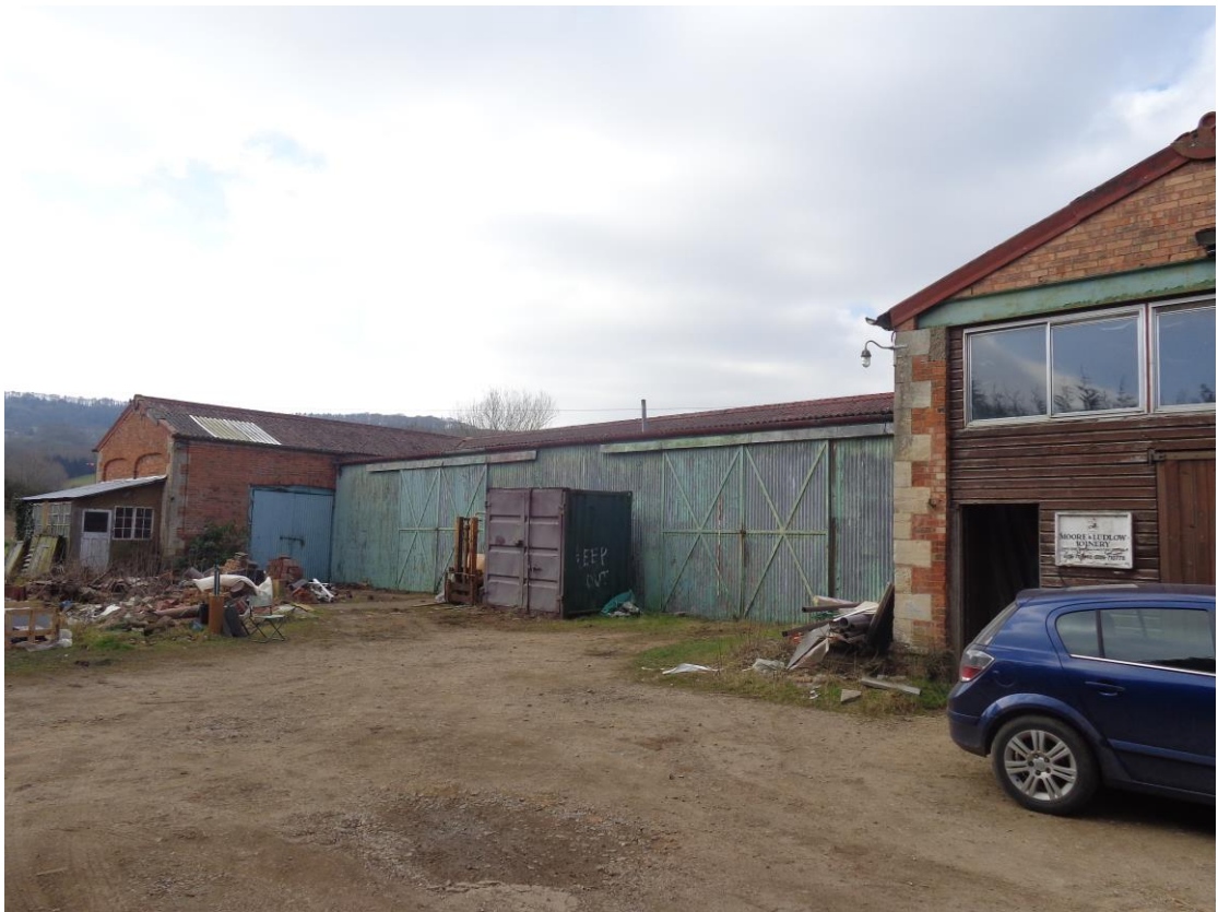
Plate 20; view from north-east
