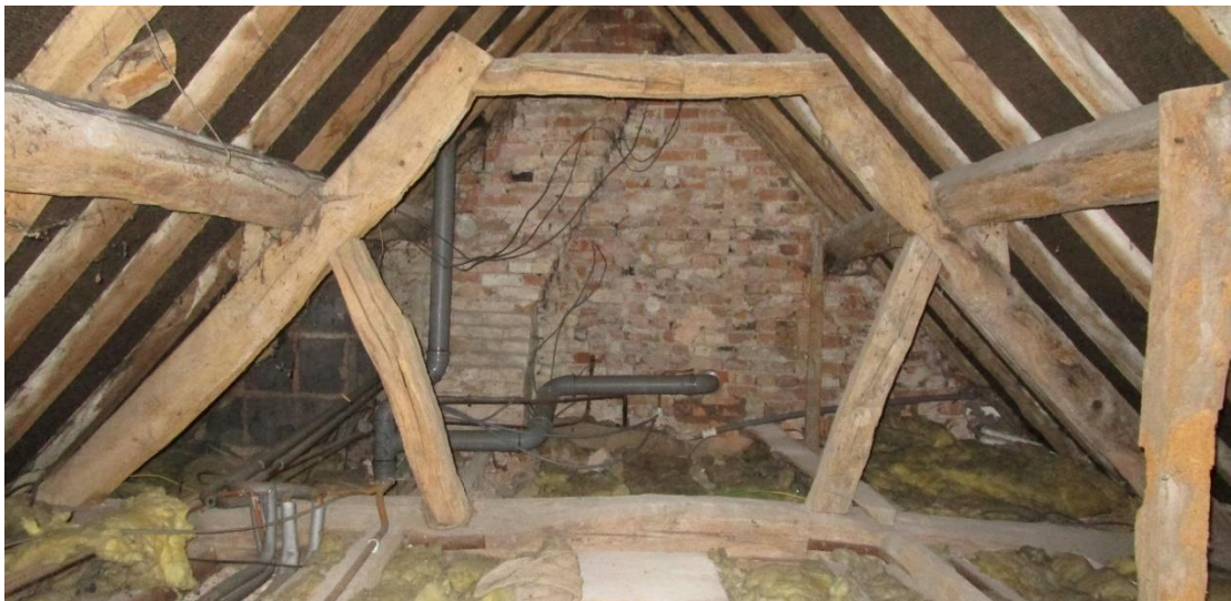
Plate 16; Roof-frame in east wing of coach-house to west
