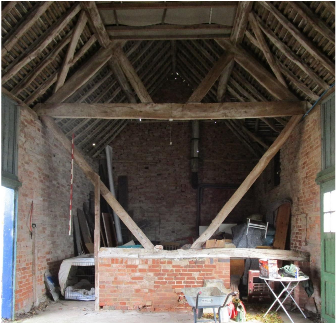
Plate 10; Brick barn, internal view to north
