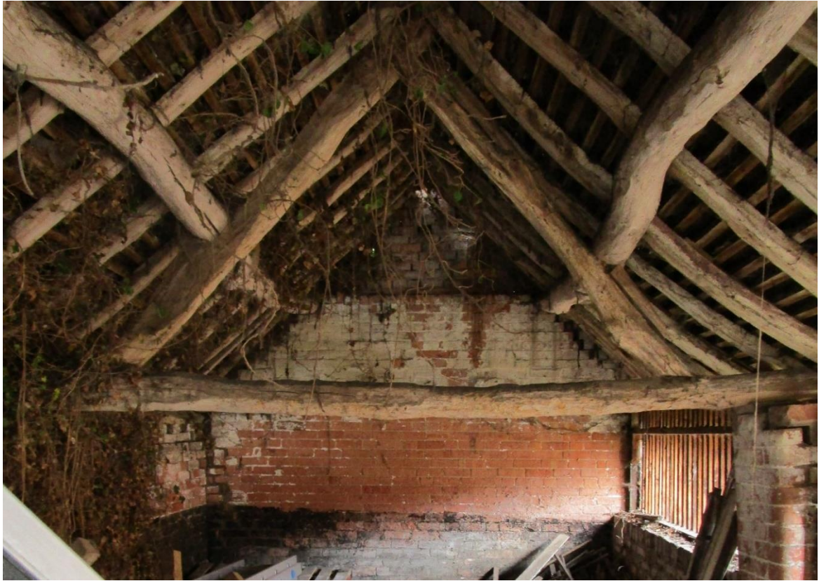
Plate 11; Open-shed, internal view to west, west end
