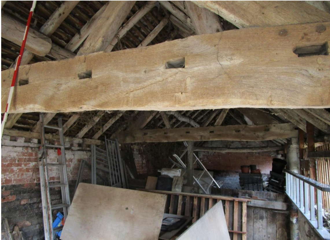
Plate 13; Open-shed, detail of re-used principal-joist
