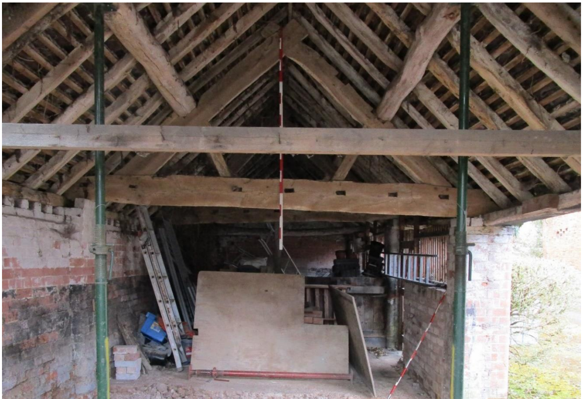
Plate 12; Open-shed, internal view to west, showing split and re-used principal joist
