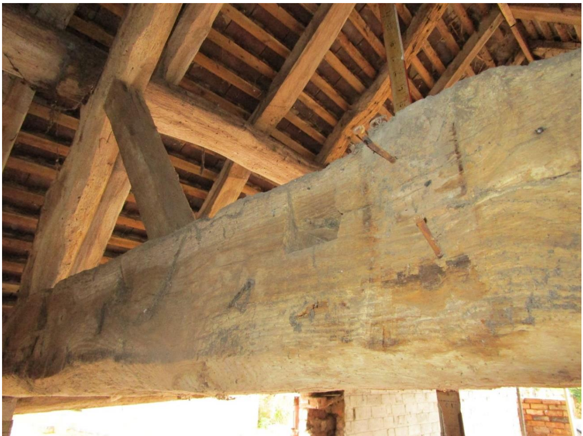
Plate 14; Open-shed, mortice with housing for diminished haunch in re-used joist
