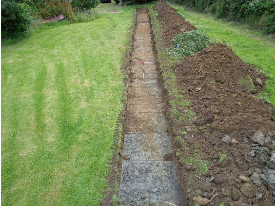
Plate 3; trench 2 from the north-west
