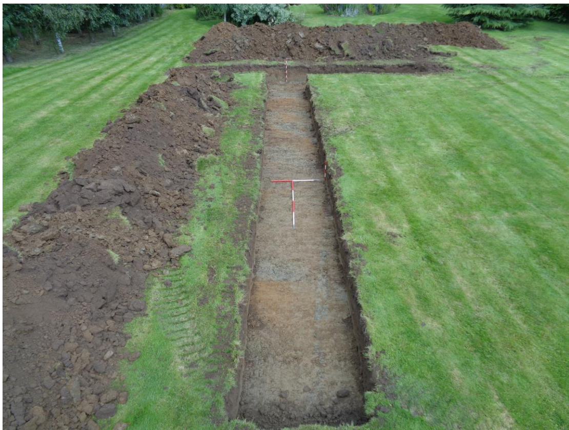
Plate 10; trench 5, from the north-west
