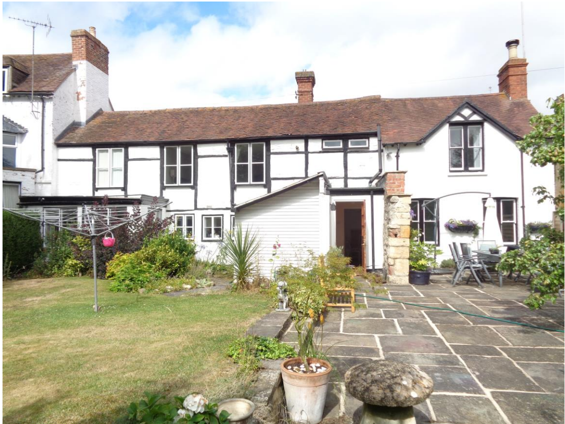
Plate 1; rear of 2 Abbey Cottages, from the south-east
