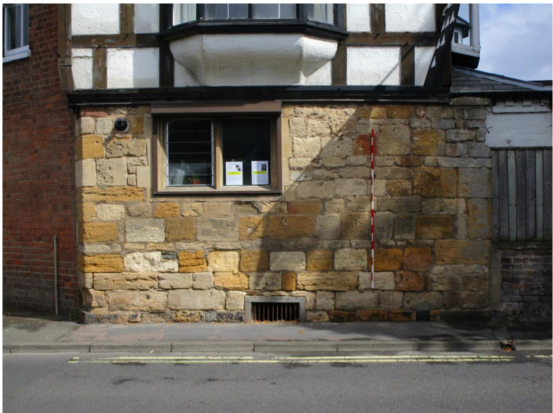
Plate 6; 1 Abbey Cottages, masonry wall at west gable end.
