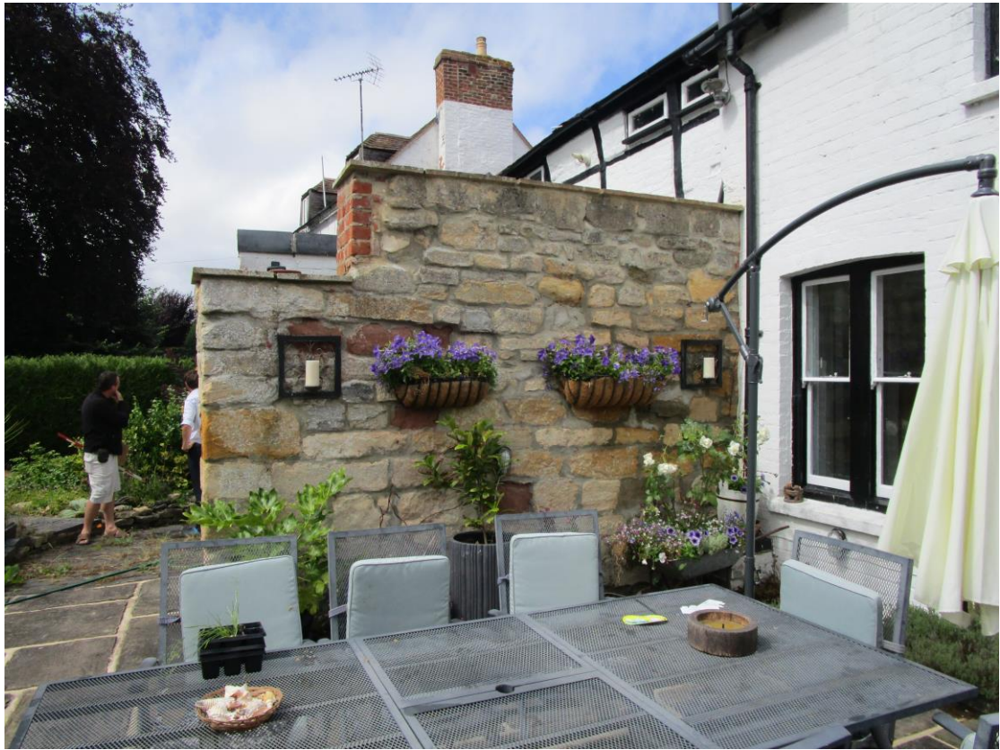
Plate 3; masonry wall in the rear garden, from the east
