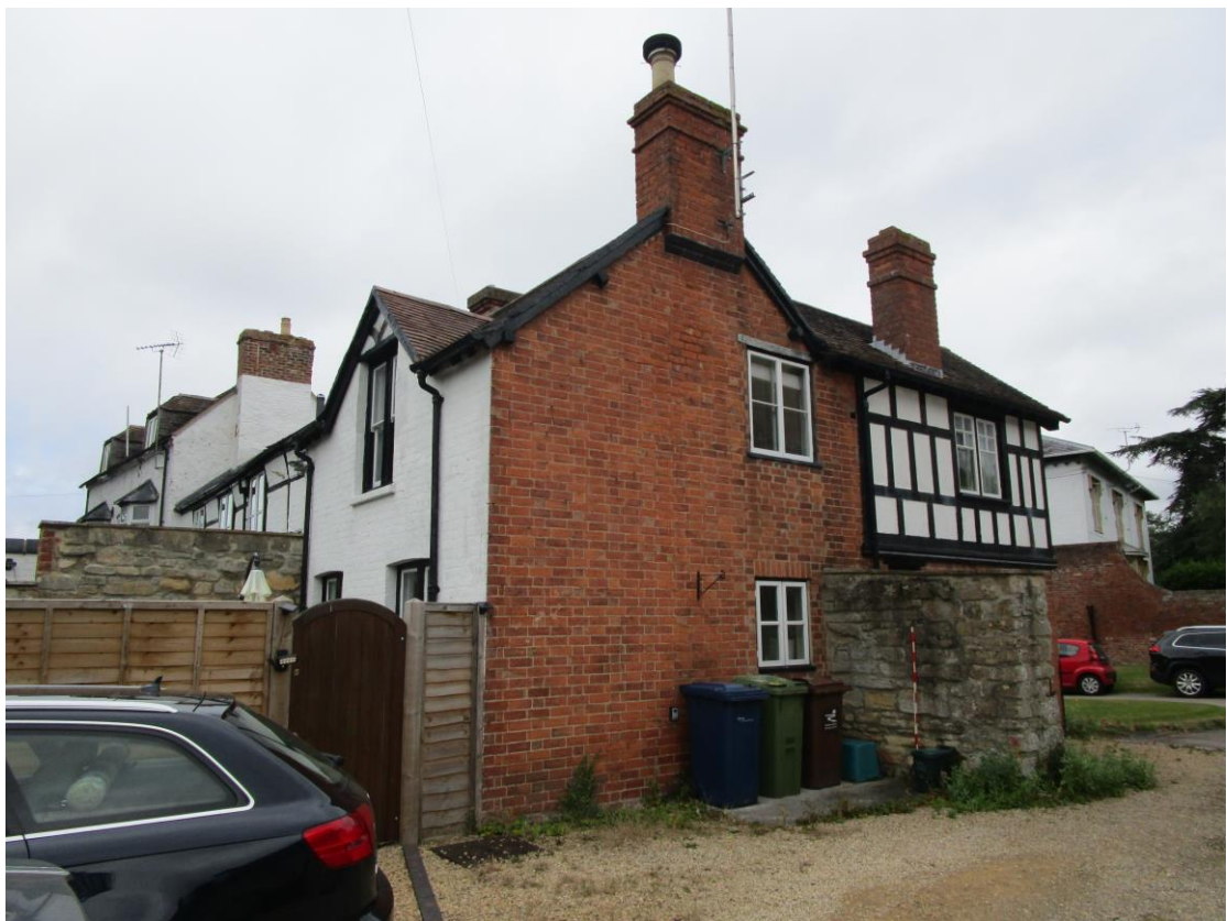
Plate 4; masonry wall at east end of the house, from the south-east
