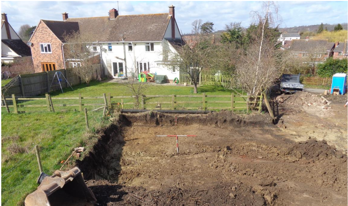
Plate 2; trench 2 excavated; from the south-west
