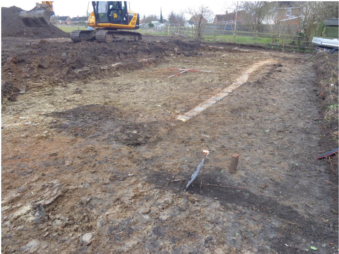
Plate 6; trench 3, from the north-east
