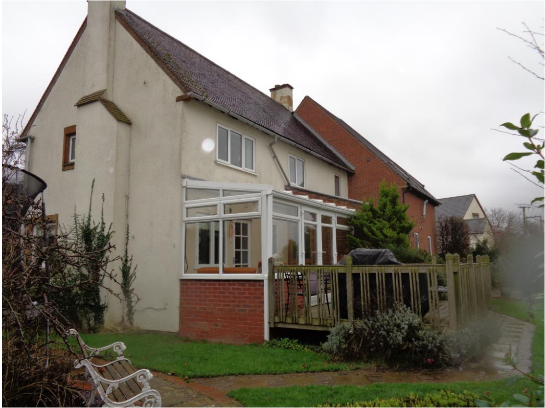
Plate 2; rear elevation showing area of proposed orangery, from the north-west
