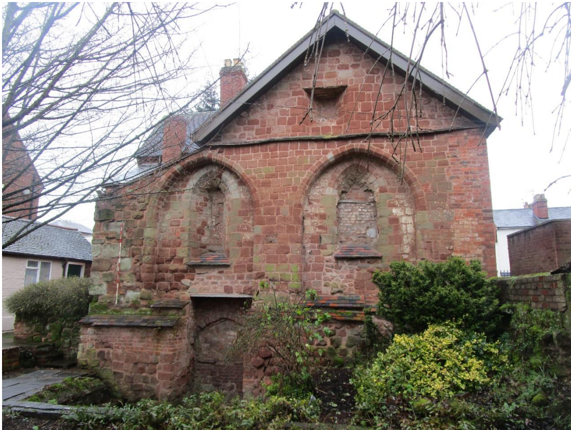
West wall view
