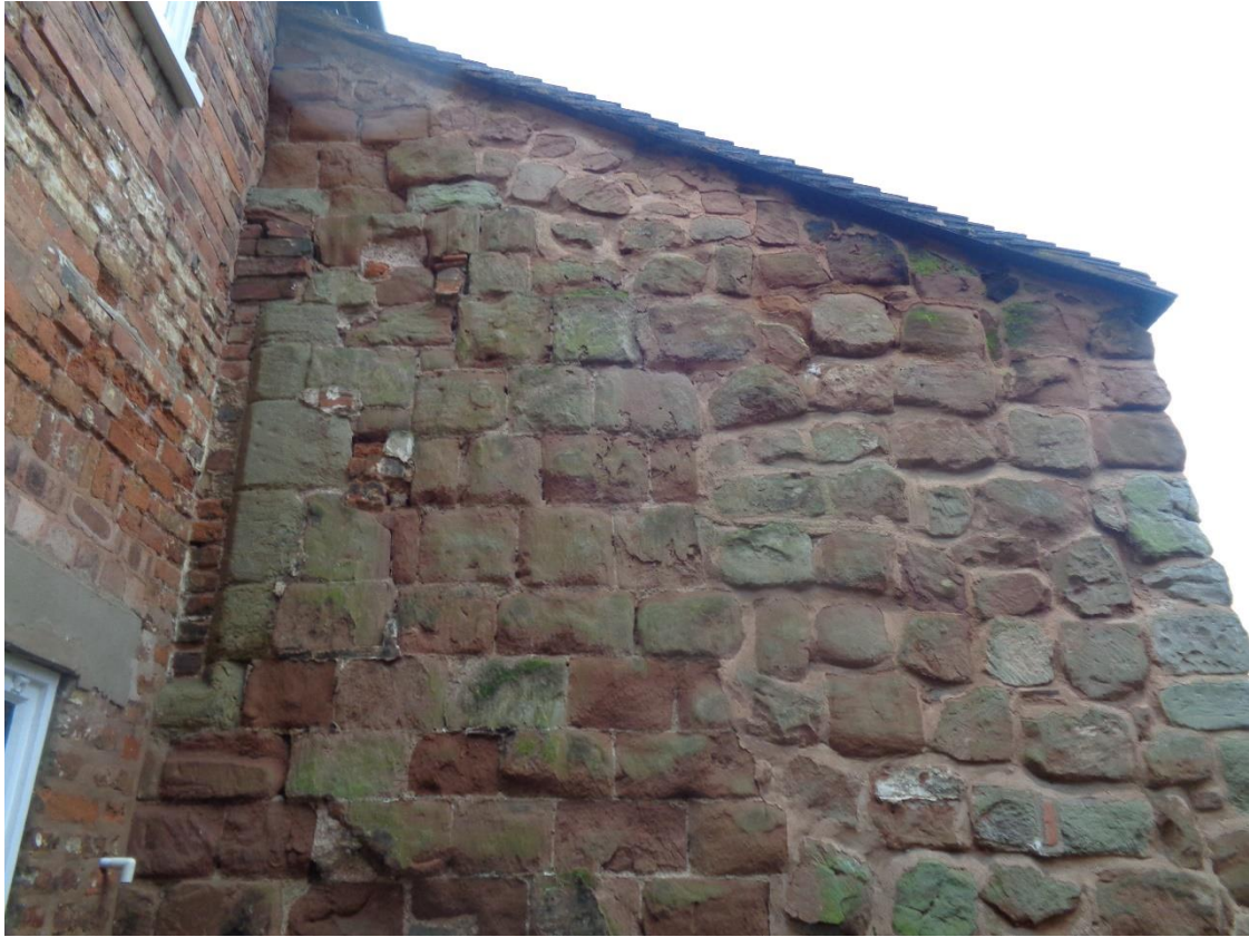
West wall exterior showing remains of C13 window.
