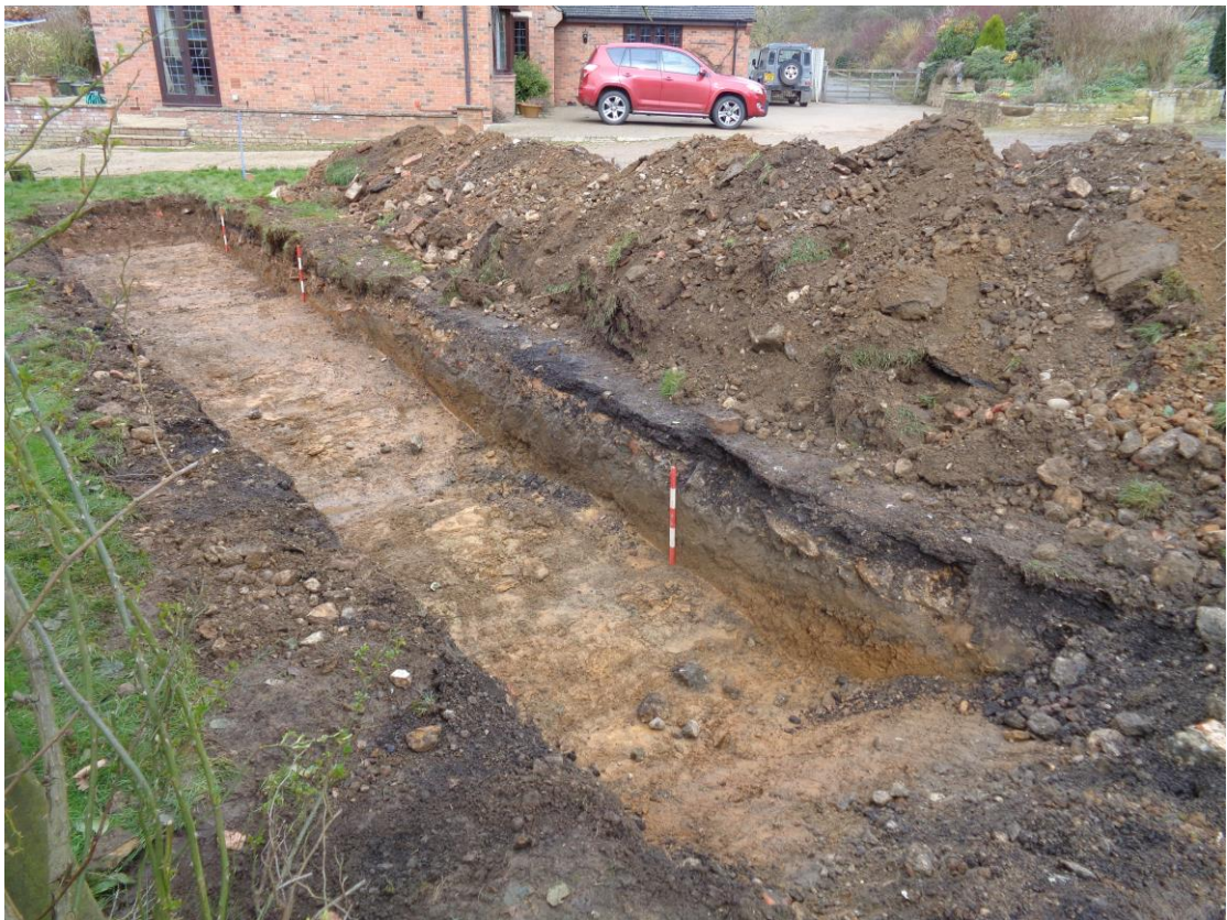
Plate 4; trench 3, view to the north
