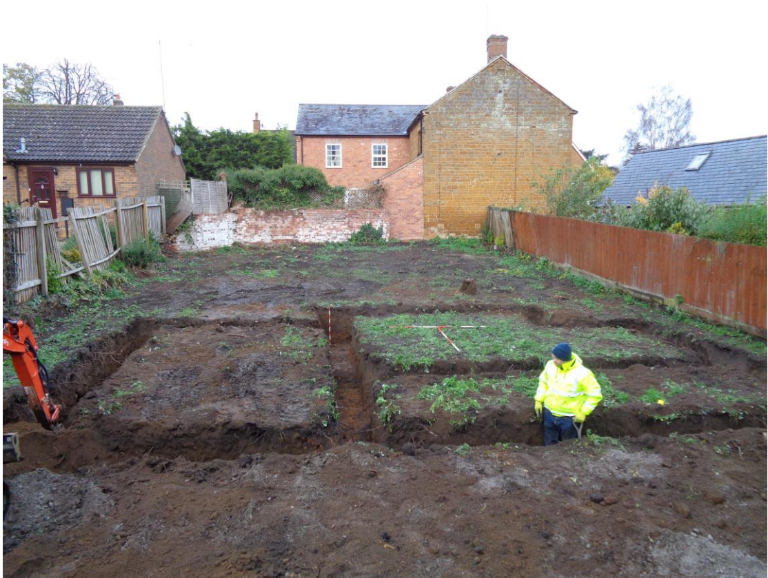
Plate 27; overall view to the north showing excavated foundation trench
