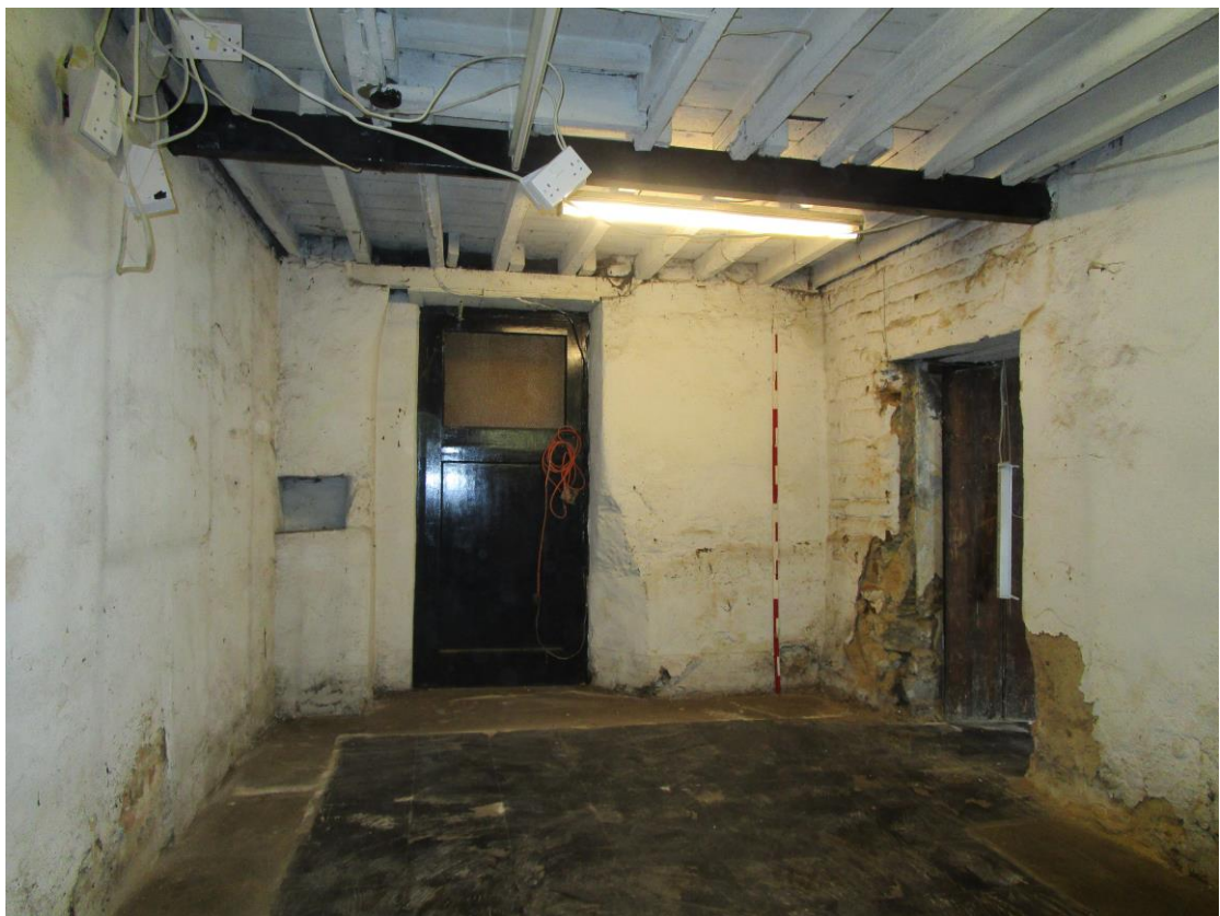
Plate 25; the old cart-shed interior from south, note niche at west corner
