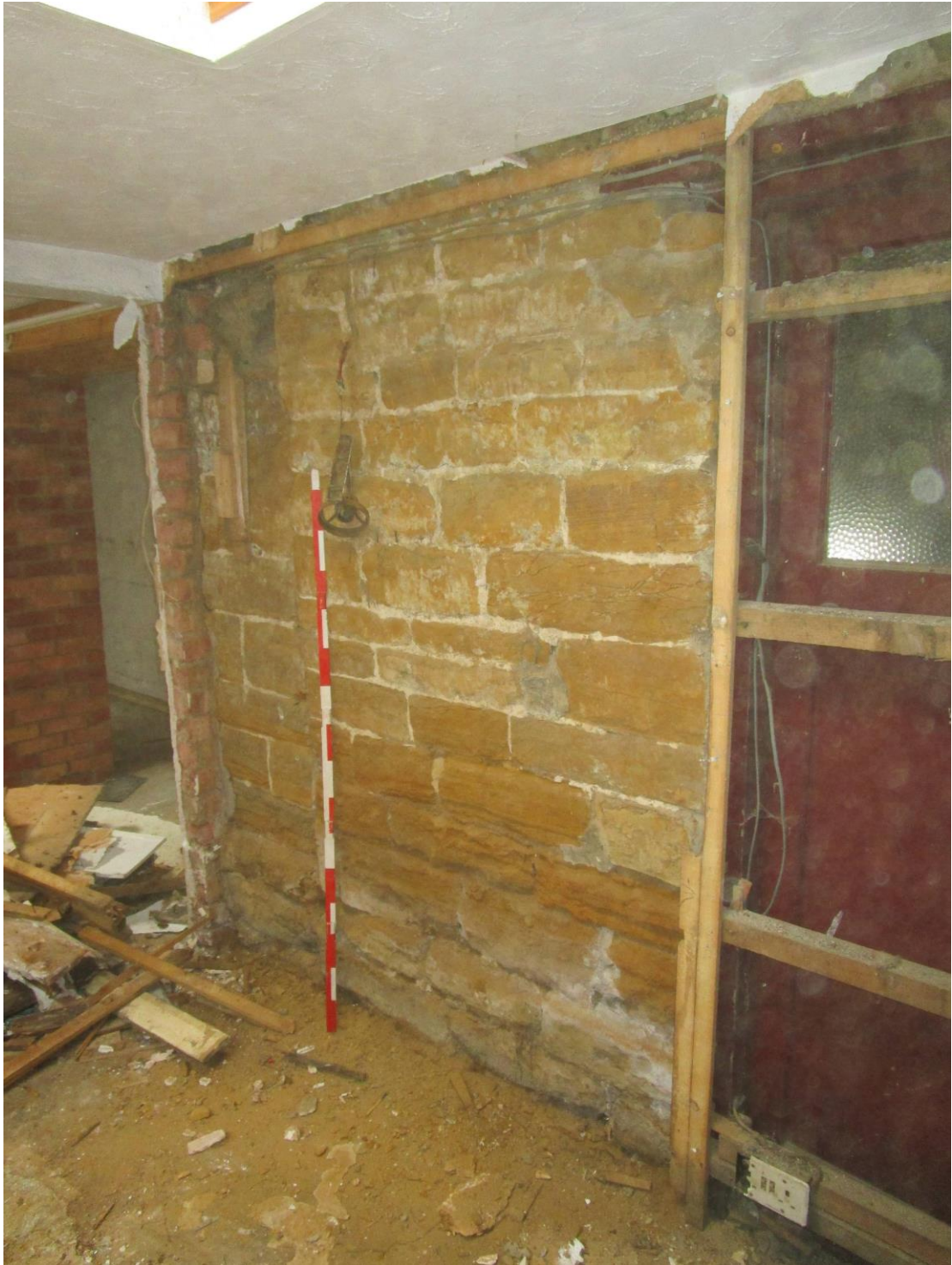
Plate 26; Blocked cart-shed doorway from north-west
