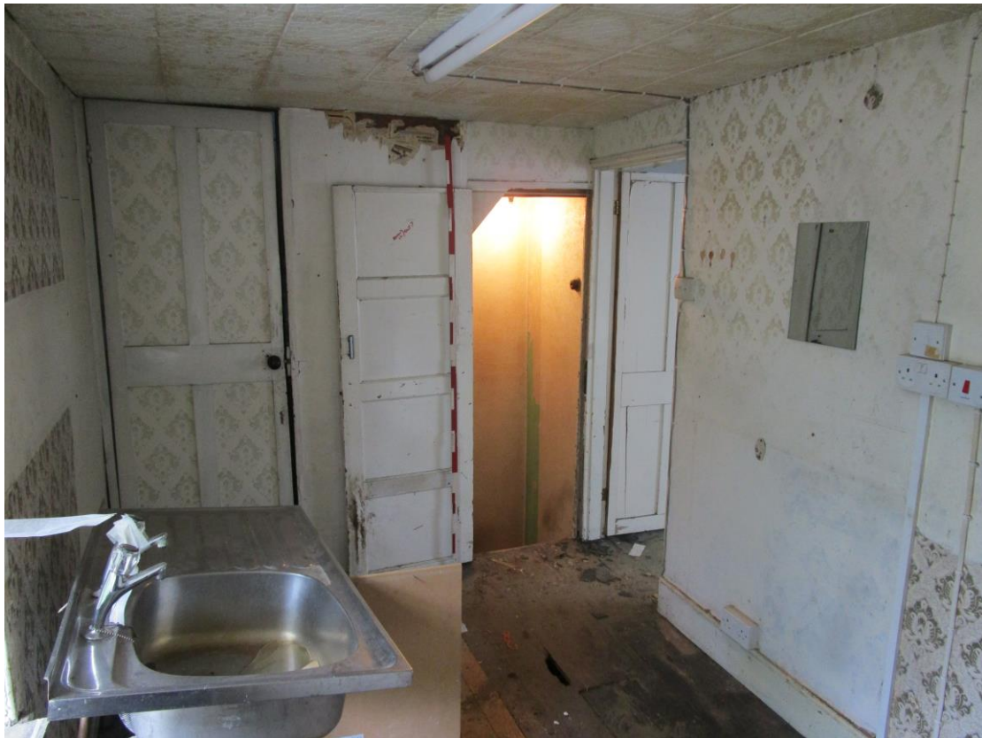
Plate 18; No.30, 1 st floor kitchen at rear
