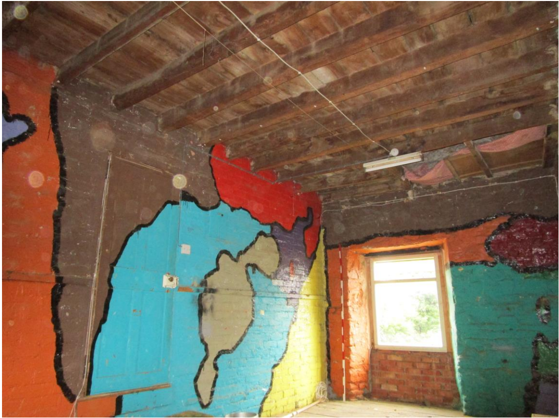
Plate 20; Room over old cart-shed, from south-east
