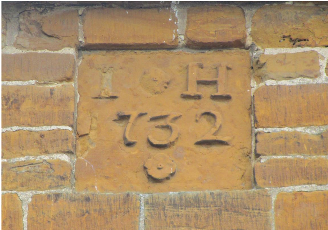
Plate 3; Date stone on the front of no. 30
