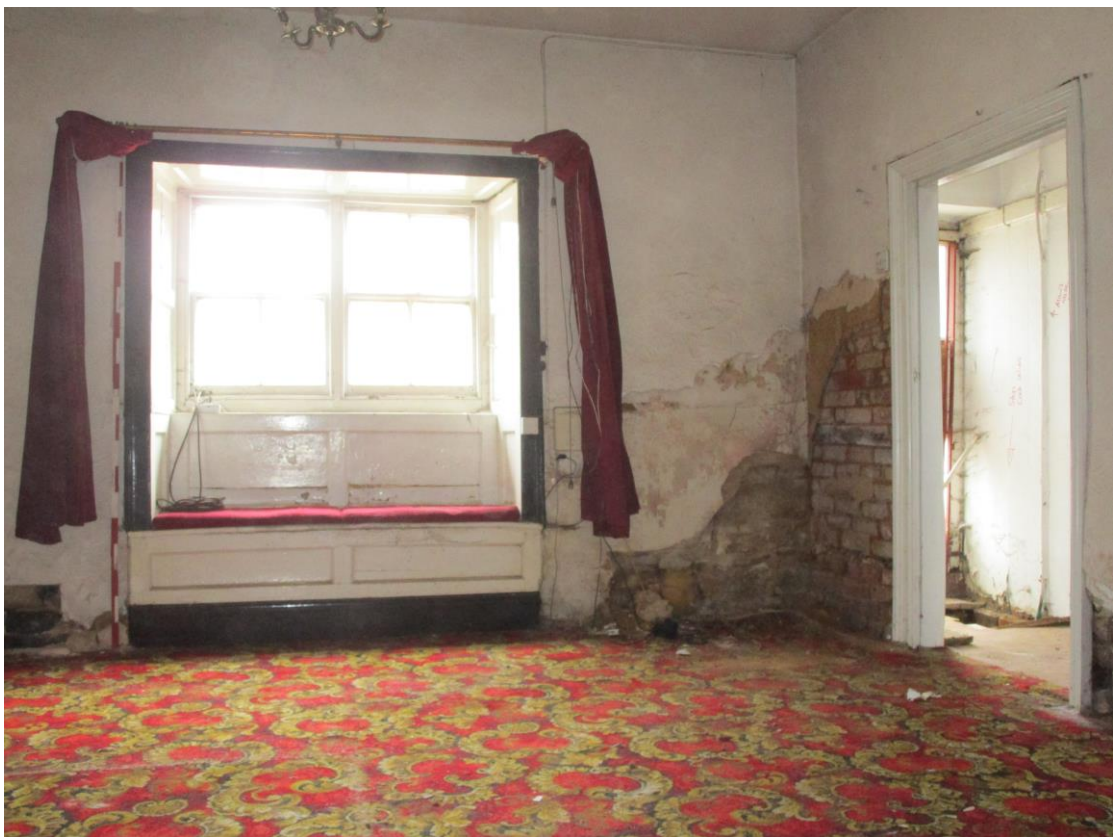
Plate 15; No.28, east room ground floor, 1688 embrasure, later window and seat
