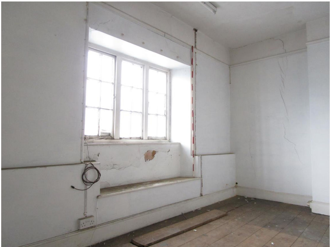
Plate 12; No.28, 1 st floor window to road
