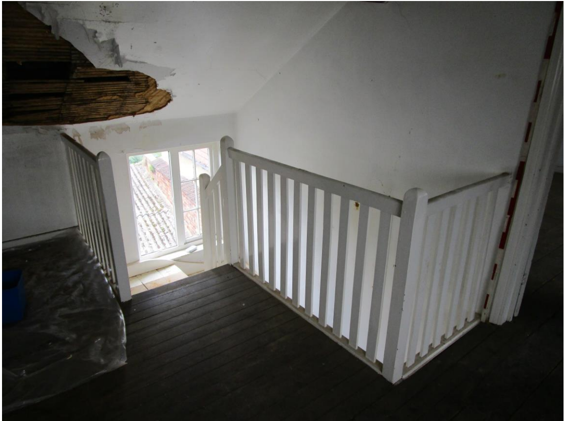
Plate 11; No.28, head of stair to attic
