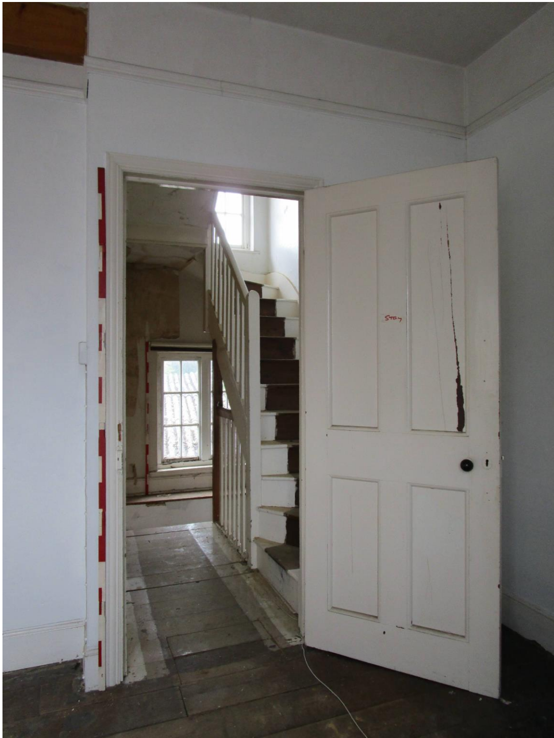
Plate 13; No.28, stair from 1 st floor to attic
