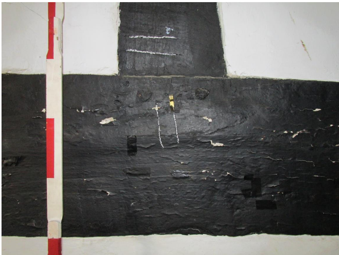
Plate 28; Carpenter's numbers on tie-beam and post of south wall
