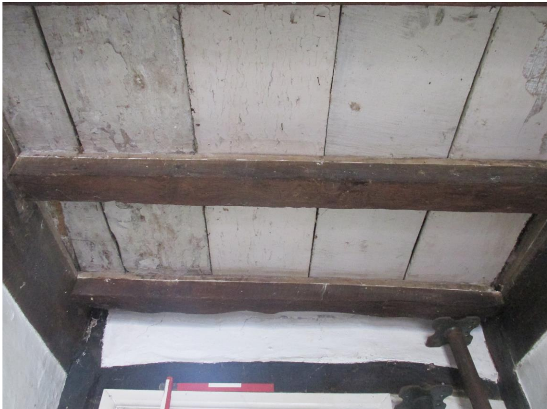
Plate 6; Detail of floor over rear of passage
