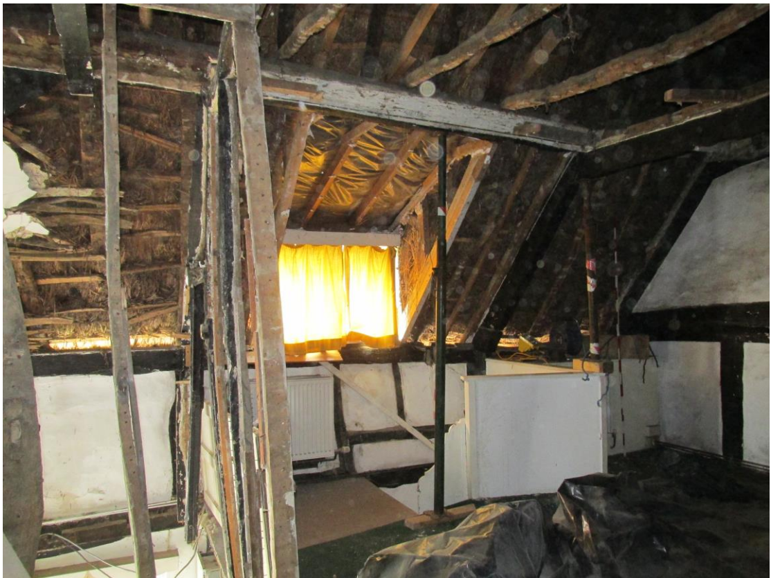
Plate 18; Upper storey interior from north-west
