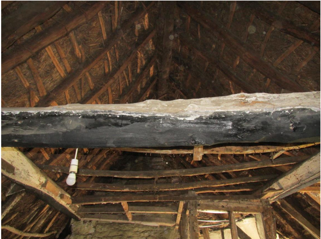
Plate 19; Roof interior over the north end
