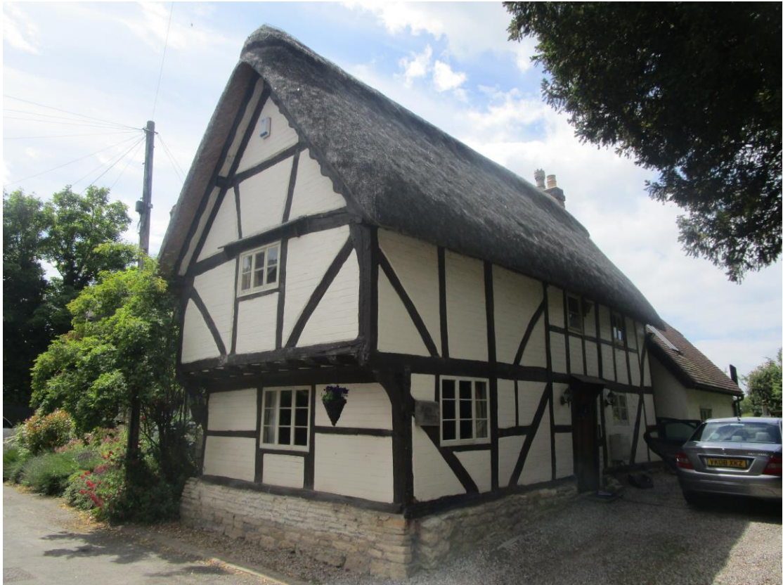
Plate 30; House, m. on Historic Environment plan, showing C15 jettied-framing and C16 fabric beyond
