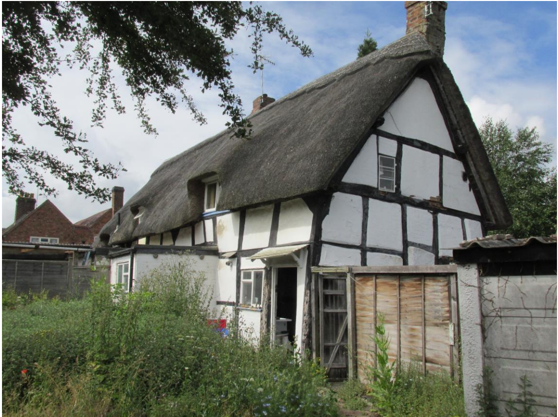
Plate 4; view from north-east
