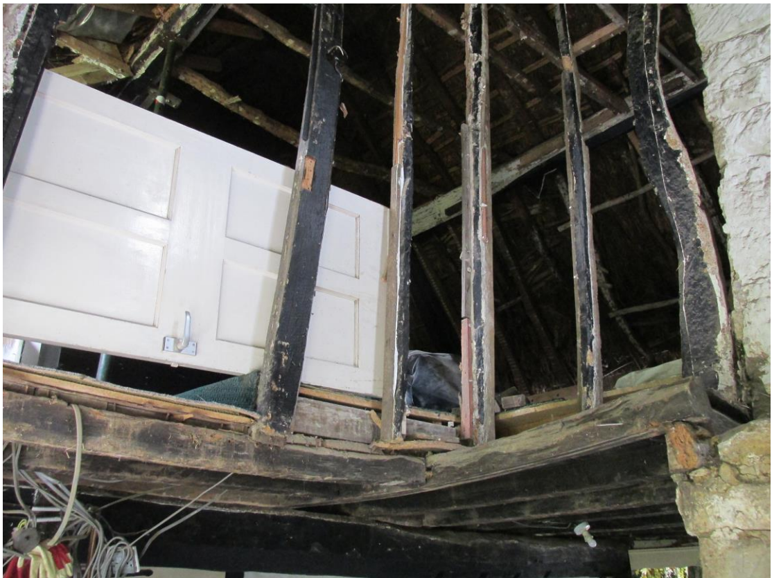
Plate 14; View of framing from the north-east corner of the dwelling
