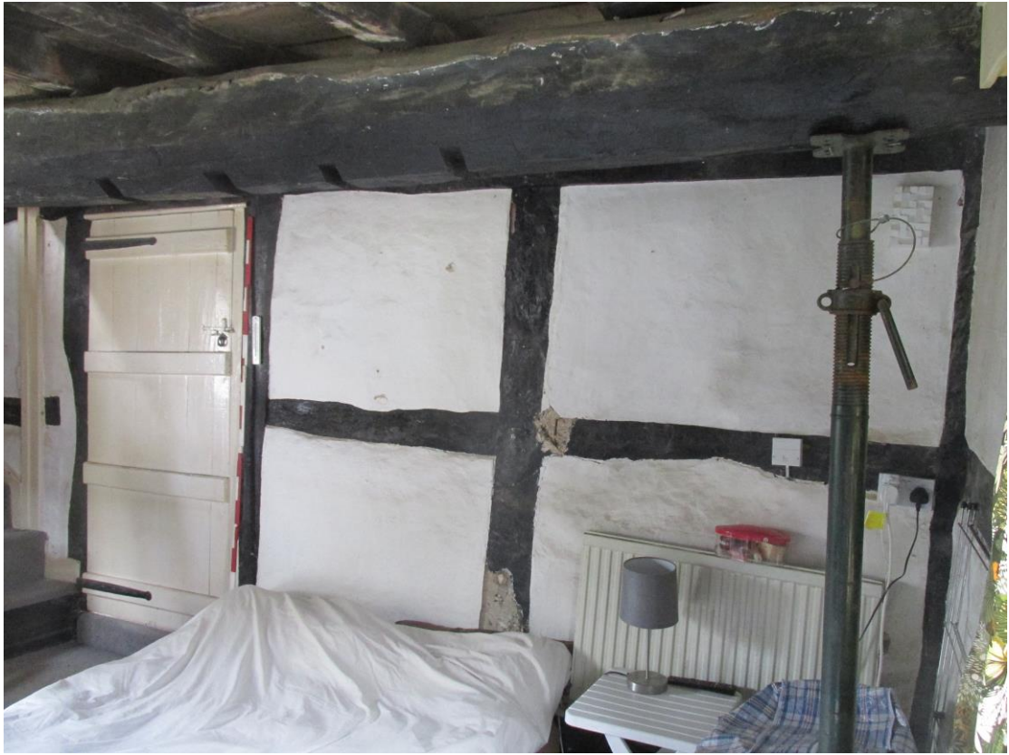
Plate 10; Ground floor room and passage-frame from north
