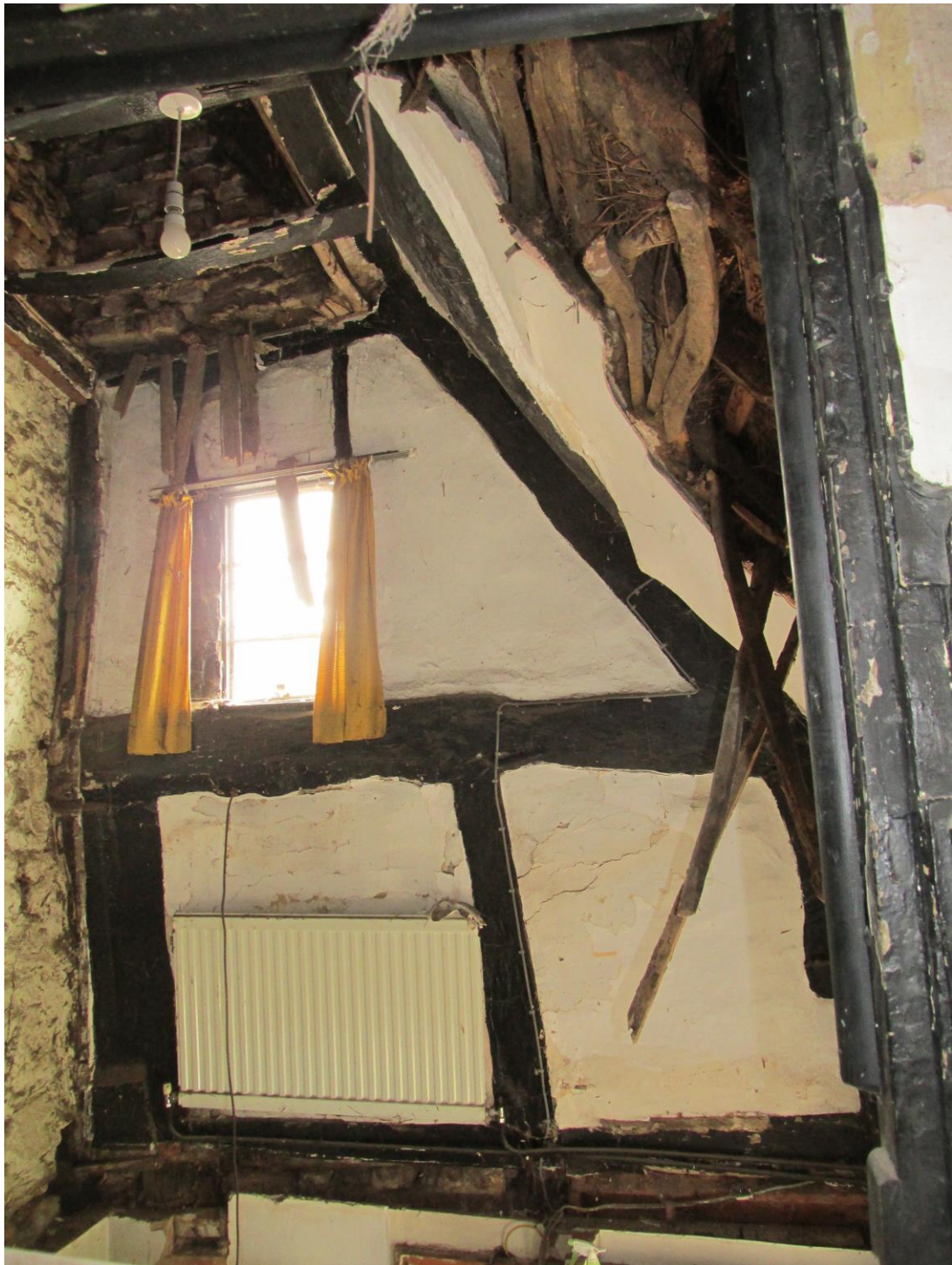
Plate 23; Interior of north wall to east of chimney
