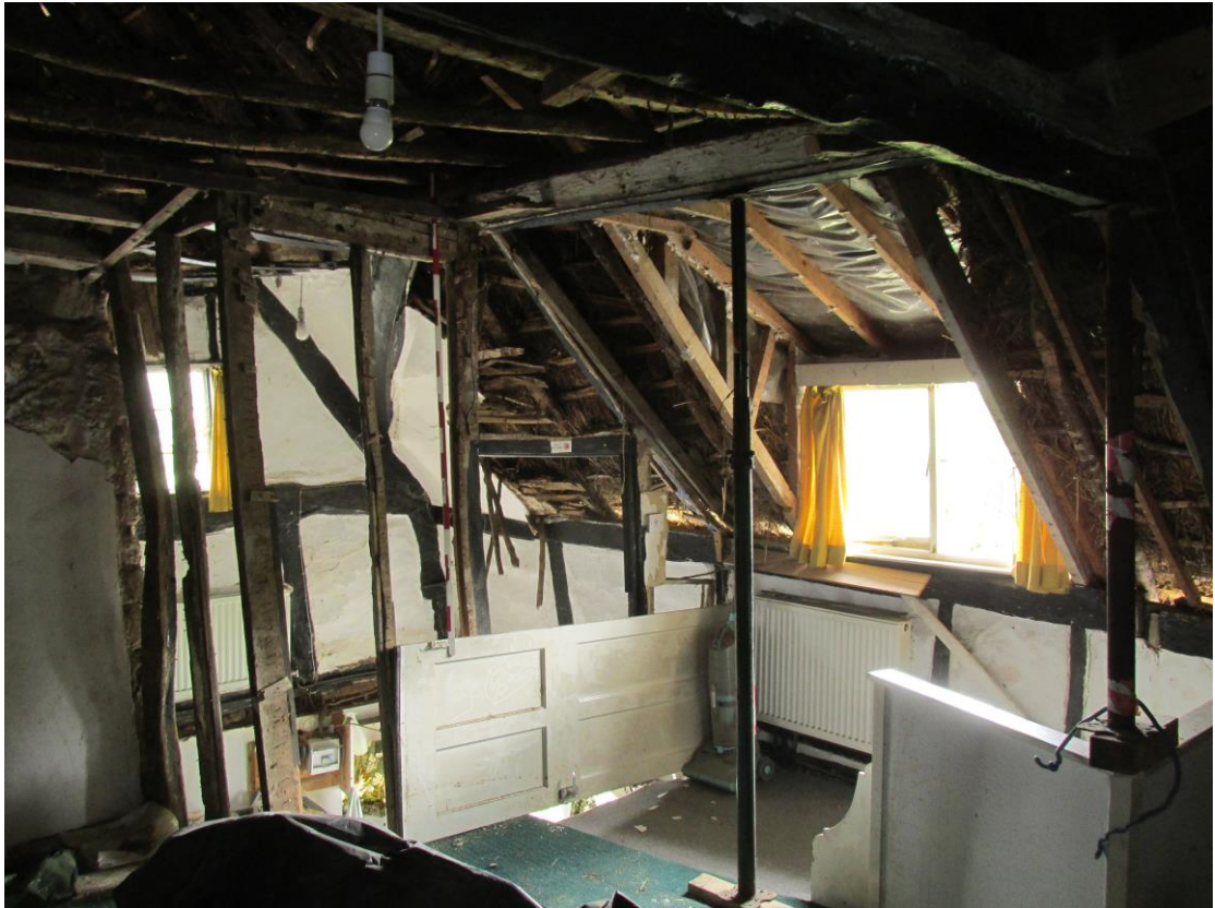
Plate 17; Upper storey interior from south-west
