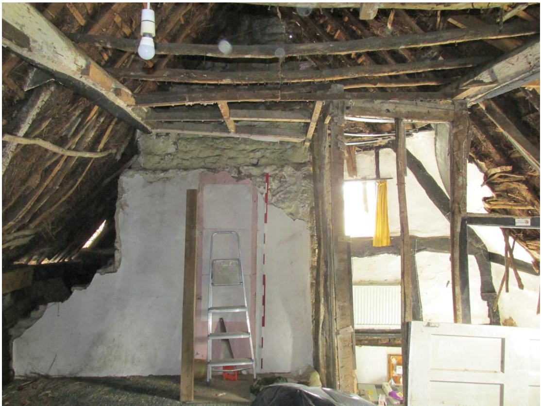
Plate 20; North end of the upper storey
