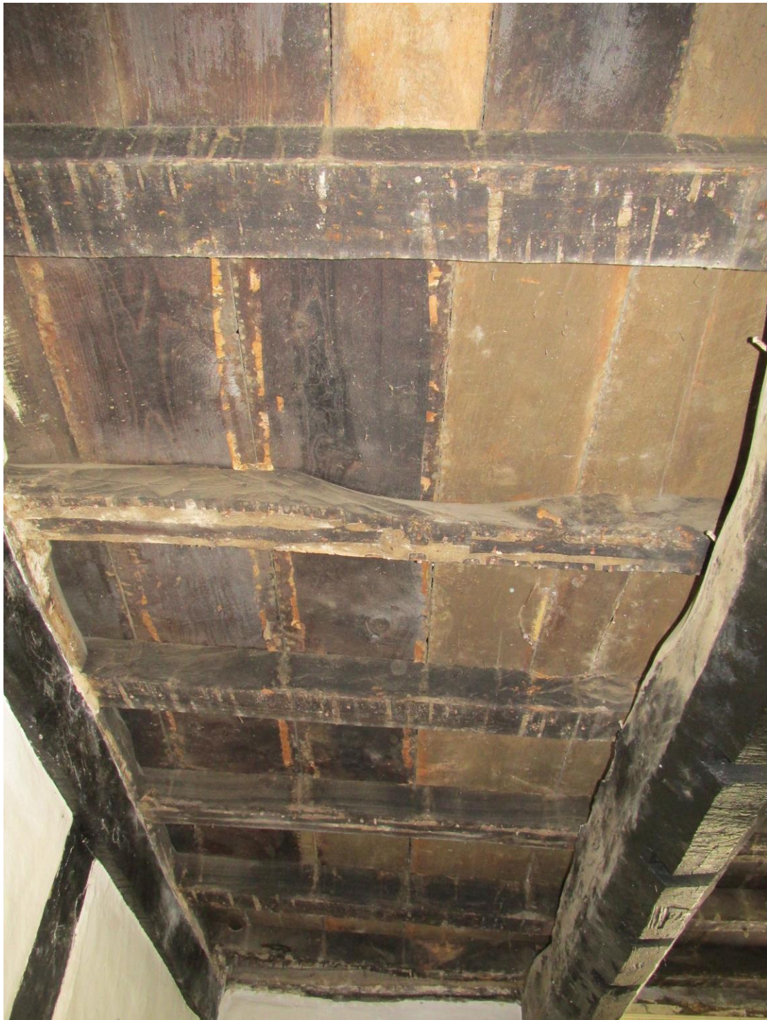
Plate 12; Floor over ground floor room adjacent to passage from east
