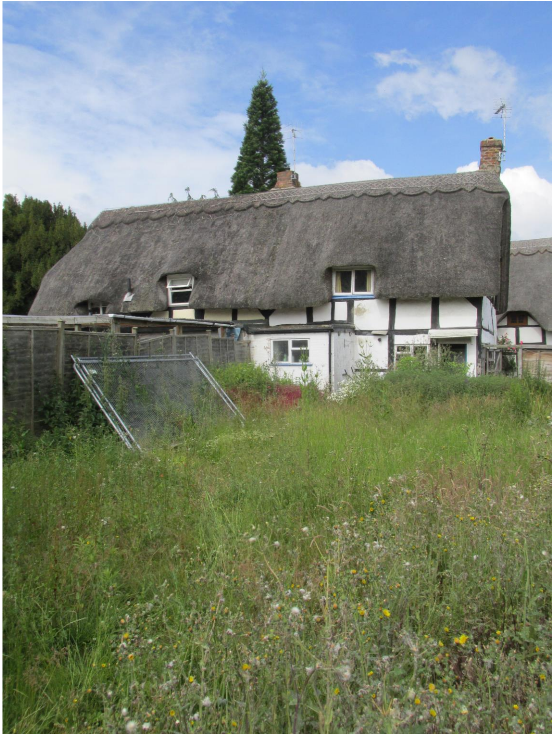
Plate 3; view from east
