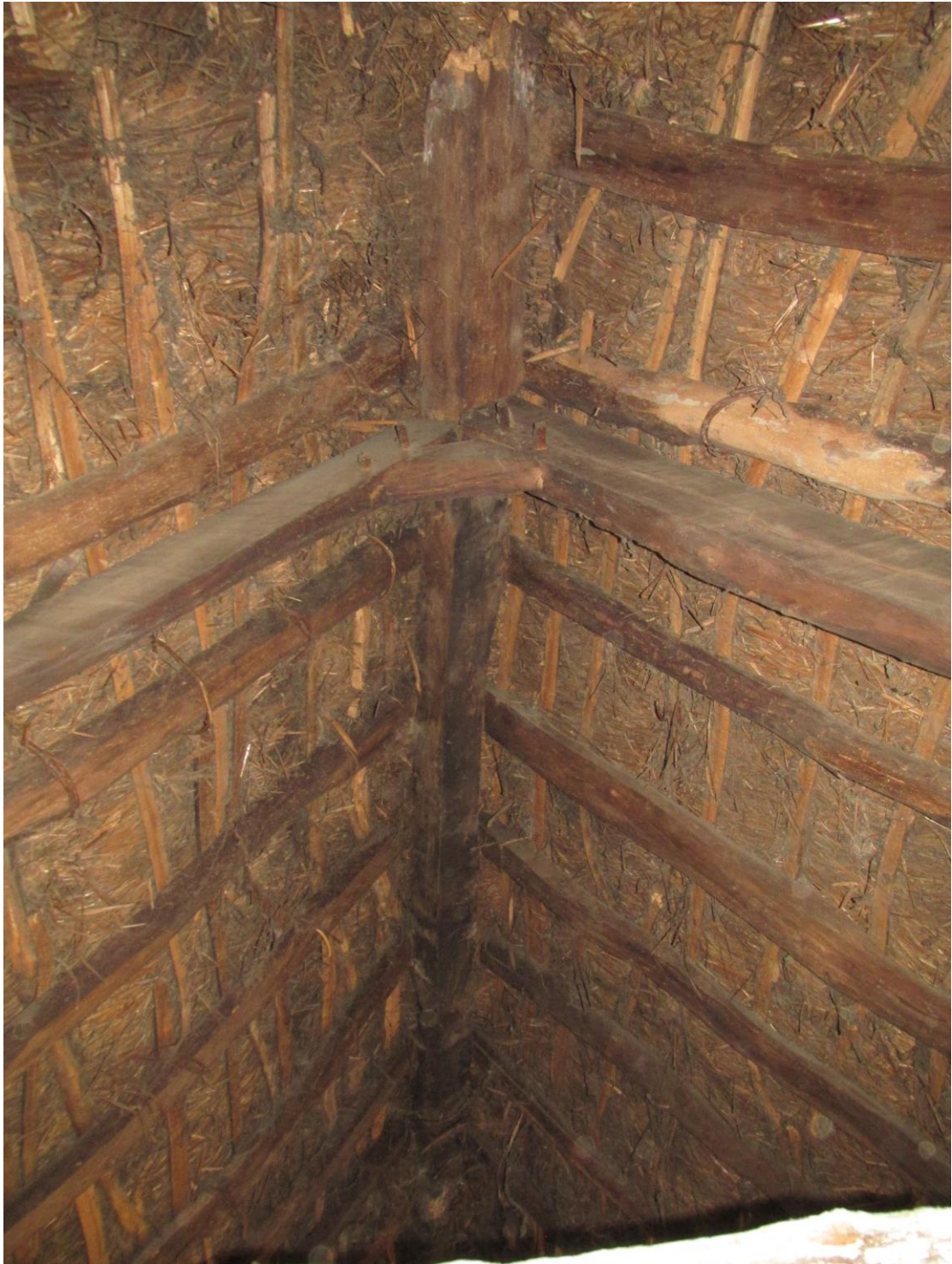
Plate 25; Roof interior from south
