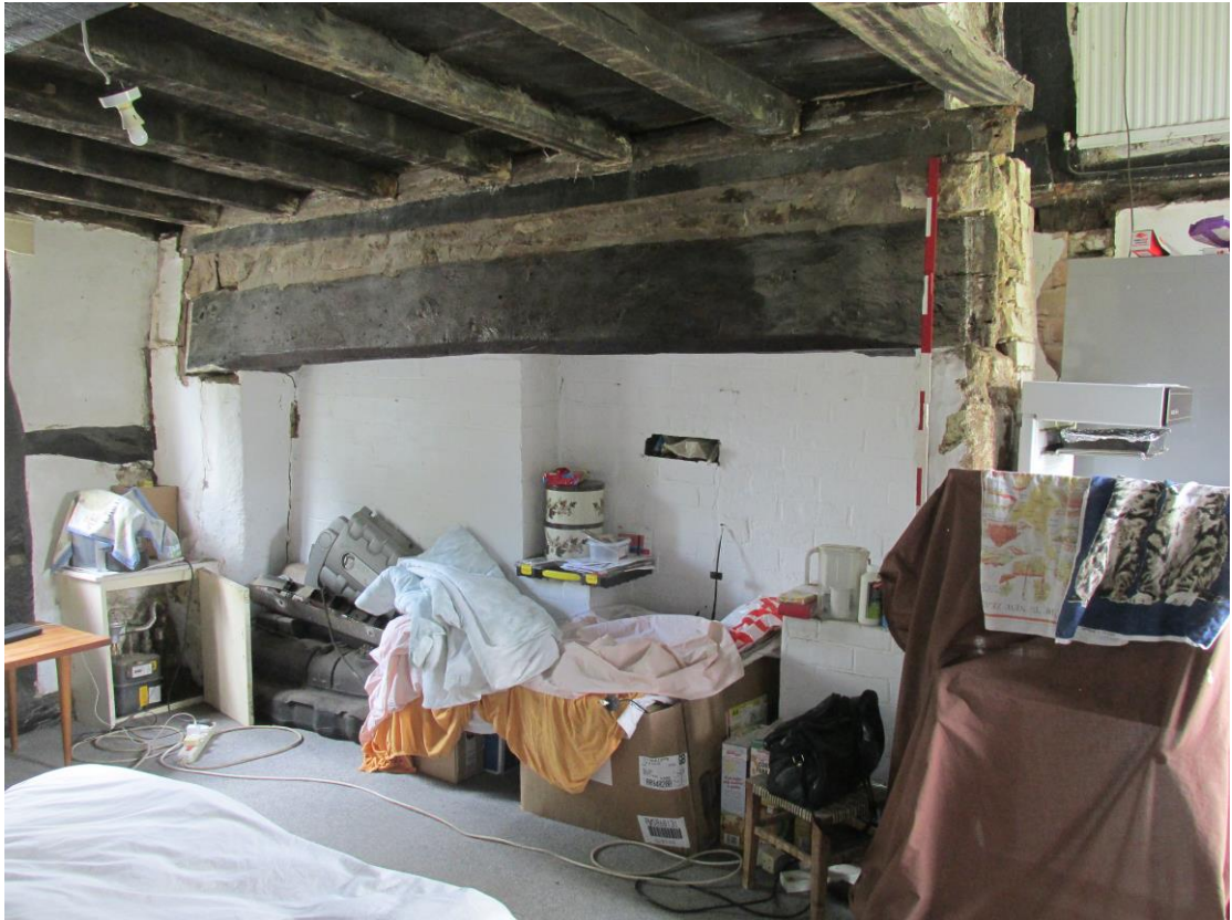
Plate 13; View of fire-place from south-east showing inserted brick range
