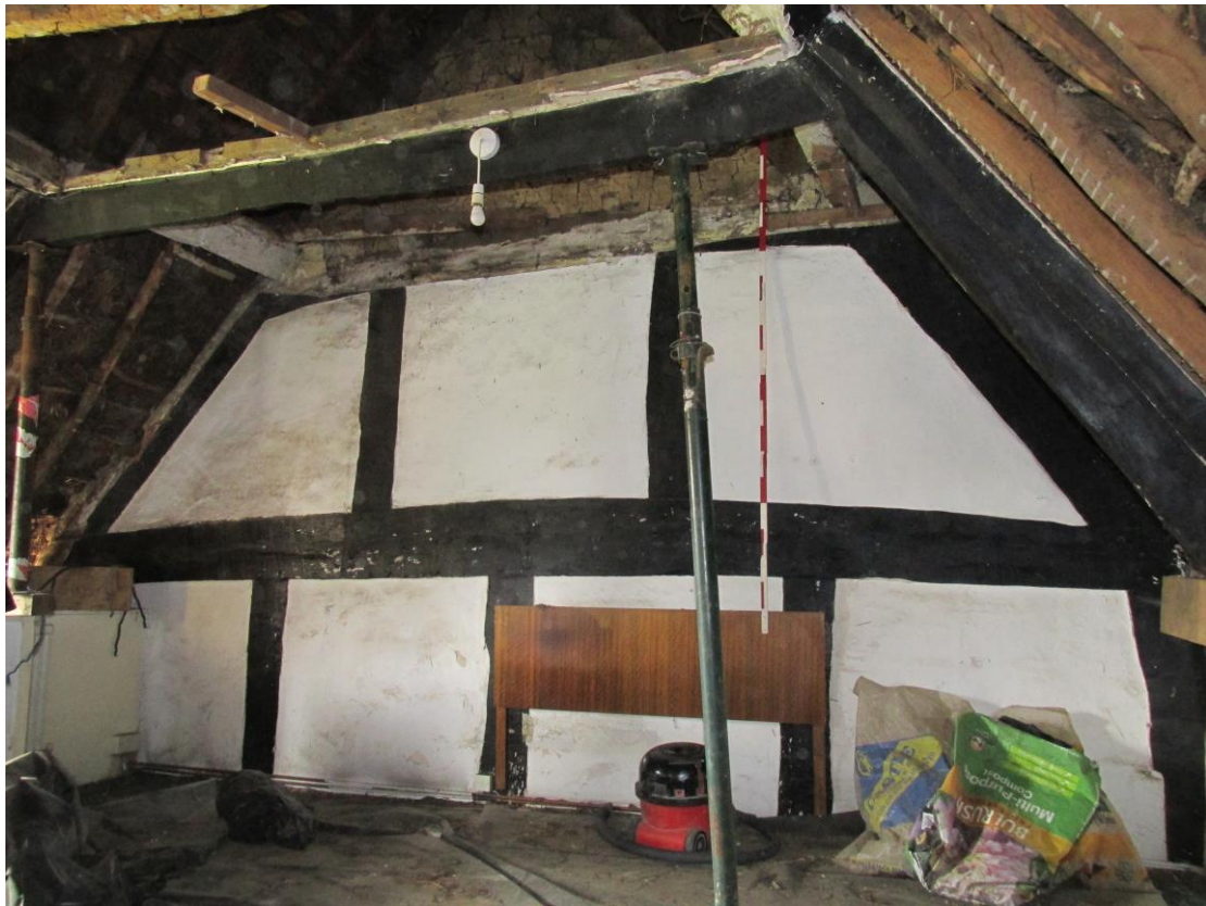
Plate 27; South wall on upper floor from north
