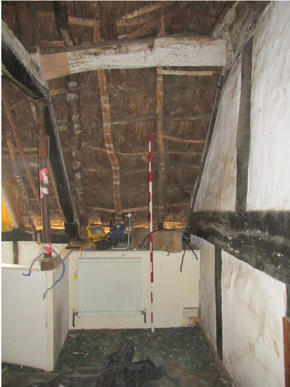
Plate 26; Upper storey over passage from west showing 'stump' of lost tie-beam
