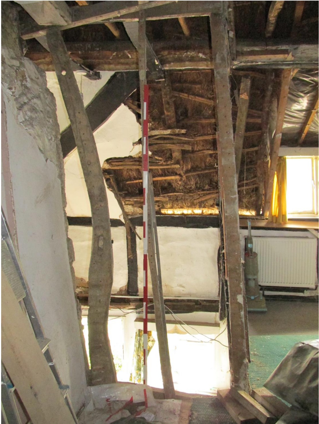
Plate 22; Re-used cart-timbers in 1 st floor partition from west
