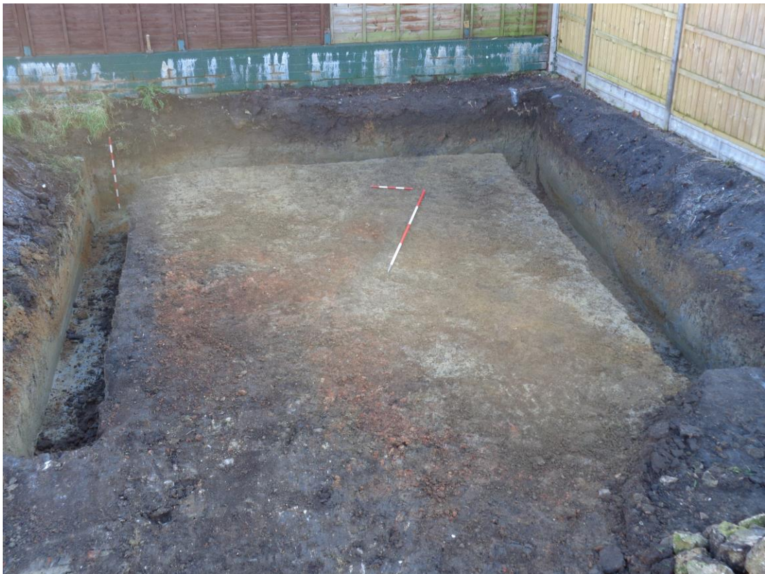
Plate 32; trench 2, foundation trench for proposed garage, from the south-east
