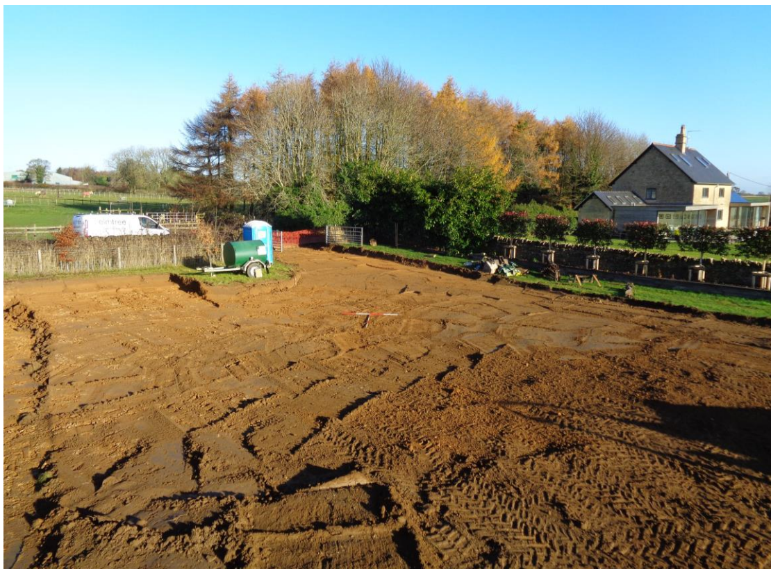
Plate 2; eastern half of the excavation showing the surface of the natural substrate, view north-east
