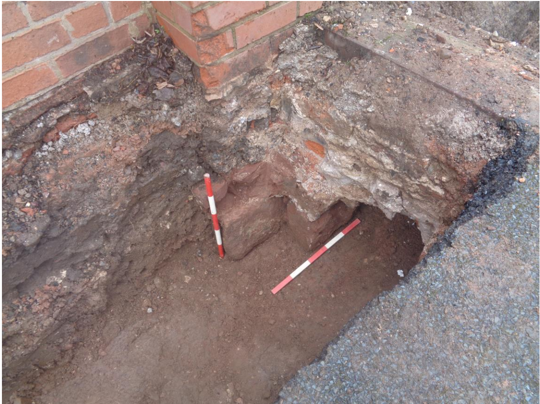
Plate 21; wall 703, view to the south-west (section 7d)
