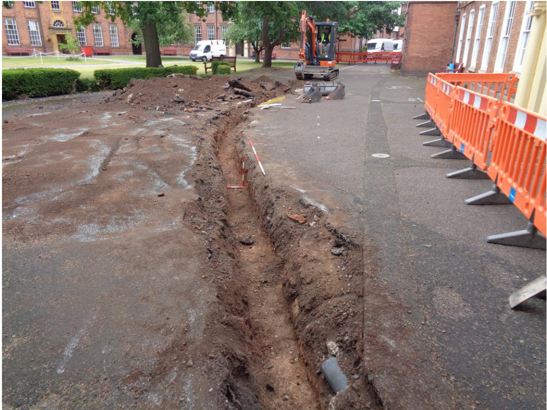
Plate 1; Trench 1 from west
