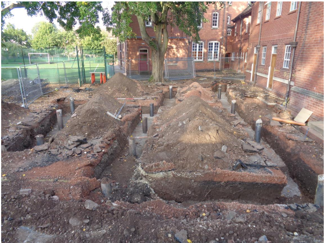
Plate 3; view of excavations from east
