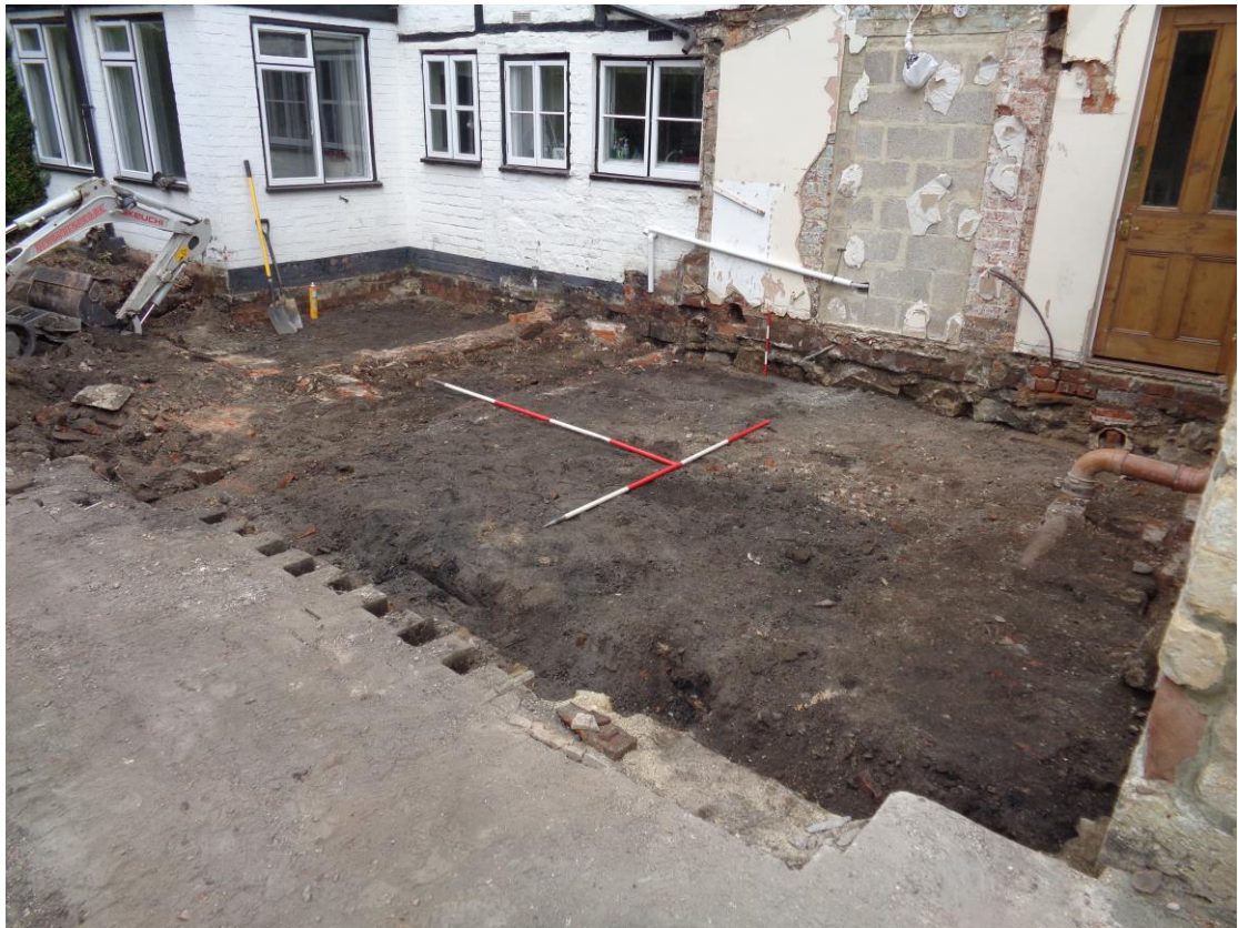
Plate 3; overall view of excavation from south
