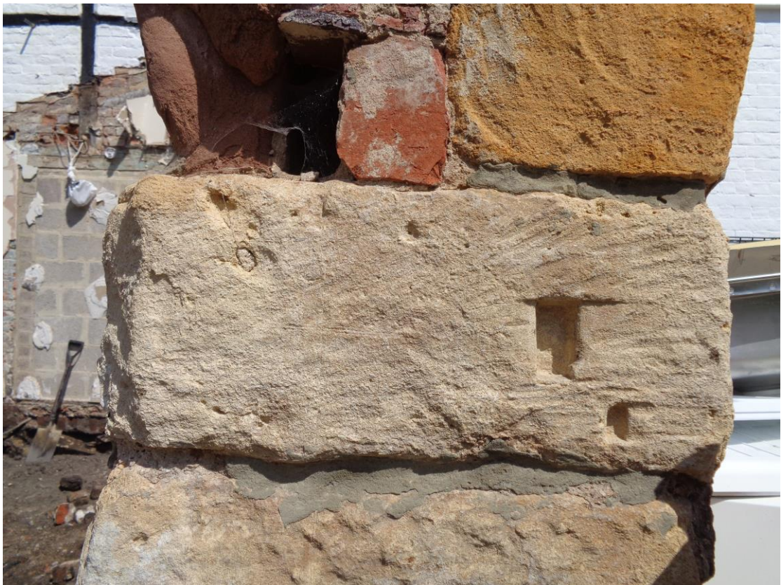
Plate 8; detail of door jamb (south-west end of wall 103)
