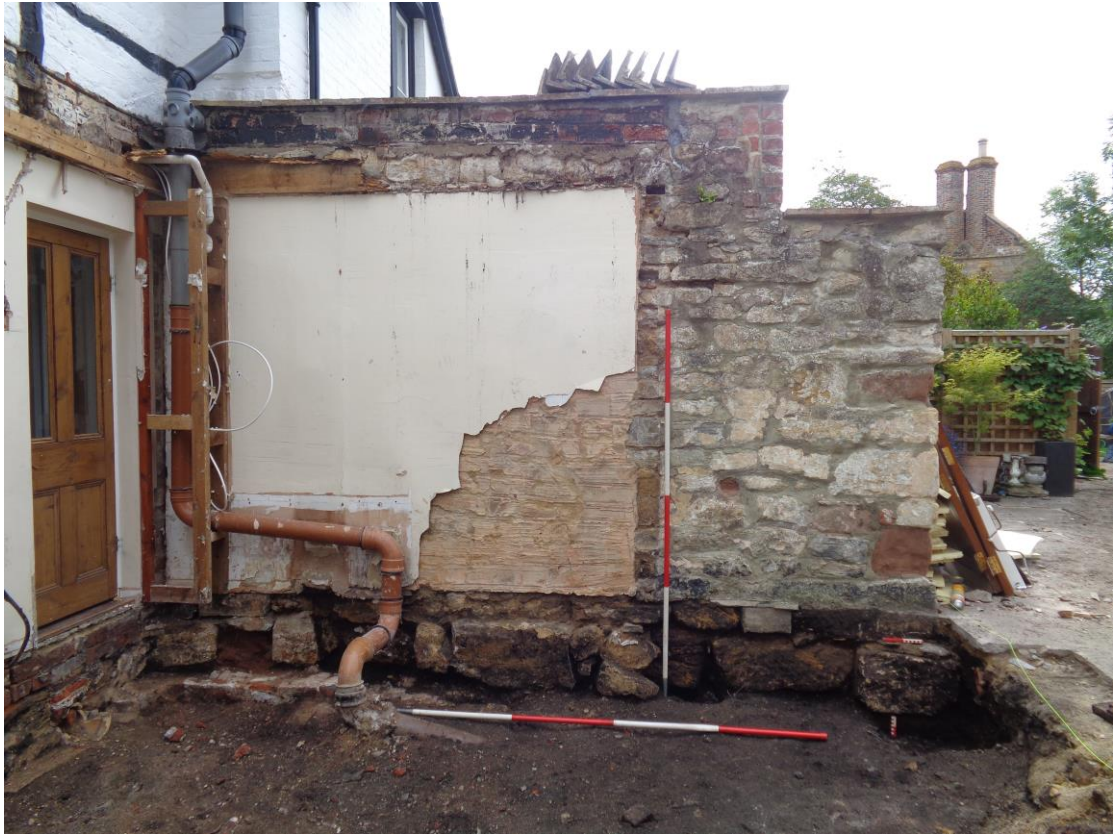
Plate 5; walls 103 & 104, north-west elevation
