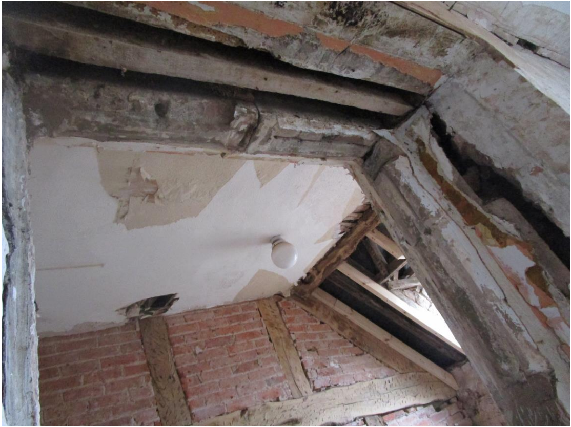
Plate 36; West-wing; detail of original first floor window
