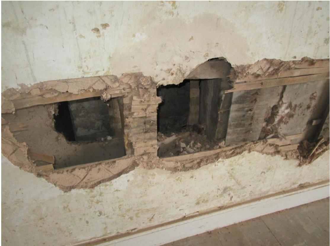
Plate 40; Cross-wing; first floor west wall detail of buried timber-frame
