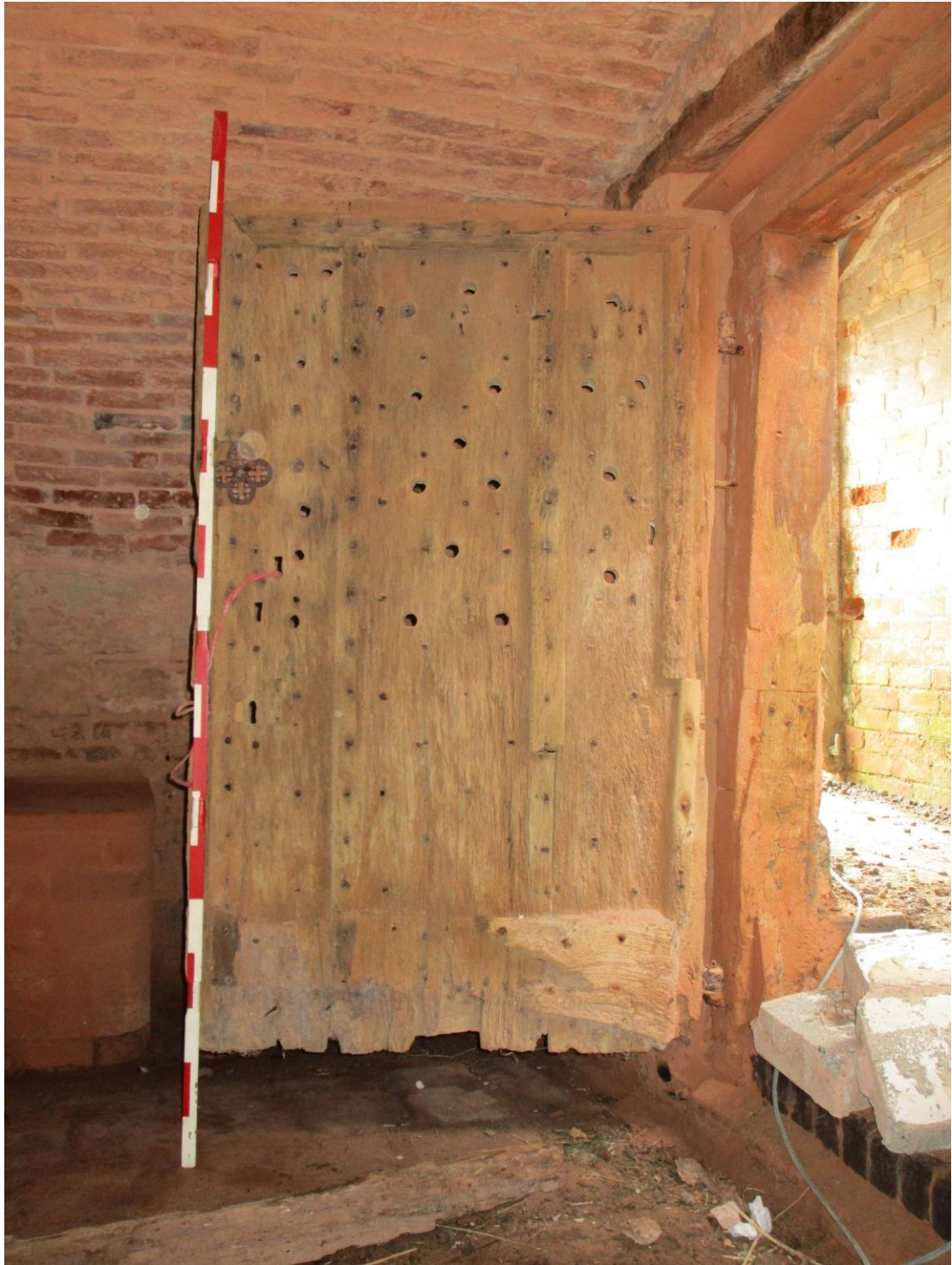
Plate 29; South-west wing; detail of re-used door in vaulted-cellar
