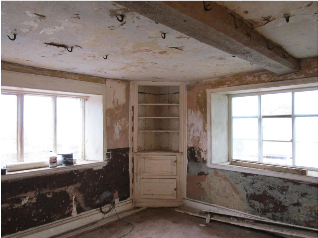
Plate 13; West-wing; ground floor corner cupboard
