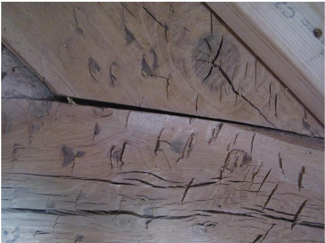
Plate 37; South-west wing; detail of carpenters' numbers on tie-beam (VIII)
