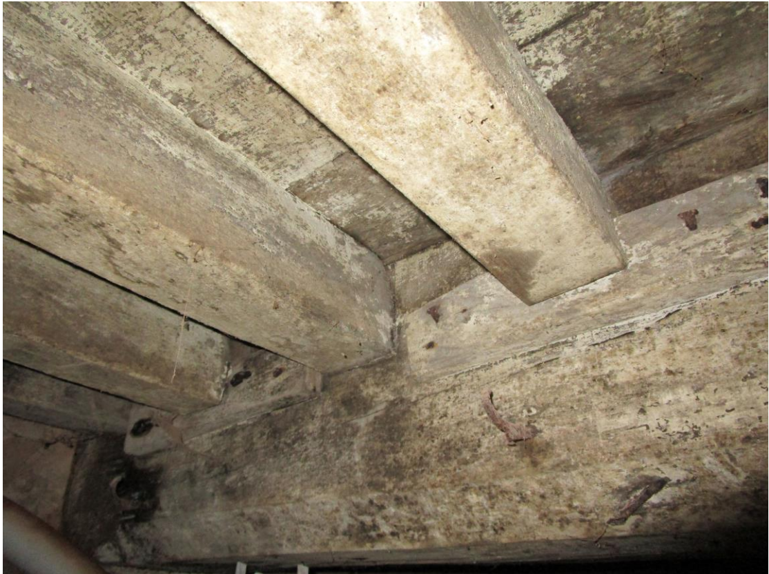
Plate 26; West-wing cellar; detail of floor over, with additional joists
