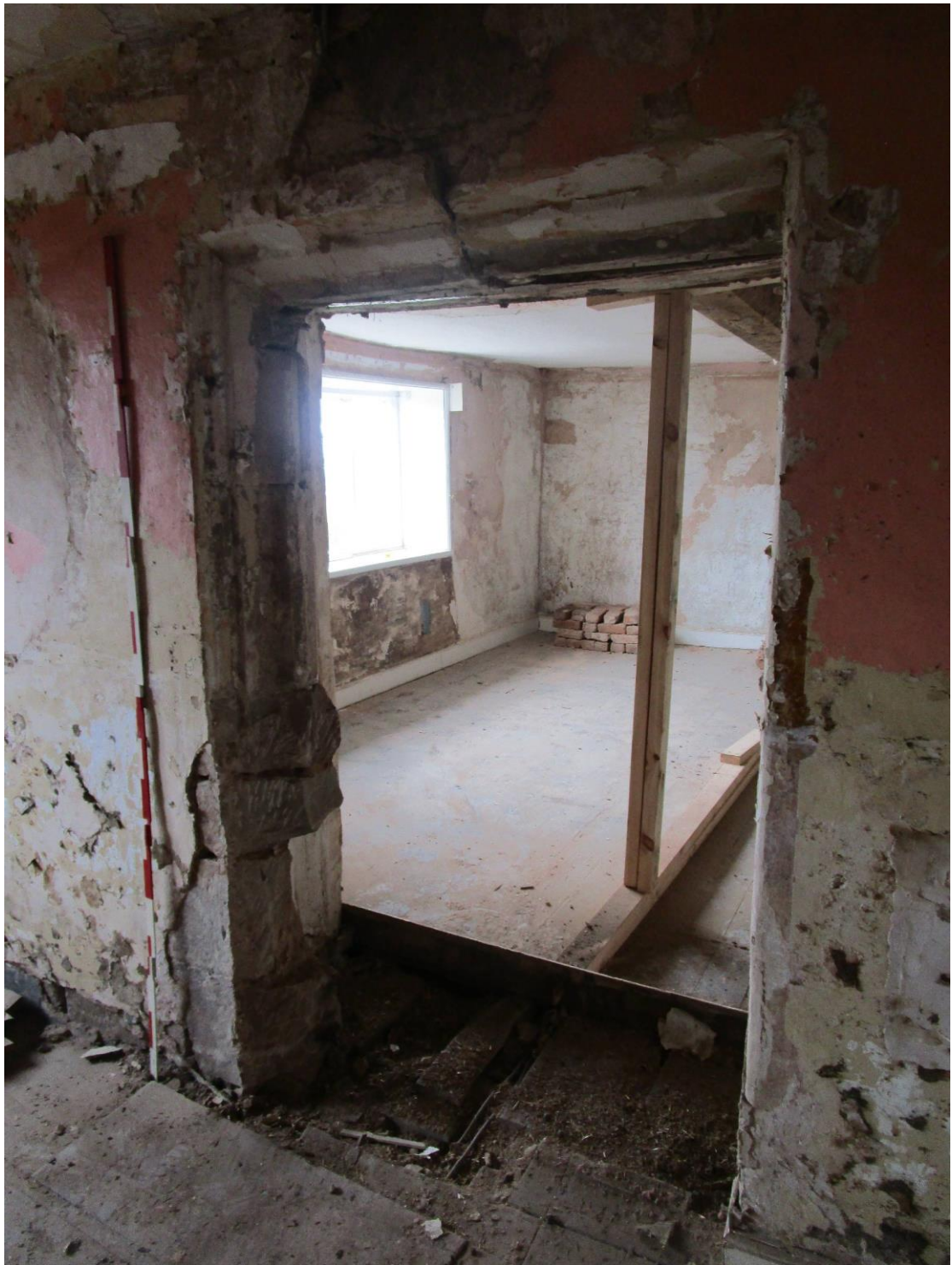
Plate 35; West-wing; remains of original first floor window in south wall
