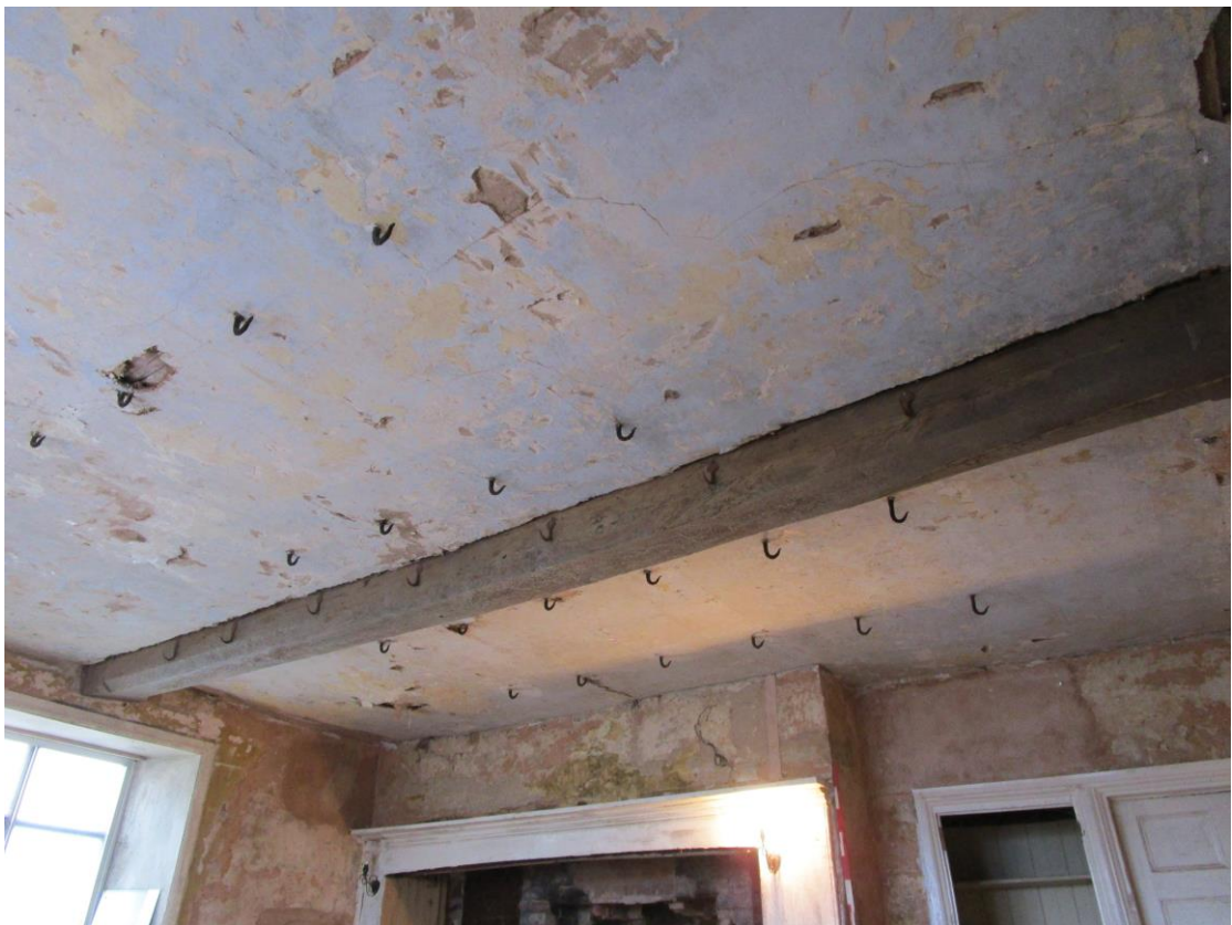
Plate12; West-wing; detail of ground floor ceiling
