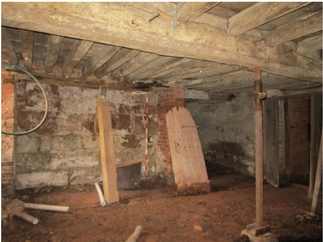
Plate 25; West-wing cellar; view to south-east
