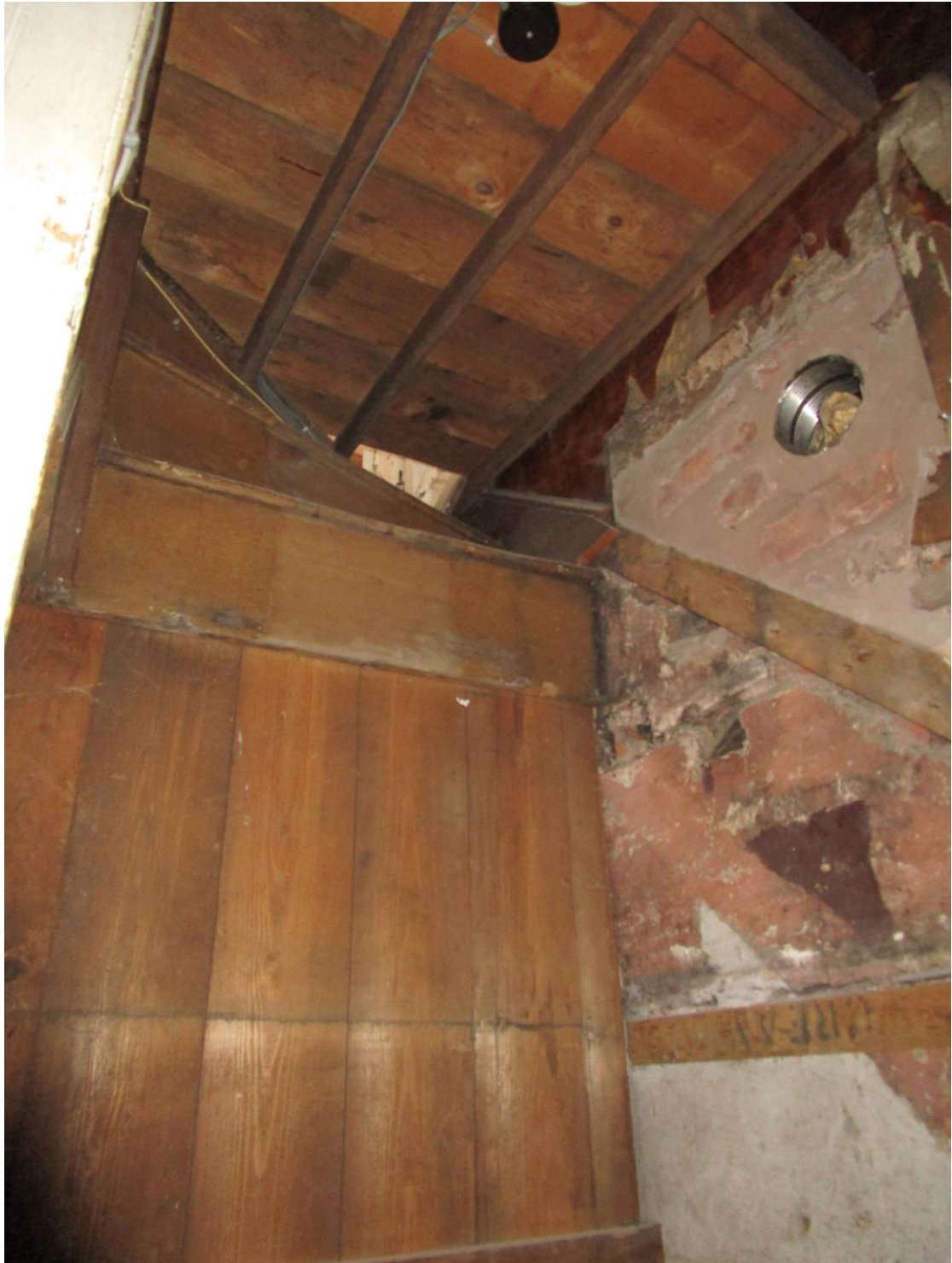
Plate 23; Remains of former ground floor winding-stair south of quadruple-stack
