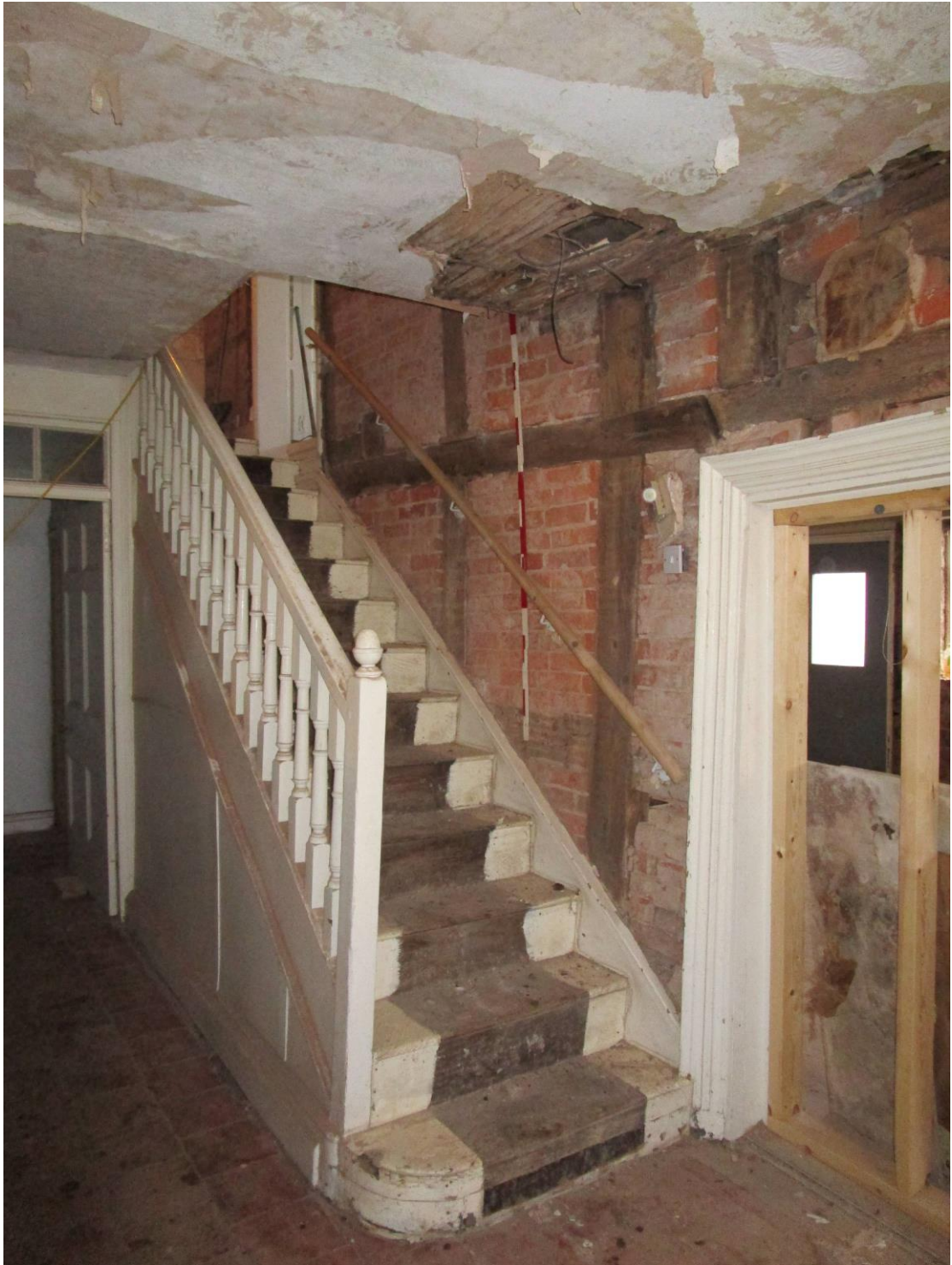
Plate 17; South-west wing; ground floor staircase
