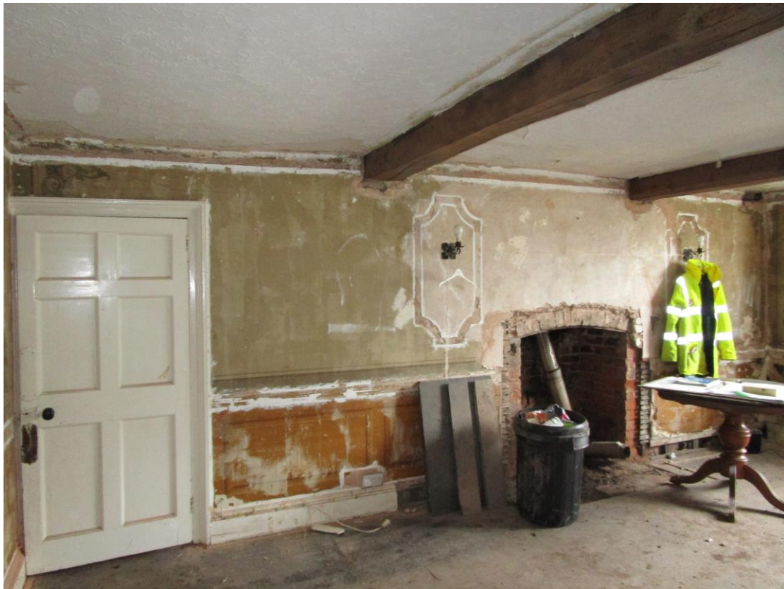
Plate 20; Cross-wing; ground floor interior from north-west
