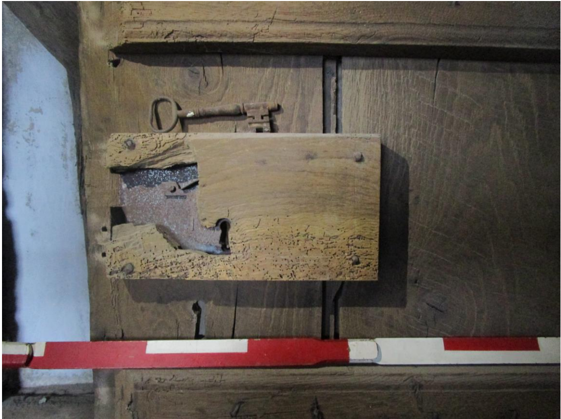
Plate 44; West-wing; detail of lock on re-used door in garret
