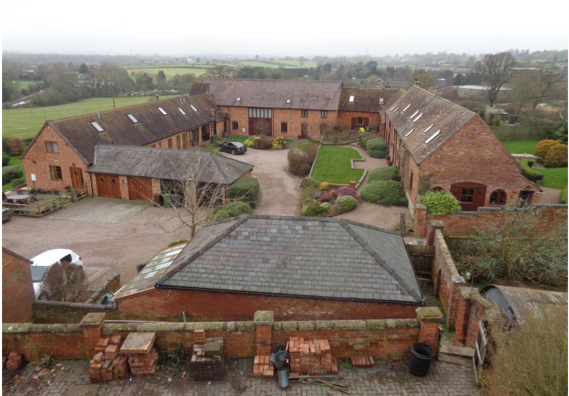
Plate 8; View of farm-yard from the farmhouse
