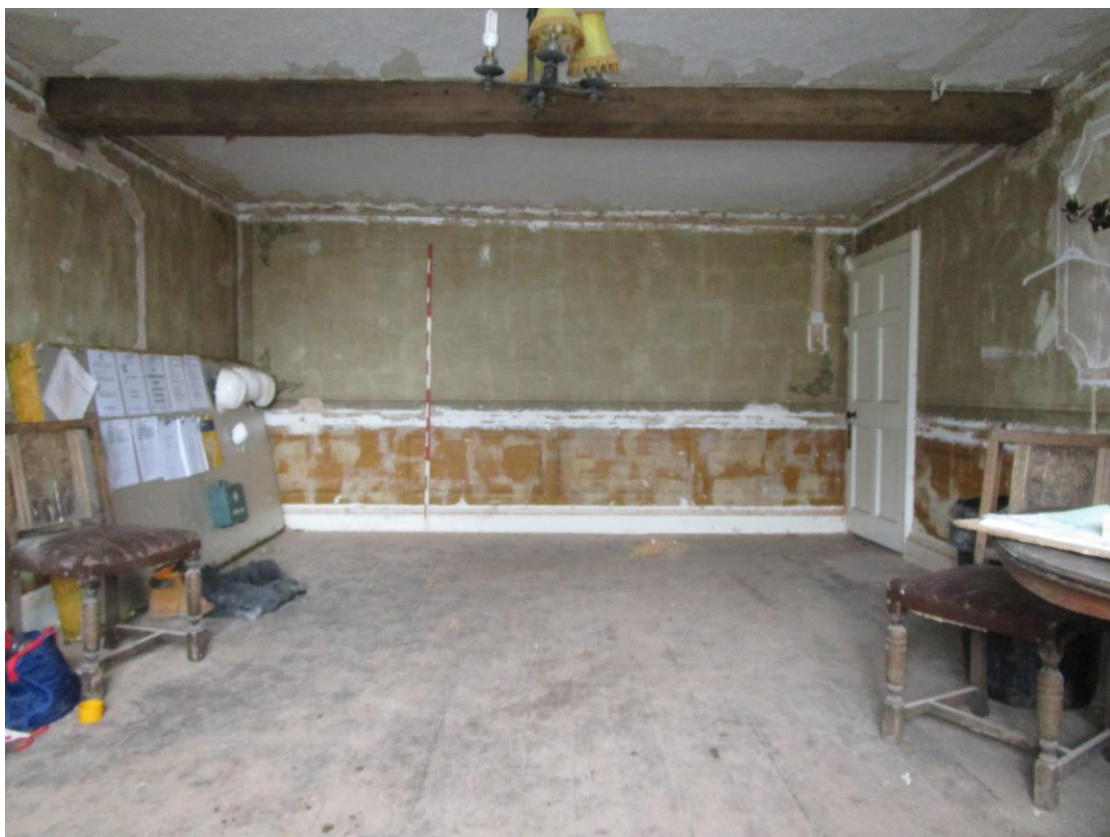
Plate 21; Cross-wing; ground floor interior to south
