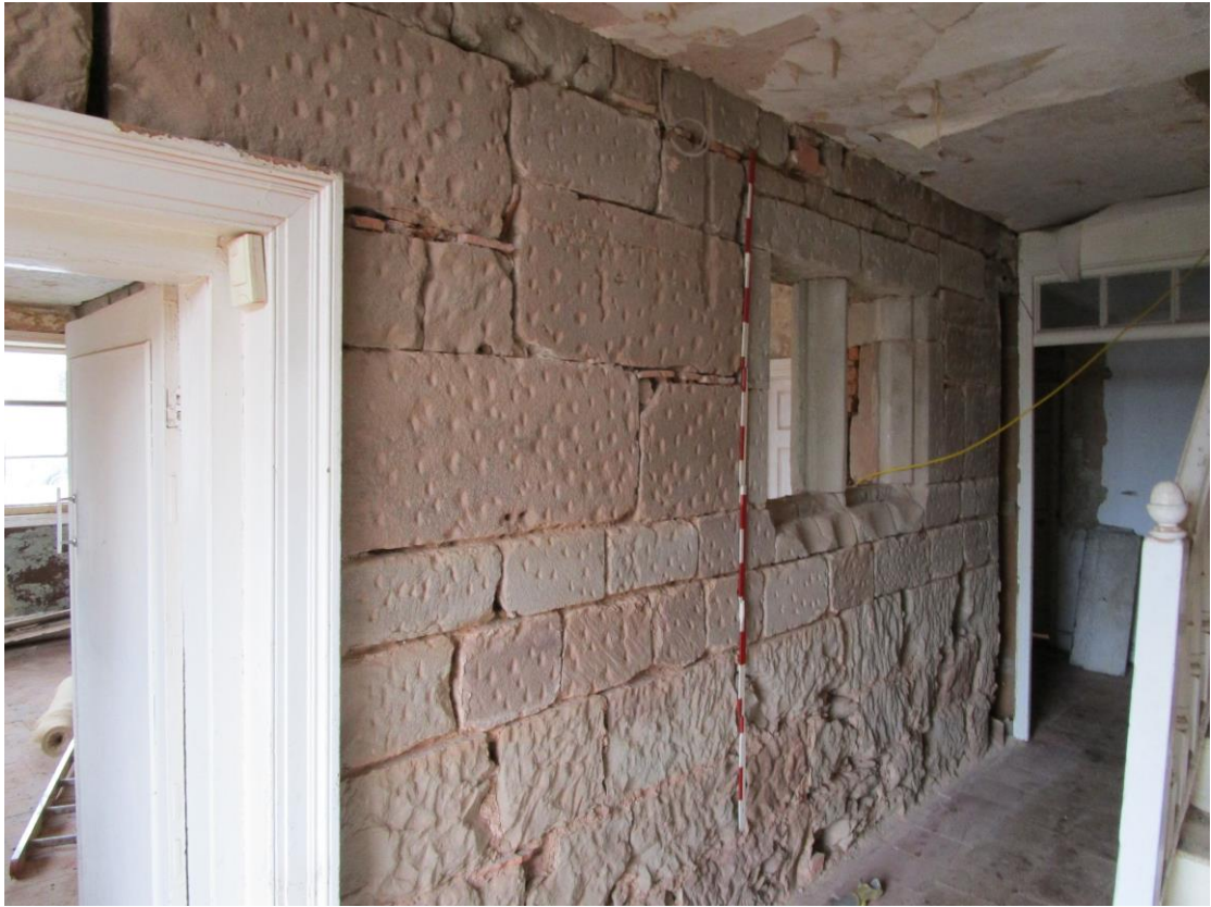
Plate 15; West-wing; south wall exterior ground floor
