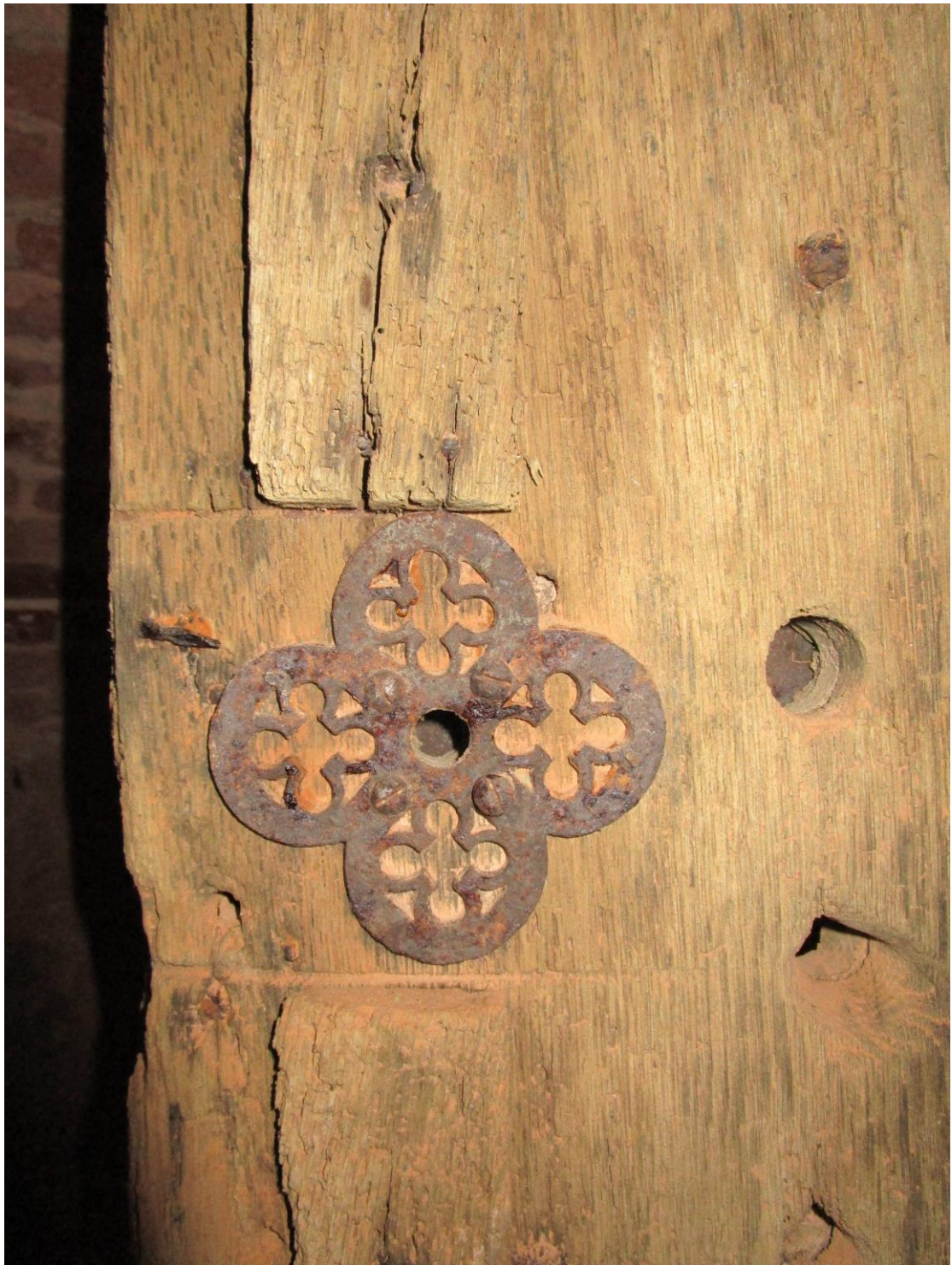
Plate 30; South-west wing vaulted-cellar; detail of iron-plate on re-used door
