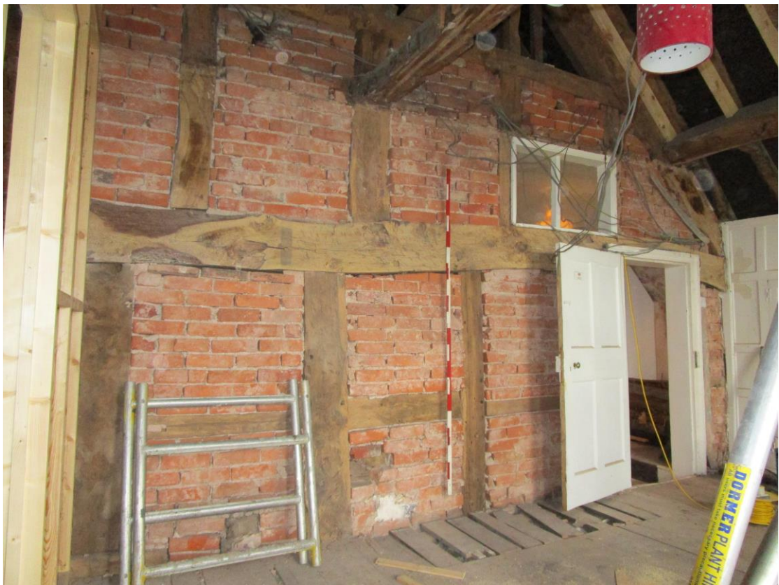
Plate 39; South-west wing; view of first floor interior from south-west
