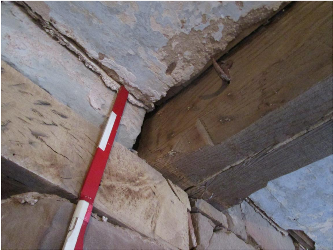
Plate11; West-wing detail of scroll-stop on chamfer
