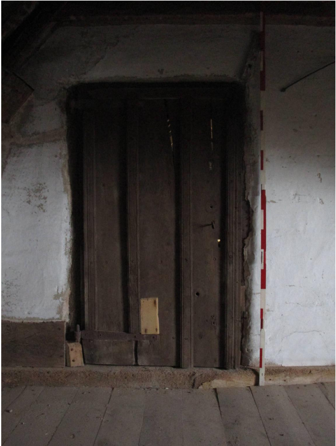
Plate 43; West-wing; re-used door in garret
