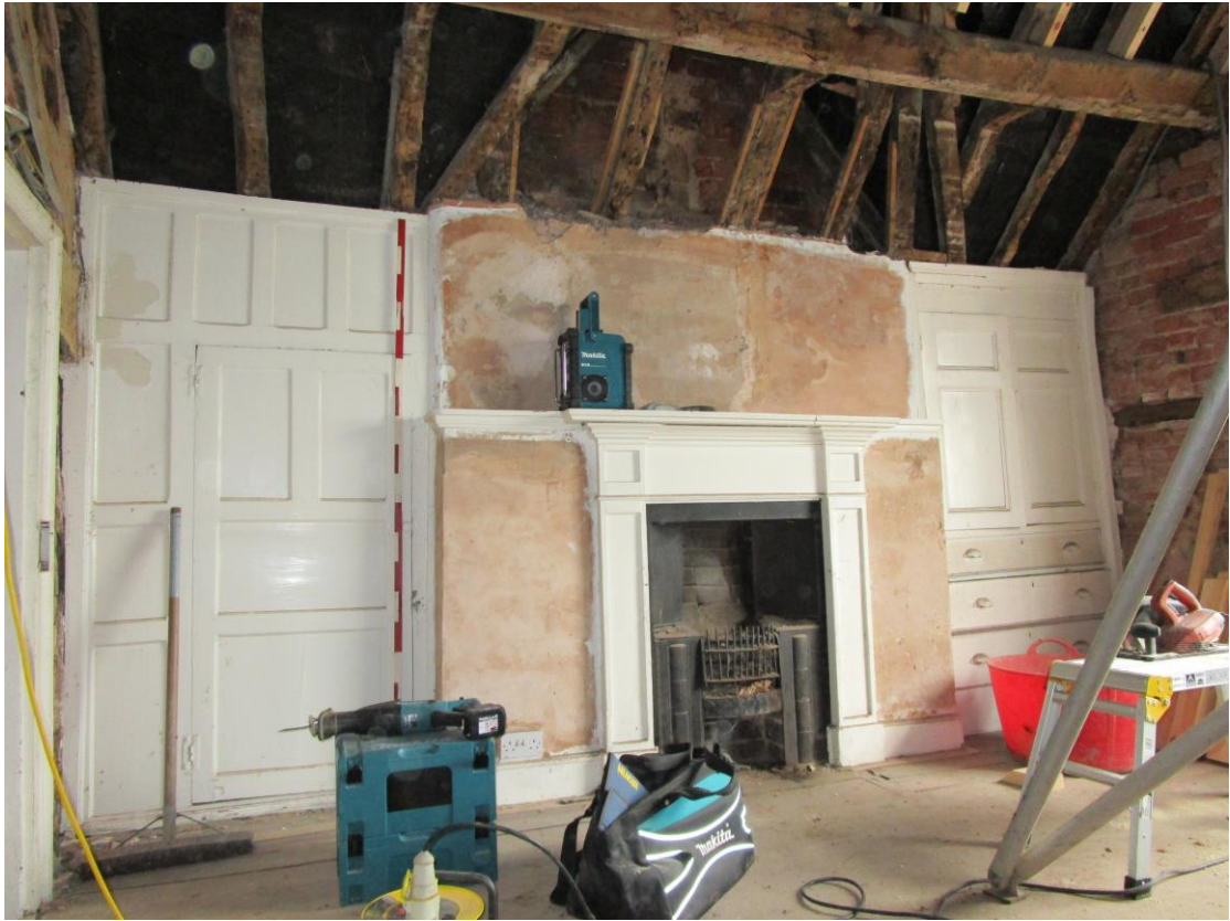
Plate 38; South-west wing; view of first floor interior from north-west
