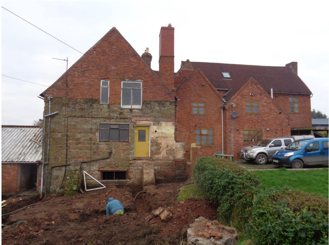
Plate 4; South elevation of farmhouse
