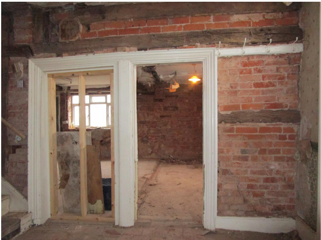
Plate16; South-west wing interior from the entrance hall
