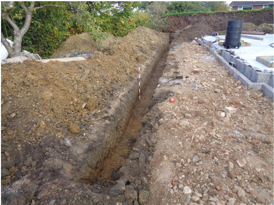
Plate 2; main sewer trench (section 1a), view east
