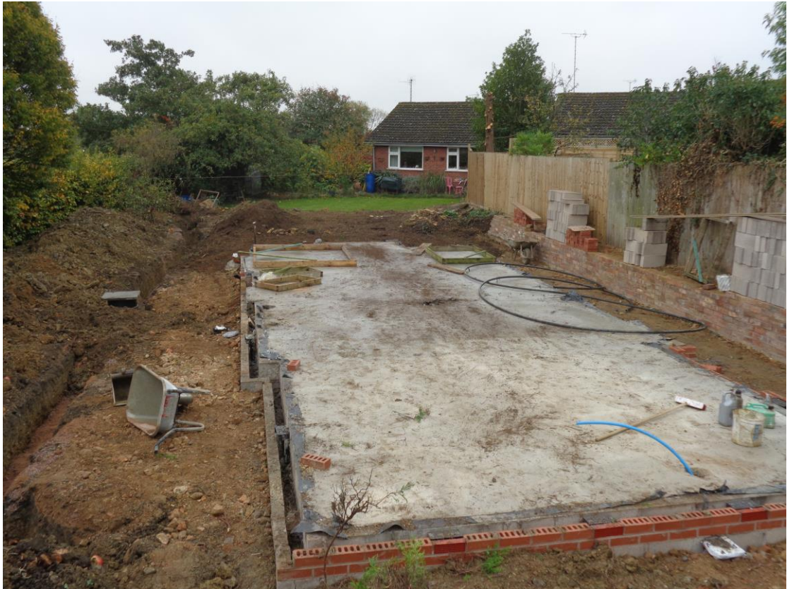
Plate 1; overall view to the east of the development site
