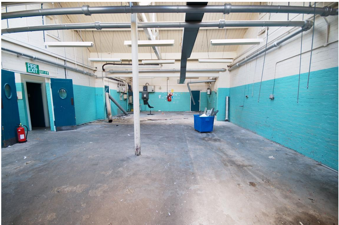
Plate 21; machine-shop 4 and beyond, to south
