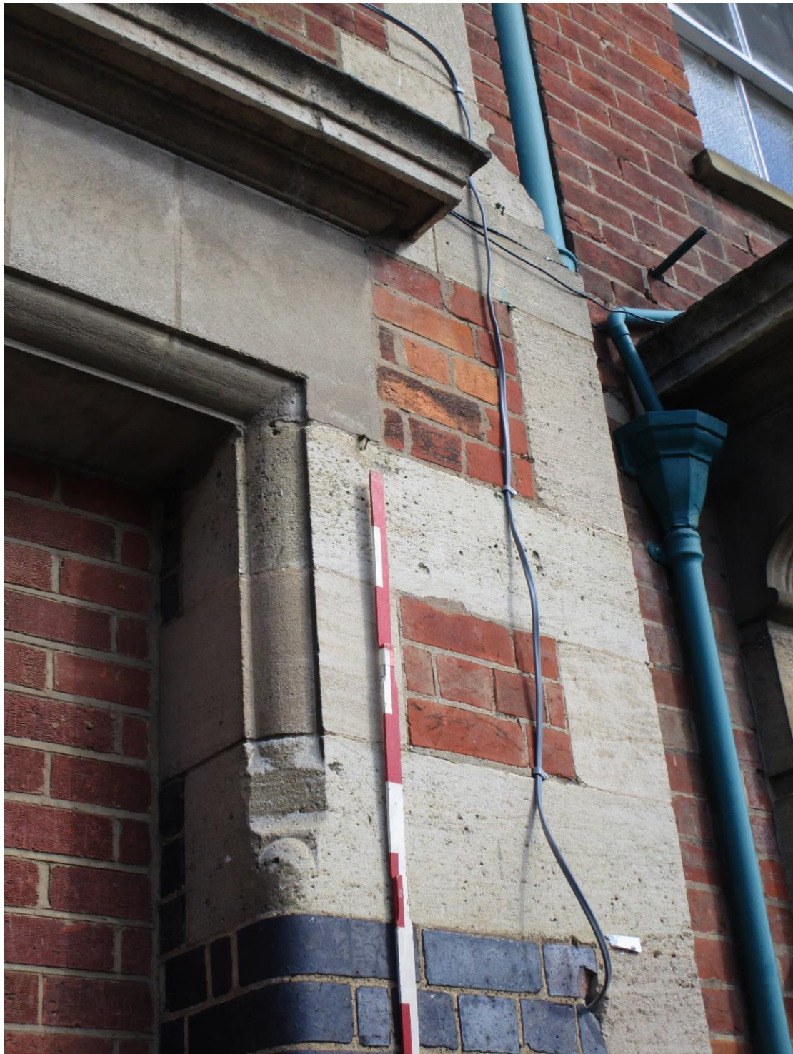
Plate 4; detail of blocked waggon-entry
