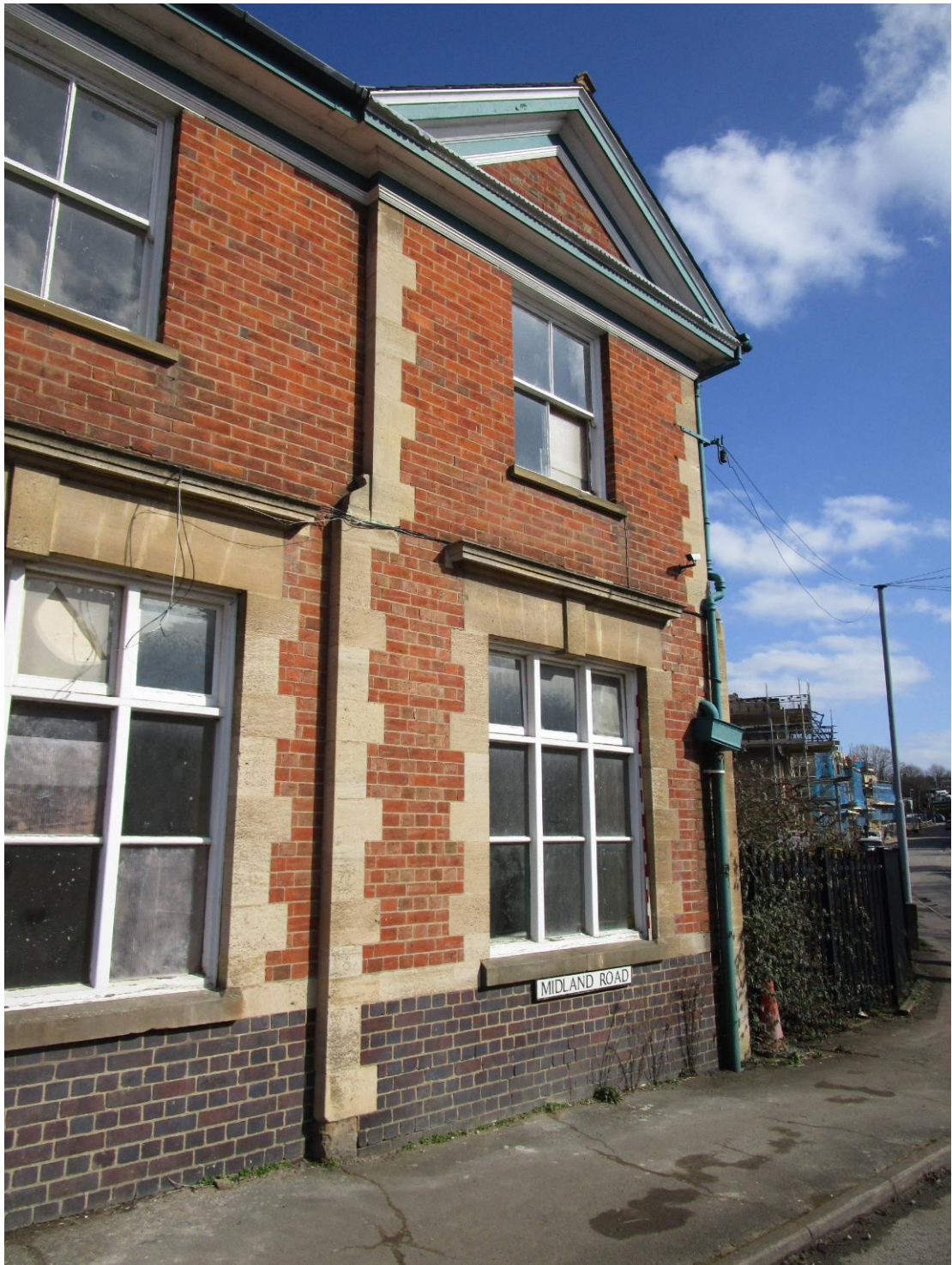
Plate 2; detail of east end of front
