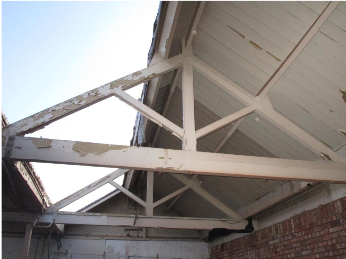
Plate 26; king-post frames over the original workshop
