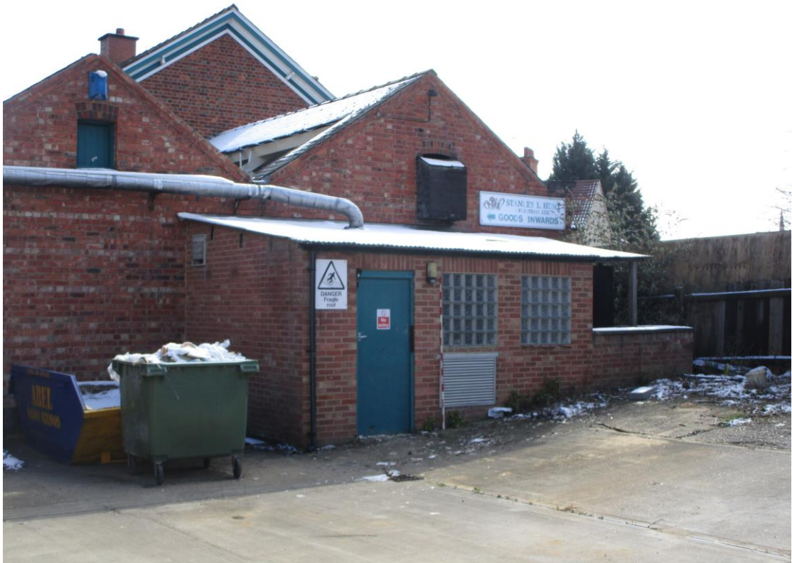
Plate 8; view from north-west of west end
