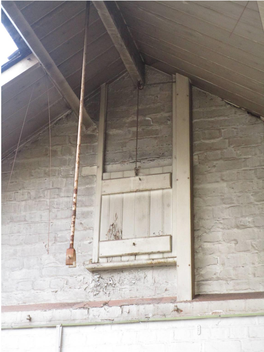
Plate 27; ventilation-hatch in gable
