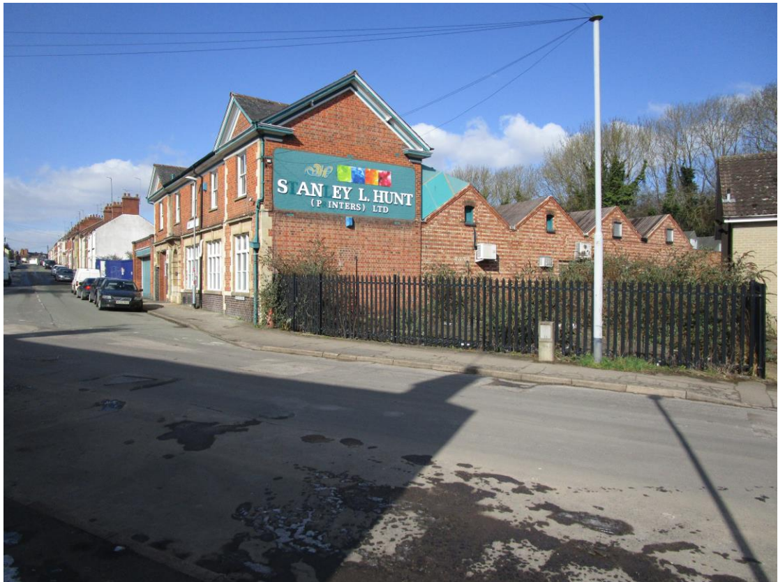
Plate 5; view from south-east showing roofing over rear workshop
