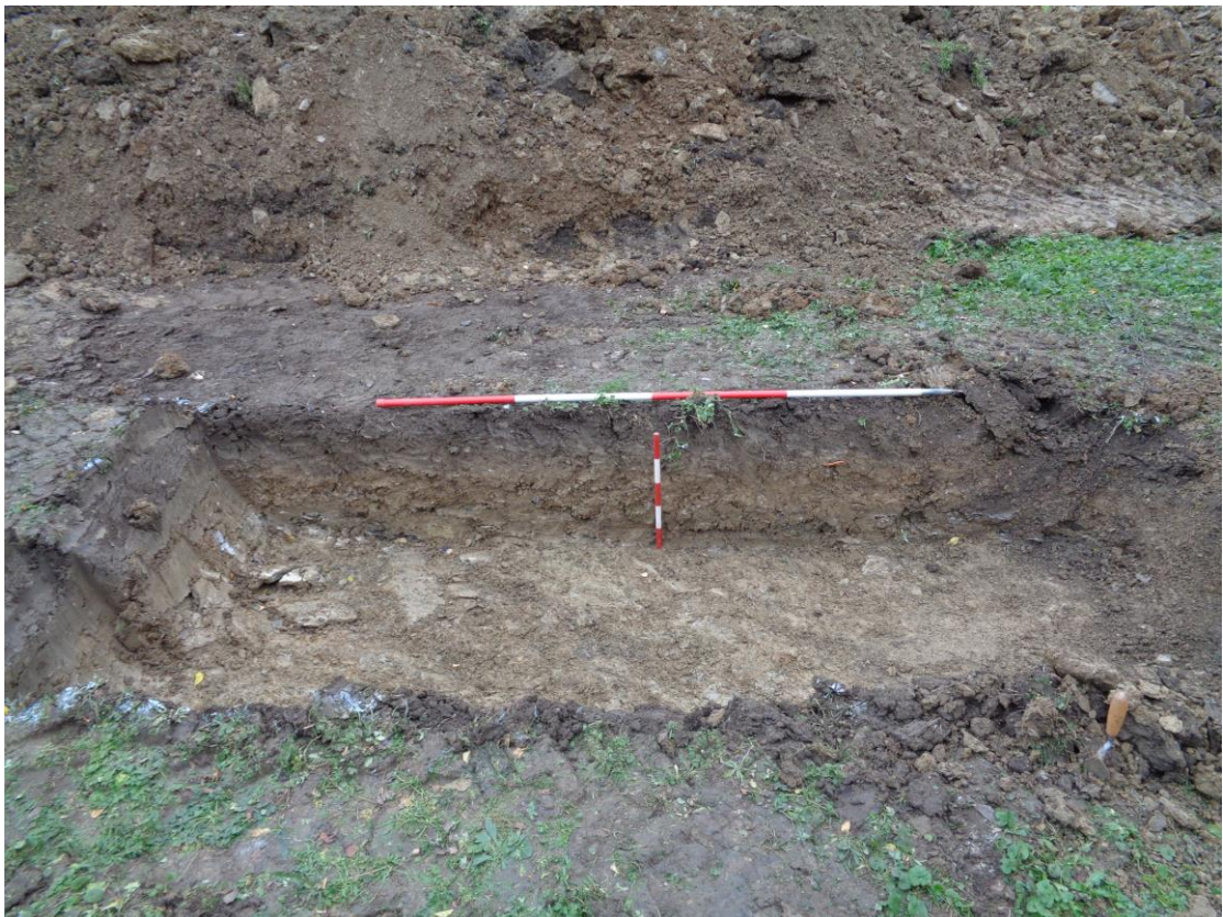
Plate 2; view north of the soak-away trench
