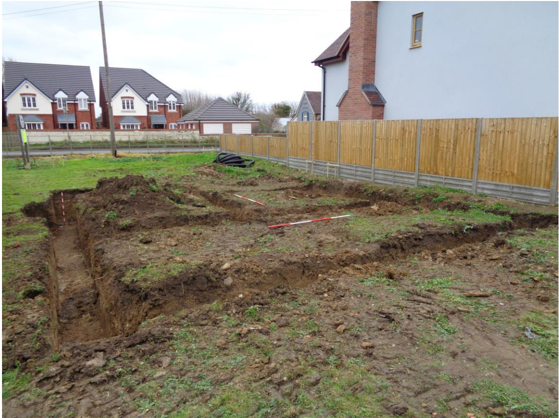
Plate 1; overall view to the east of the excavation
