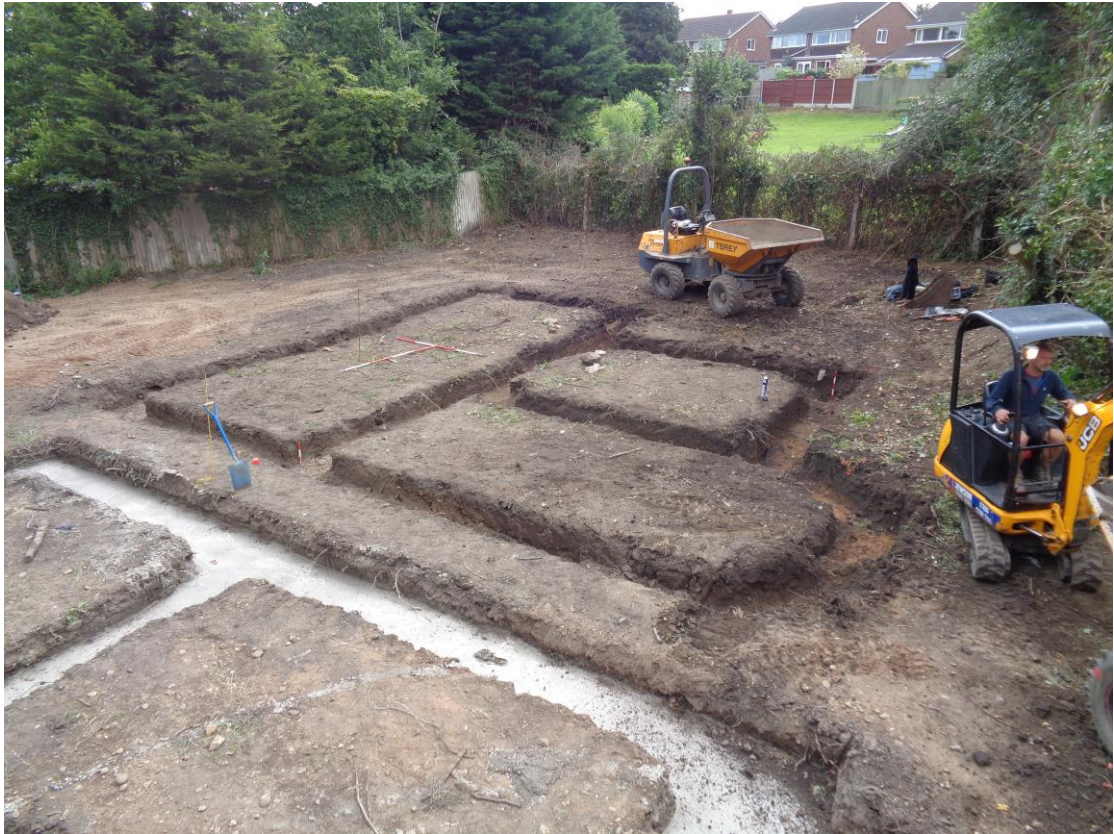
Plate 1; overall view to the south-east of trench 1 (plot four)
