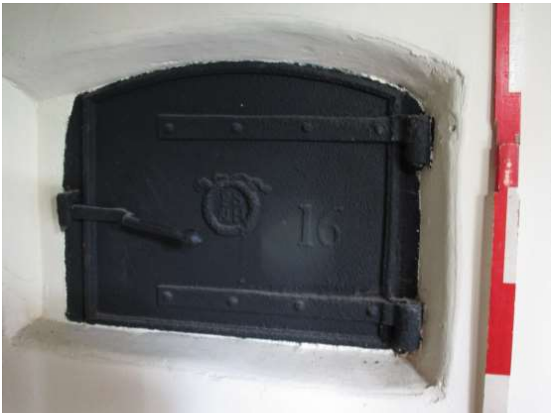
Plate 3; south chimney; oven door.
