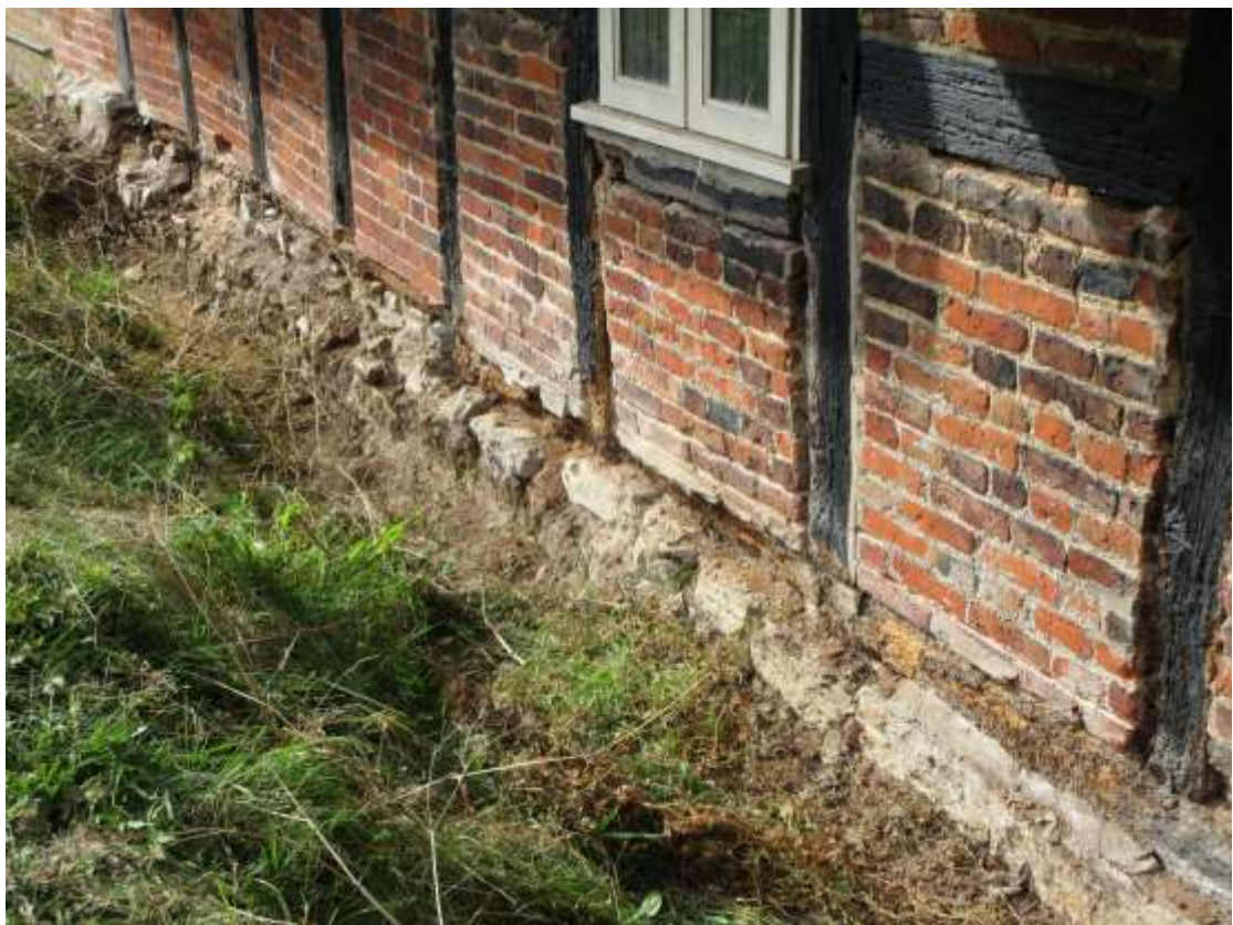
Plate 10; rubble dwarf-wall and cill-beam in southern part of east elevation.
