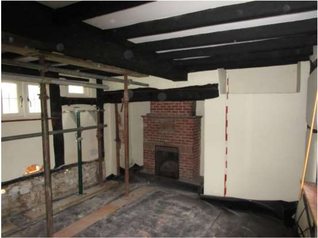
Plate 2; south chimney with inserted early C20 fireplace, note rubble dwarf-wall.
