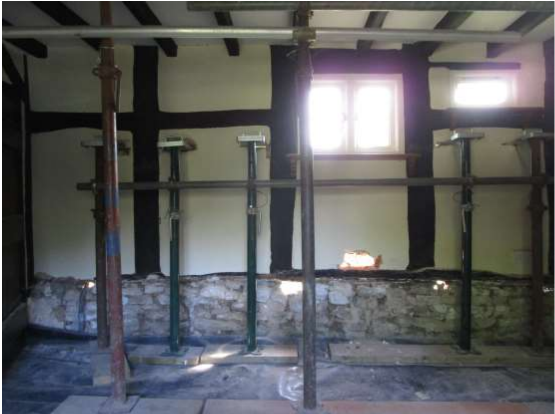
Plate 11; south room; showing rubble dwarf-wall.
