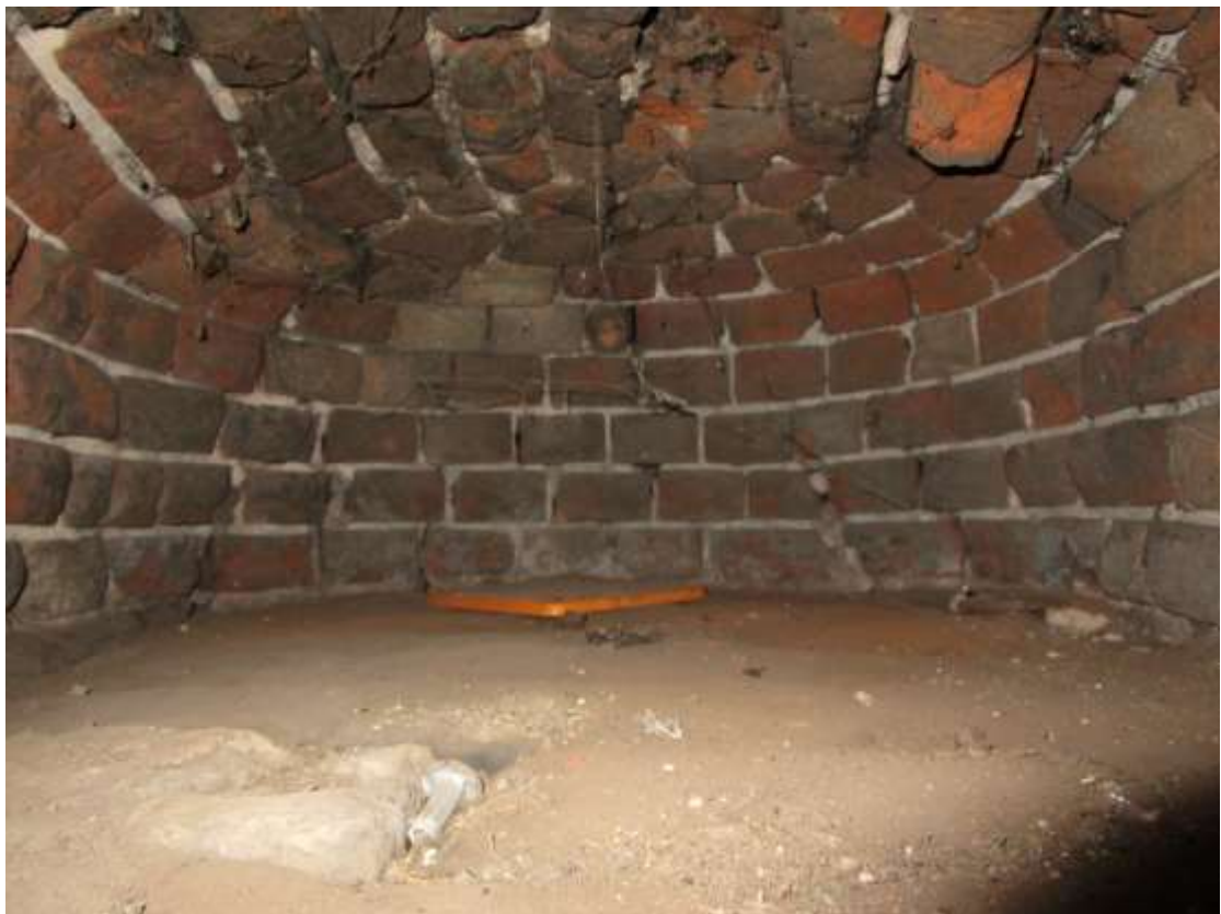
Plate 5; south chimney; oven interior.
