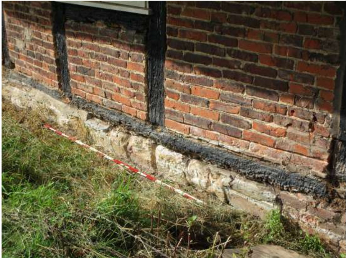
Plate 9; dwarf-wall at northern part of east elevation constructed of limestone blocks, possibly reused from demolished south chapel of All Saints' church.
