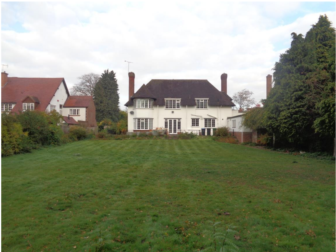
Plate 2; rear elevation of no.42 Tiddington Road, view to north-east
