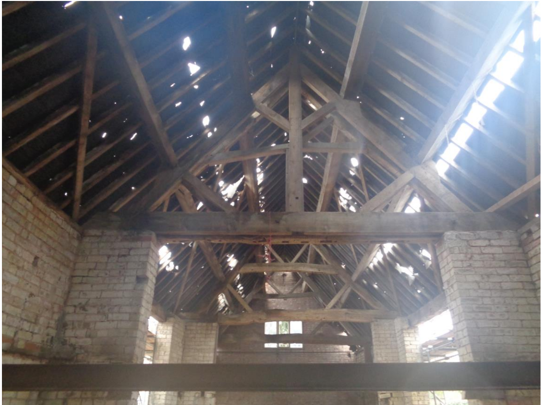
Plate 10; roof trusses in main barn, view to the west
