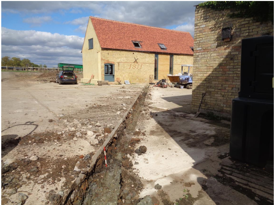
Plate 5; trench 11 across farmyard
