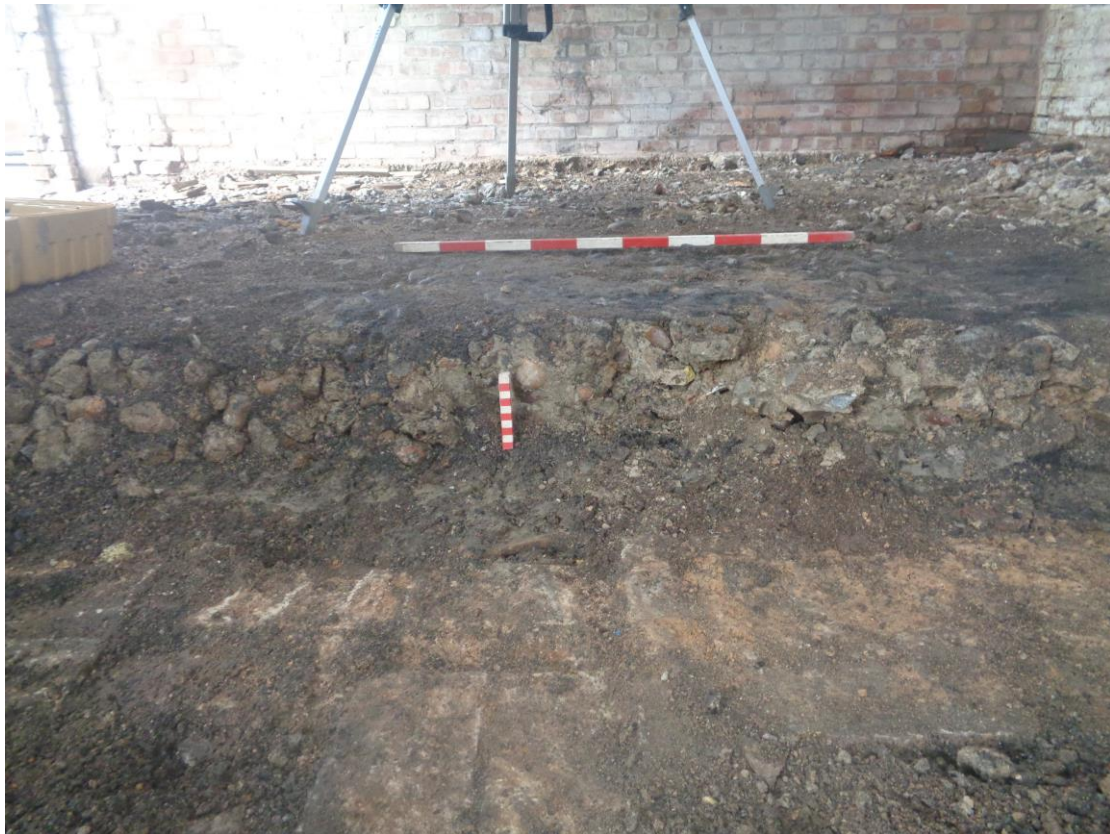
Plate 3; former internal floor surface (100) of the main threshing barn (east bay)
