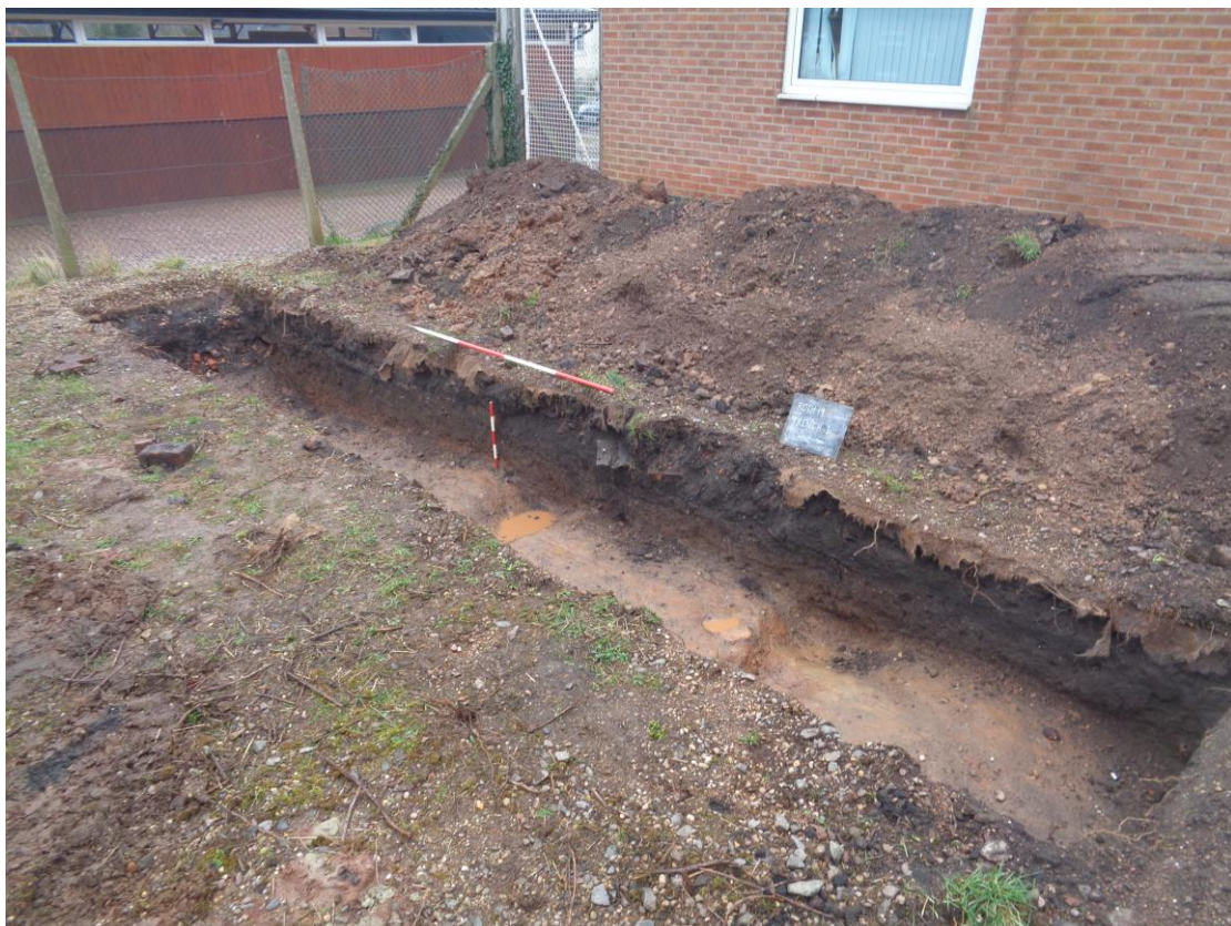
Plate 2; trench 1, view to the SW
