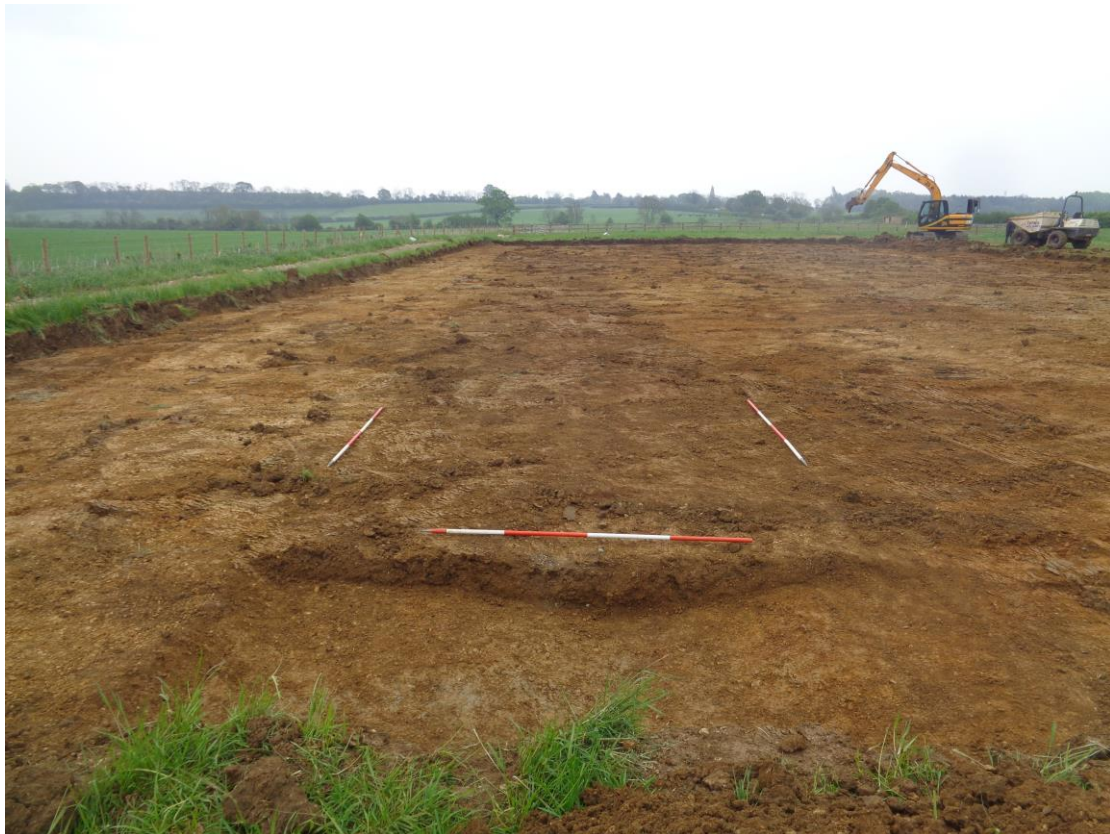
Plate 3; ditch feature 104, view to the north-east
