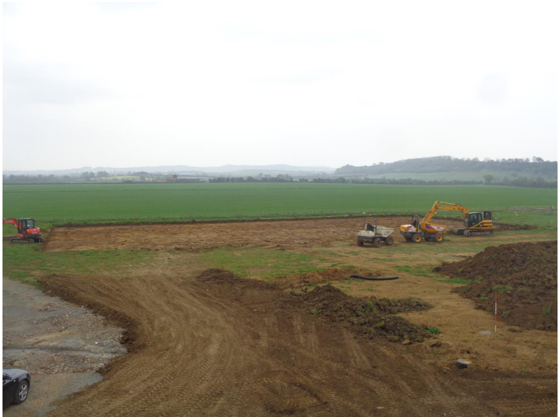
Plate 1; area of excavation, view to the north
