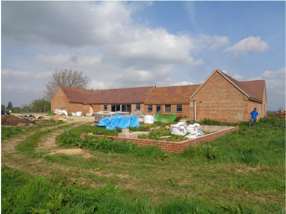
Plate 7; former C19 outfarm, front elevation, view to the north-west
