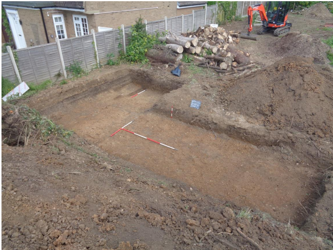
Plate 1; Trench 5, view from south-west.
