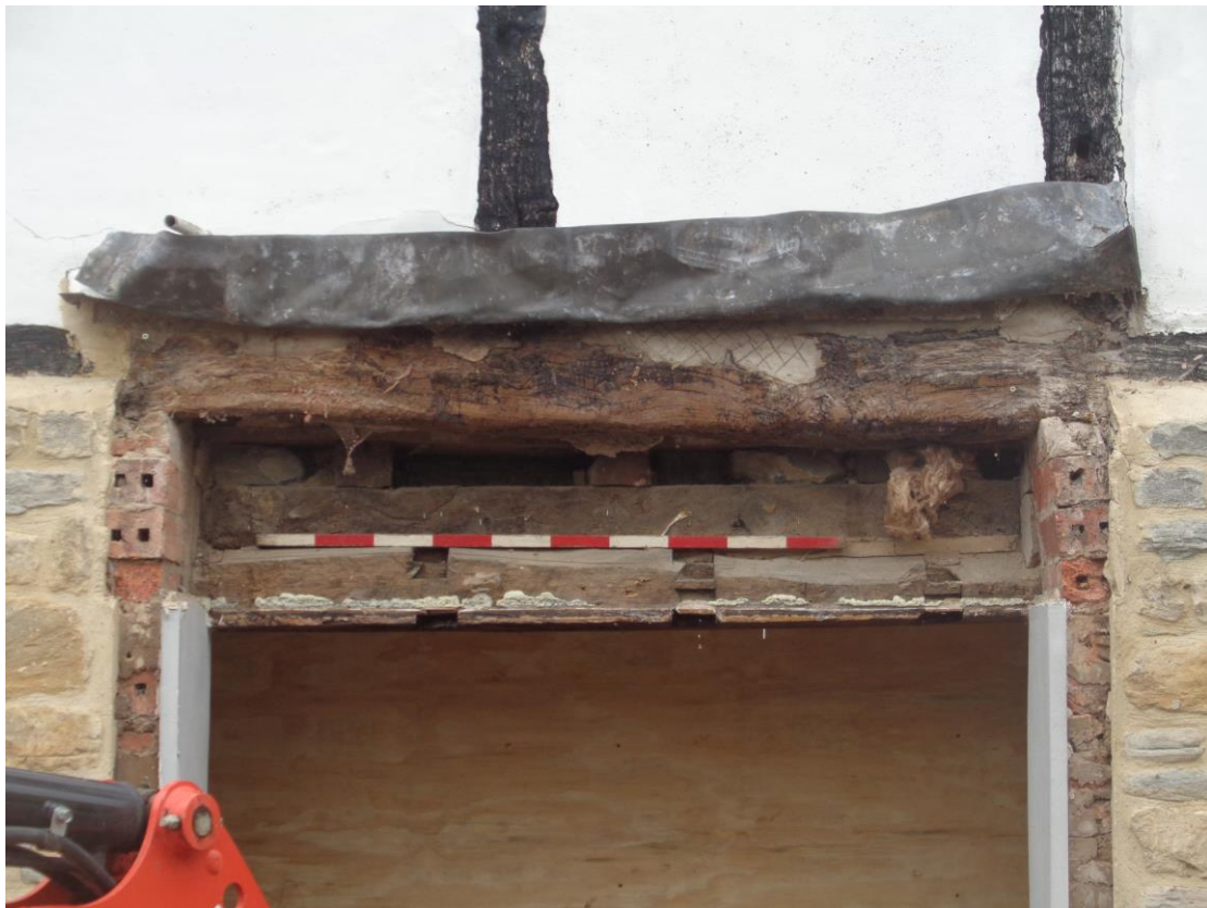
Fig 4; Rear elevation; detail of lintel, reused C18 principal-joist with notched-lap joints.
