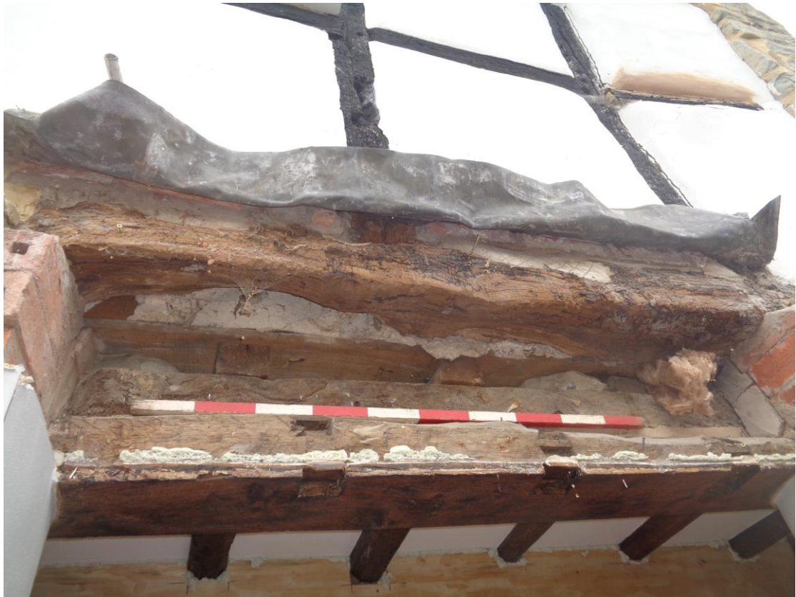
Fig 5; Rear elevation; view of lintel, reused C18 principal-joist with notched-lap joints.
