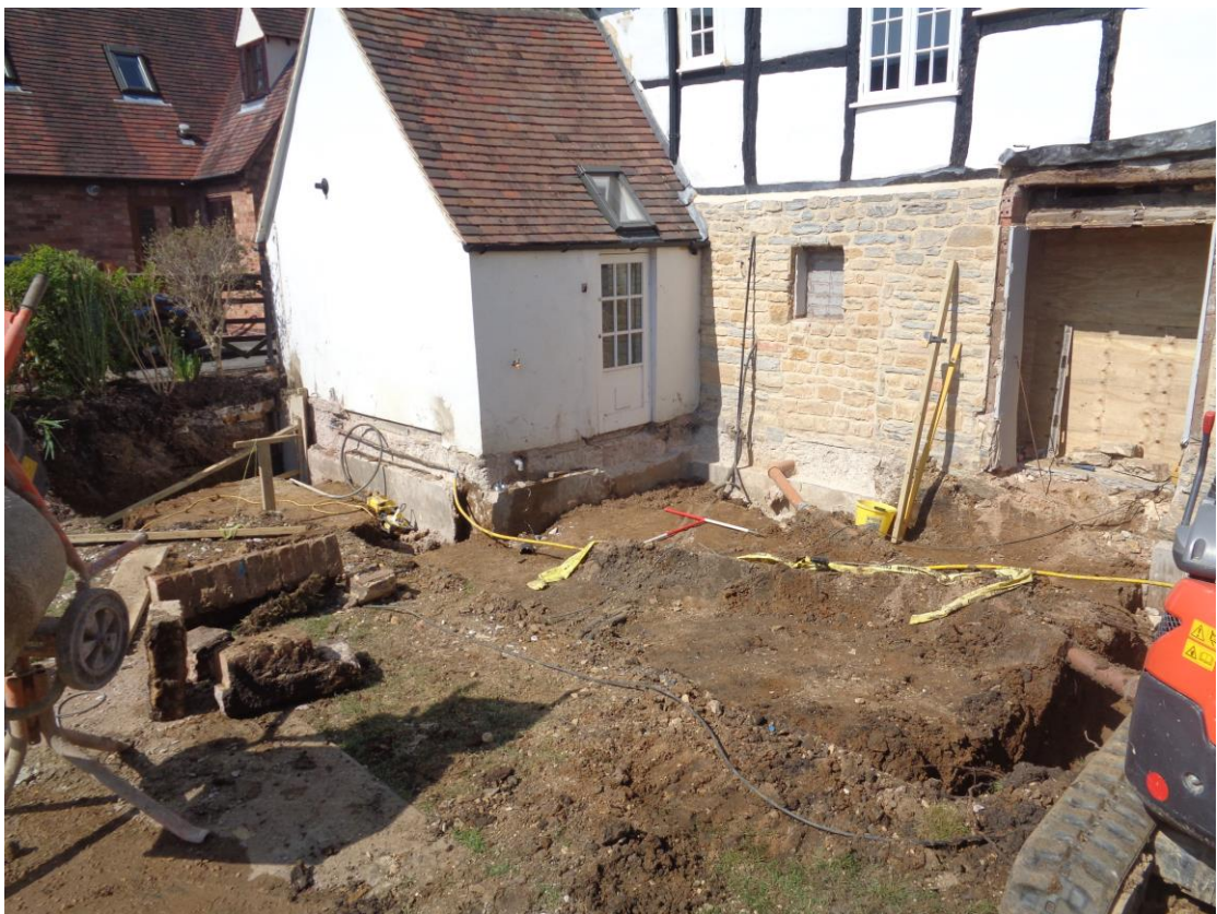
Plate 5; View of excavation from north-east.
