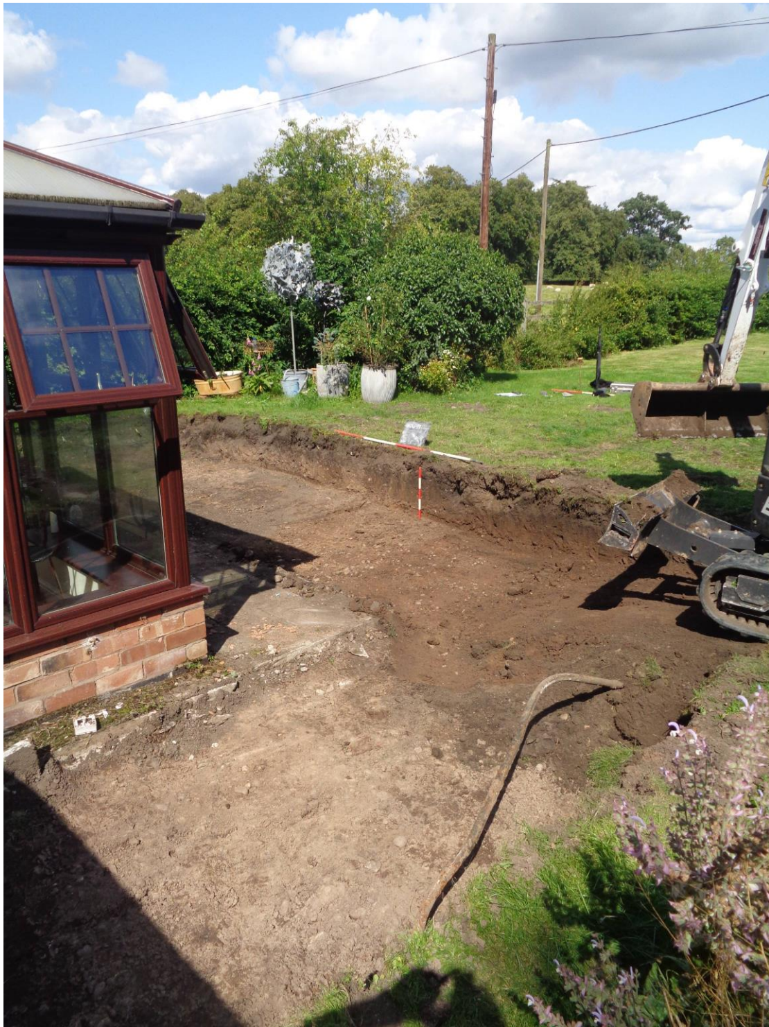
Plate 2; View of excavation from south-west.
