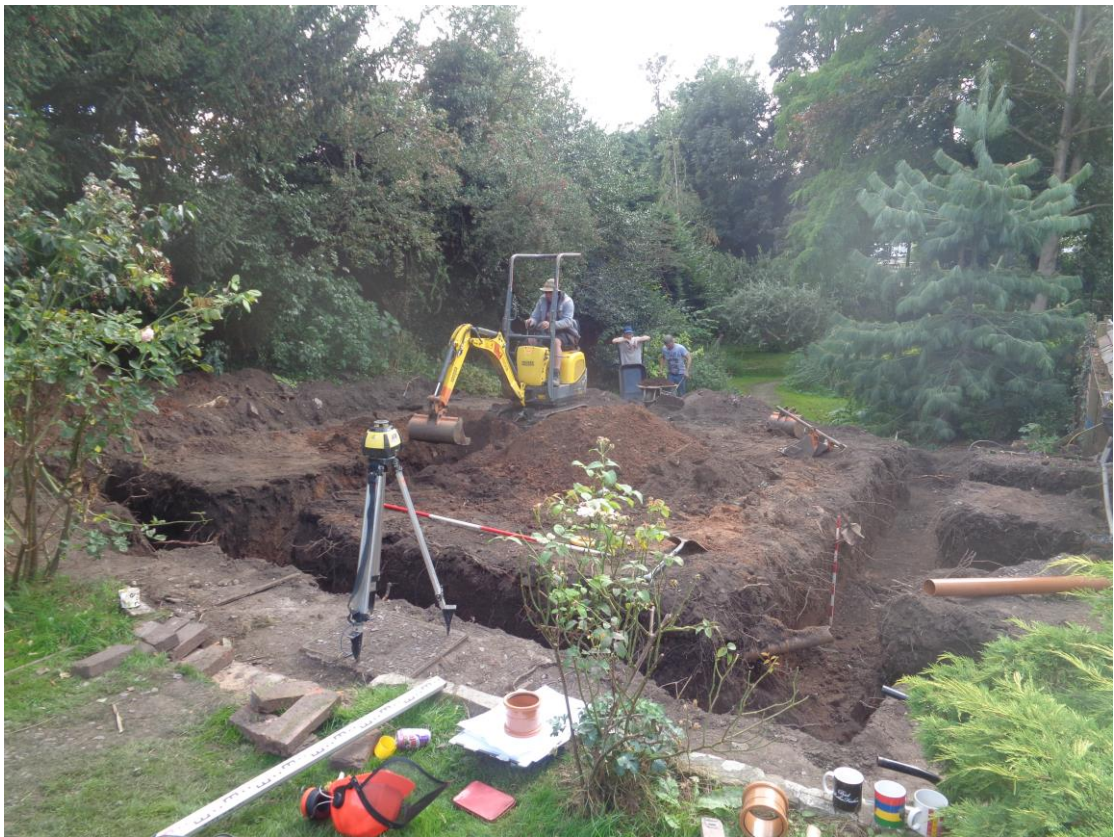
Plate 4; View of excavation from north-east.
