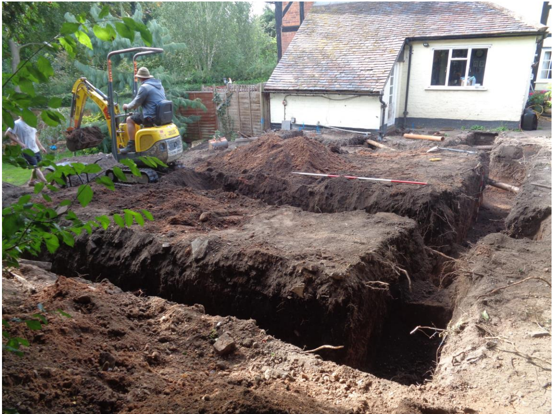
Plate 3; View of site from east during excavation.
