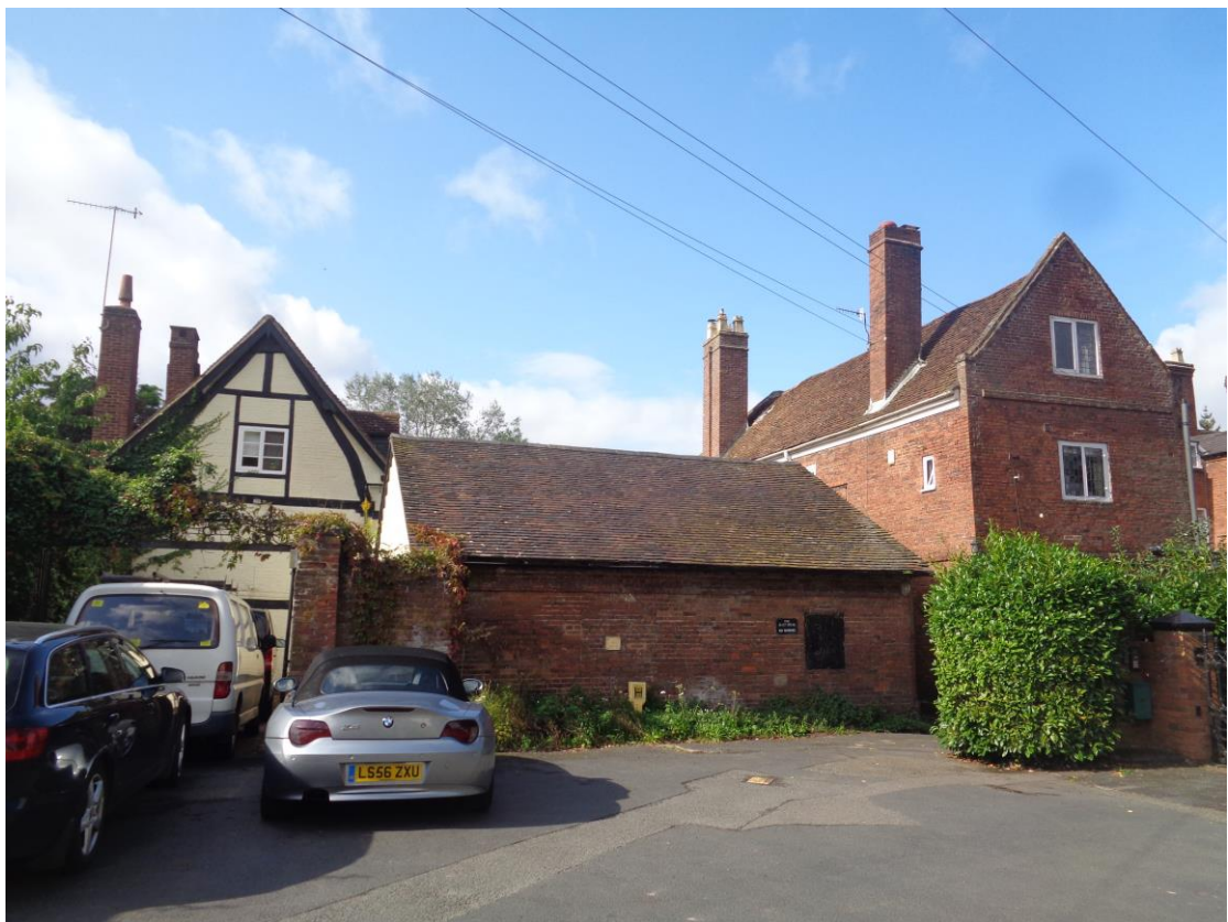
Plate 11; north side of Malthouse, view from the north
