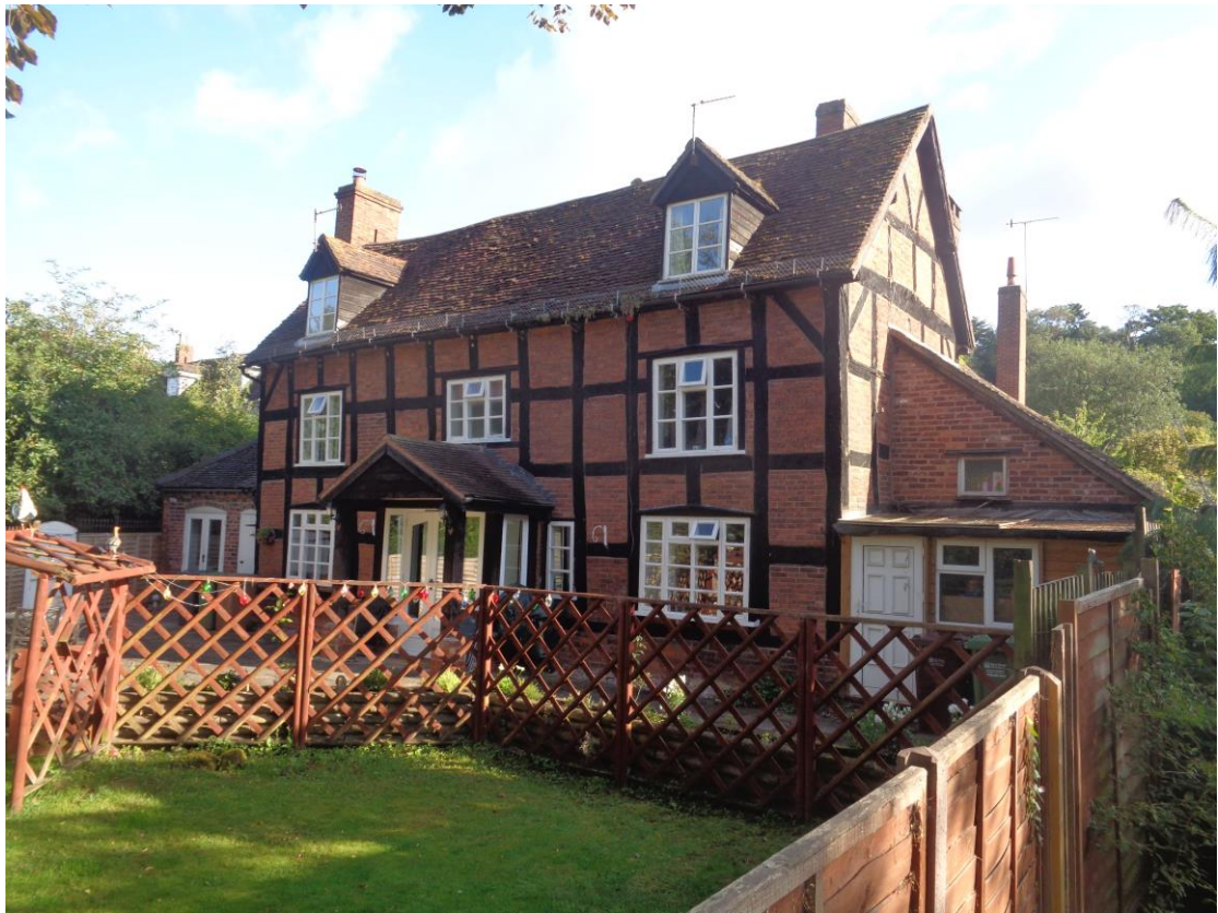
Plate 10; Bridgewater Cottage, view from the southeast
