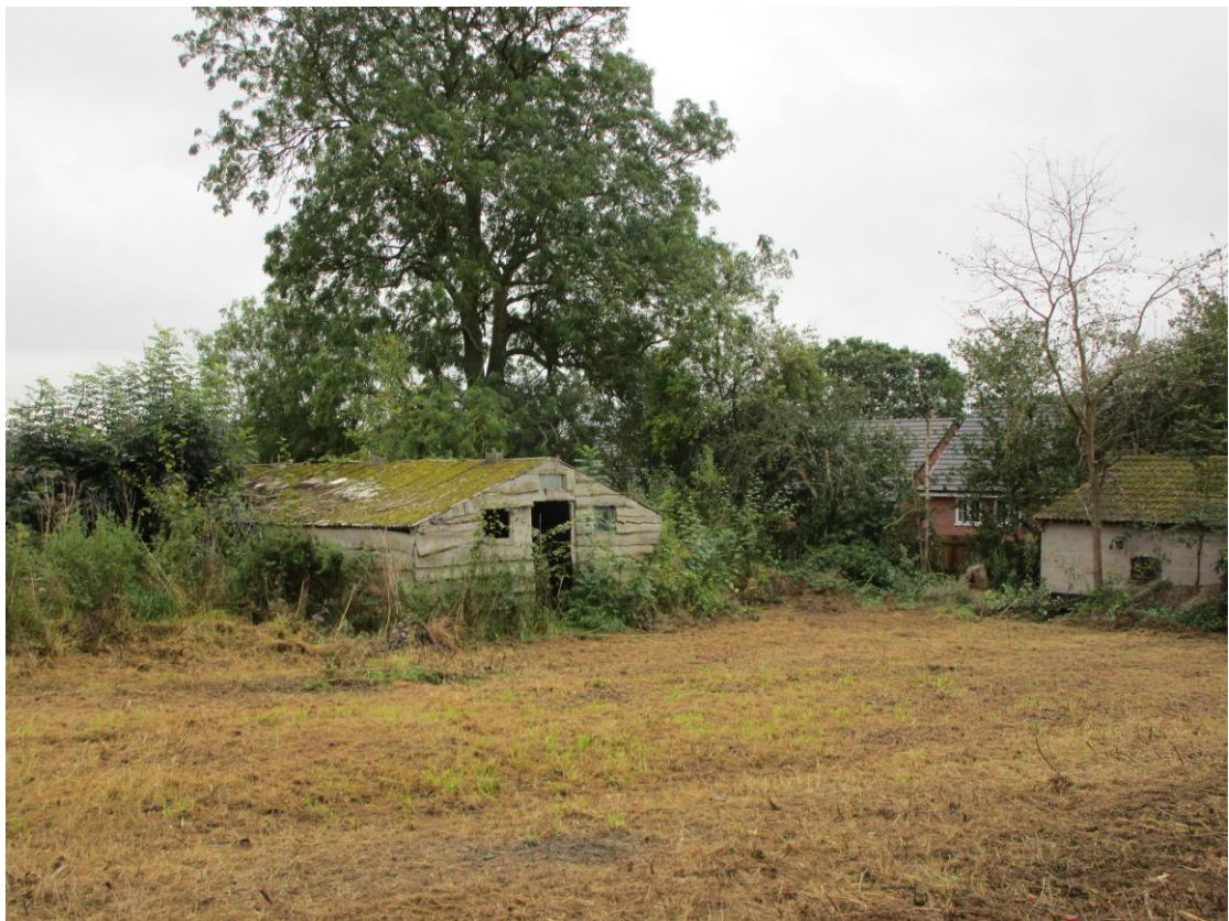
Plate 2; The ruinous shed from north.
