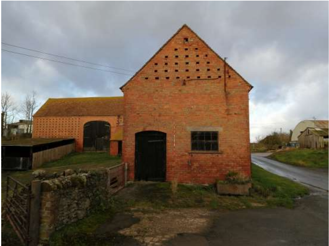
Plate 12; The gable end and remains of brick-dressed stone rubble foldyard walls.
