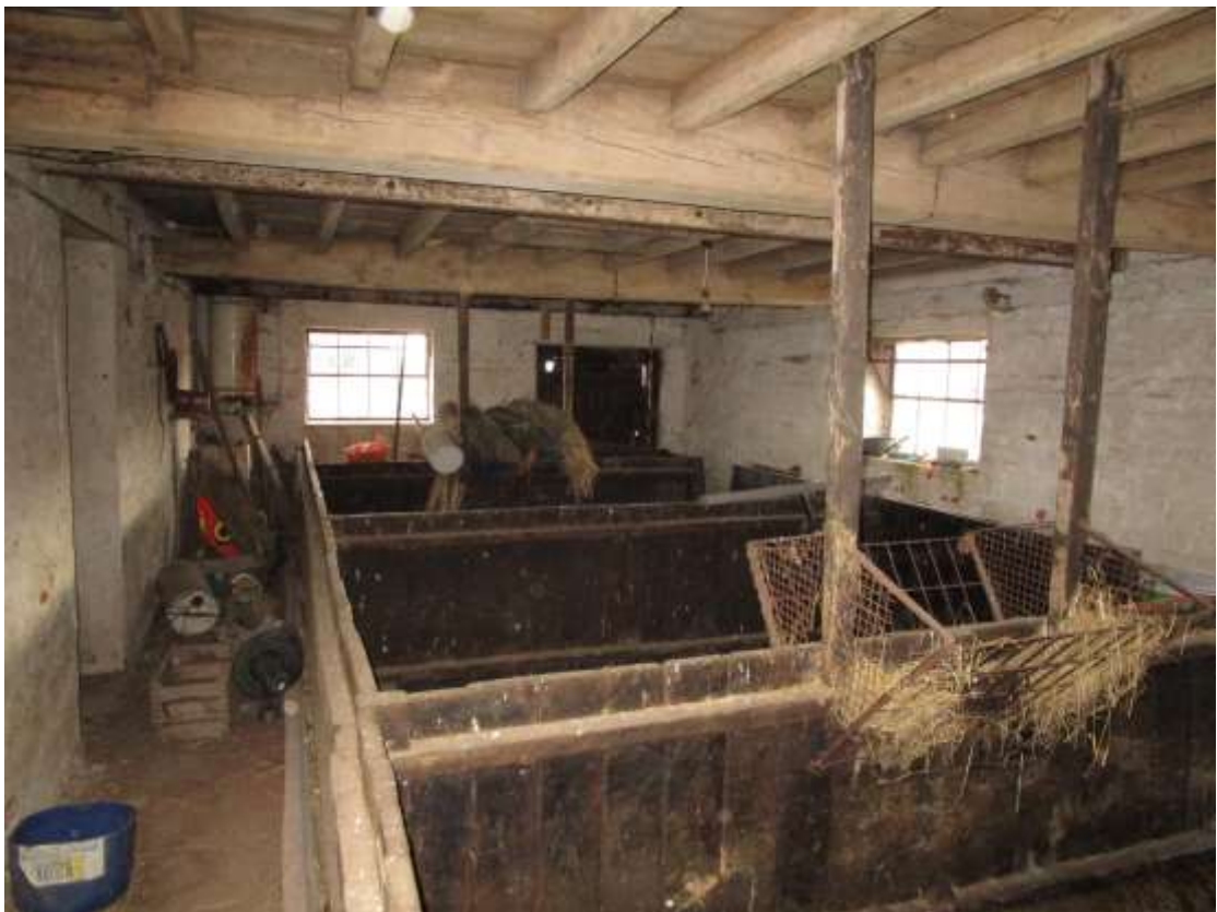
Plate 19; Former stables; with inserted cattle stalls and feeding-passage.
