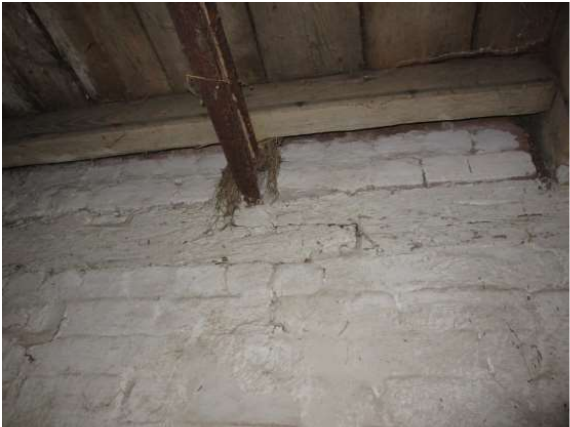
Plate 23; Former stables; Scarph in reused wall-plate, note birds' mouth to left.
