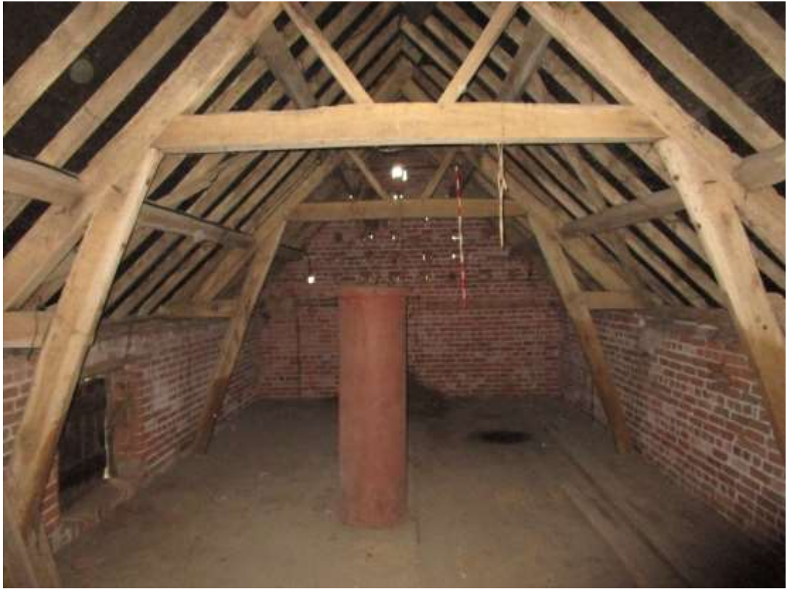
Plate 26; Former stables; Hayloft over
