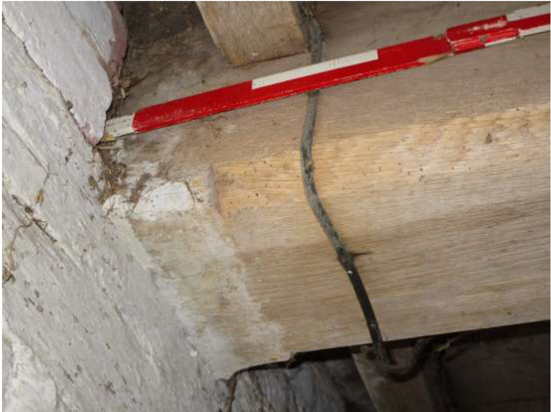
Plate 24; Former stables; neatly cut scroll-stops to chamfers on principal-joist.
