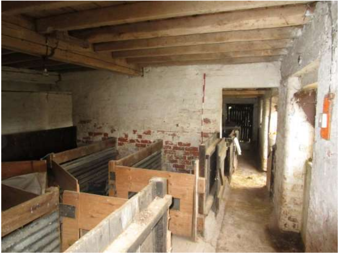
Plate 16; Former loosebox; inserted doorways, stalls and passages.
