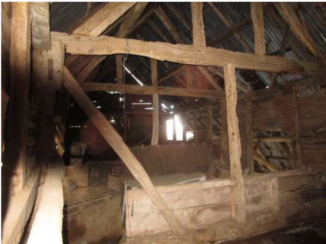
Fig 2; The barn interior showing the outshot beyond, late C17/early C18.
