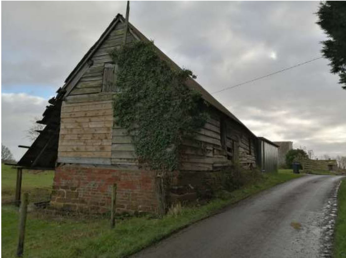
Fig 1; The timber-framed barn, late C17, north-west of the cart-shed.
