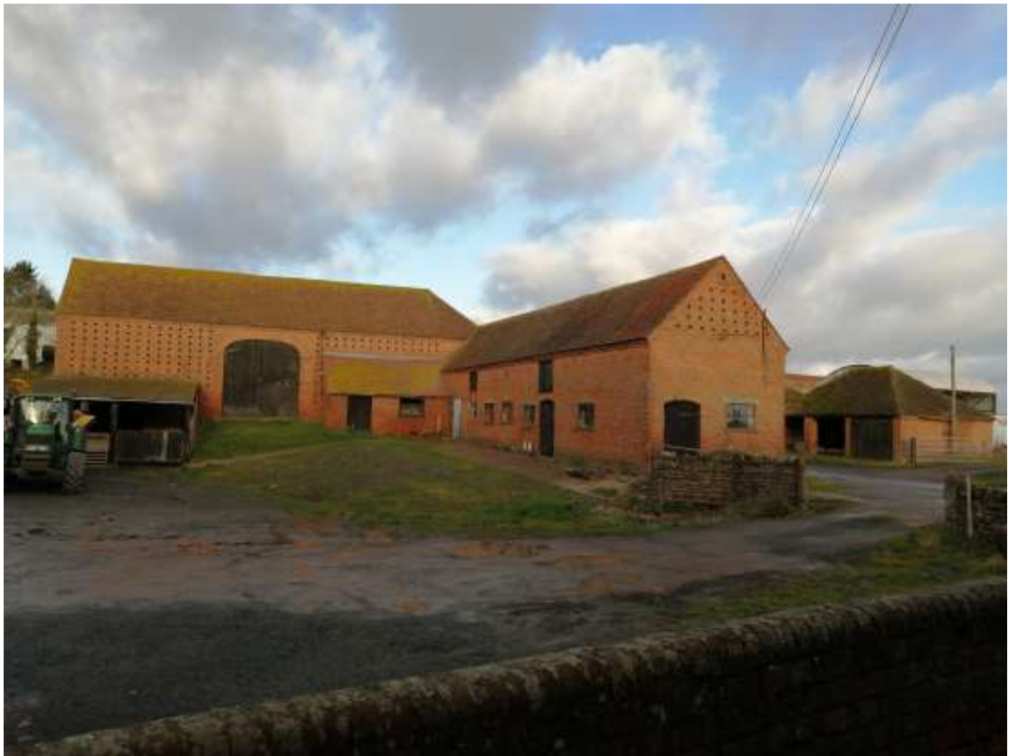
Plate 6; The south prospect of the barn and north-east range.
