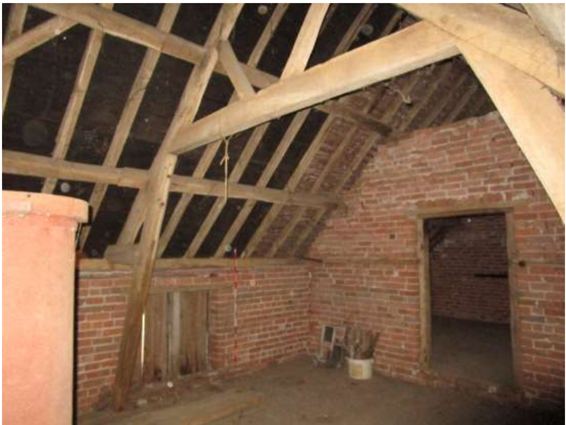
Plate 27; Former stables; Hayloft over
