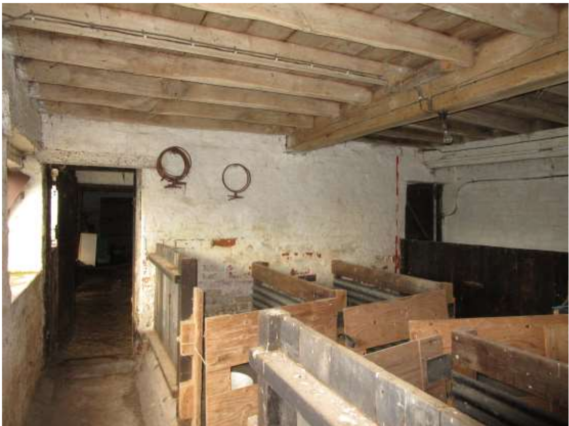
Plate 15; Former loosebox; inserted doorways, stalls and passages.
