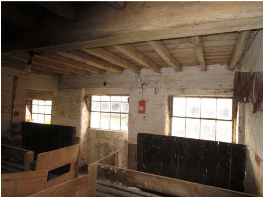
Plate 17; Former loosebox; inserted stalls, passages and blocked door.
