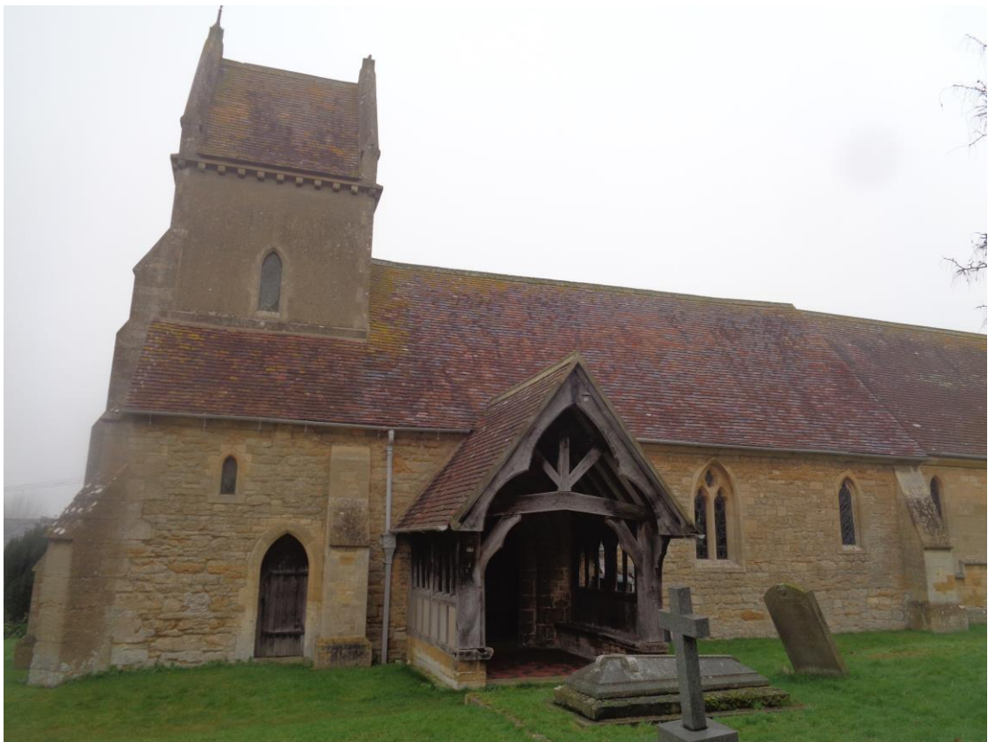
Plate 2; The south wall of the nave showing later insertions and additions.
