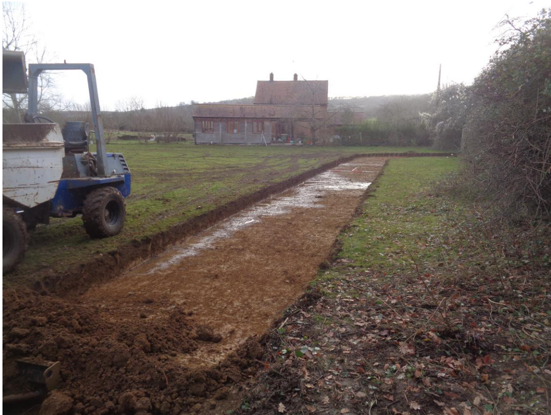
Plate 1; View of the excavation southward, toward Bredon Hill in the distance.
